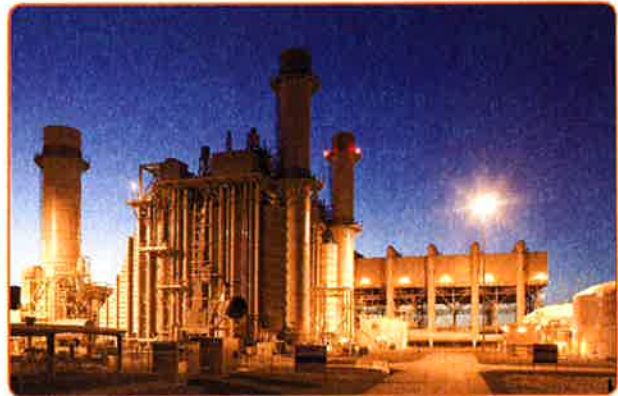
Currant Creek Power Plant, Mona, Utah
