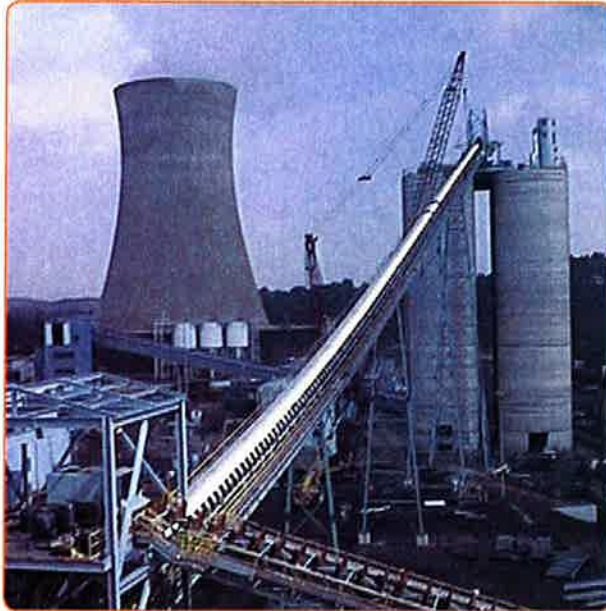
Miller Steam Plant, Alabama
