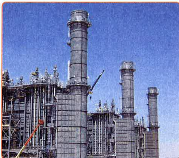
Harquahala Power Plant, Tonopah, Arizona
