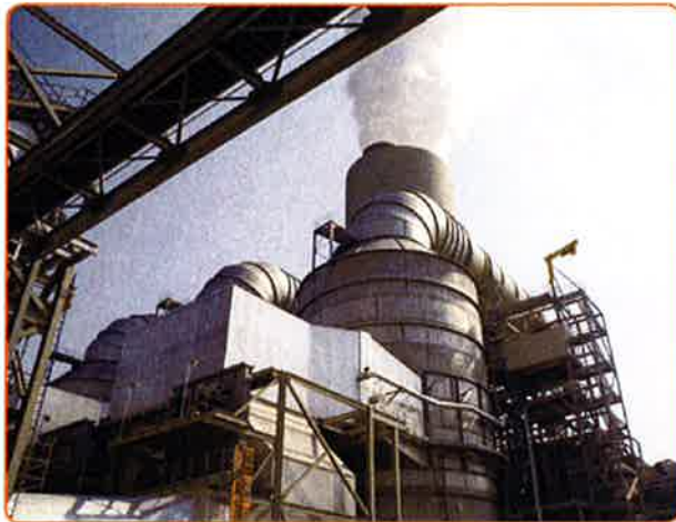
FGD Retrofit at Coal-Fired Unit
