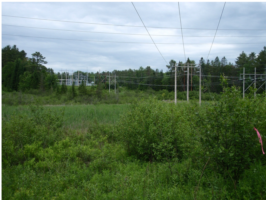
Photo 4: View southwest towards Littleton Substation from Interstate 93.
