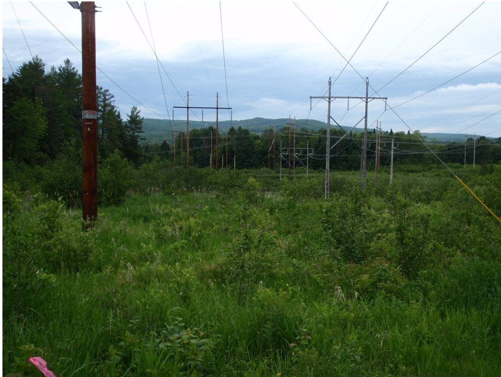
Photo 1: View of the project Site facing north taken from Littleton Substation.
