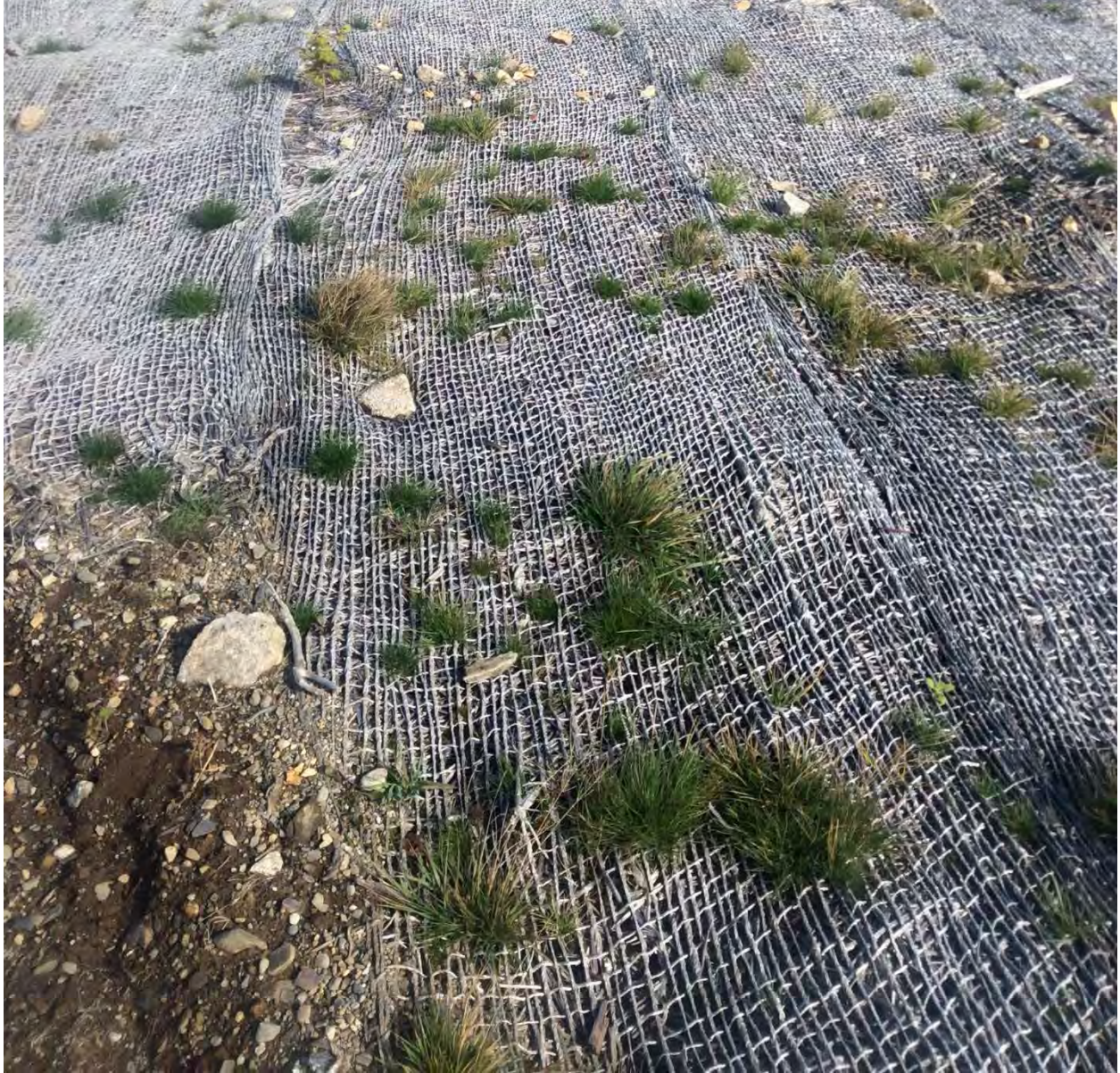
Figure 20: Jute Erosion mesh. After one growing season grass is already establishing itself
