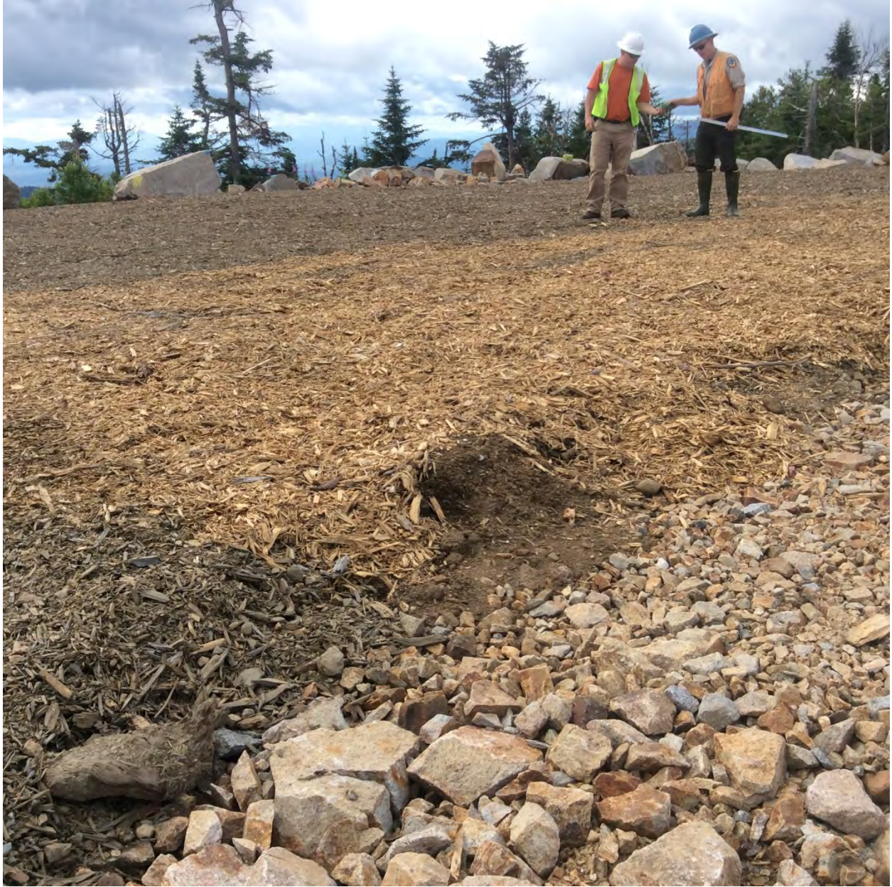
Figure 5: Pad area ready for planting, with correct soil depth and woodchips
