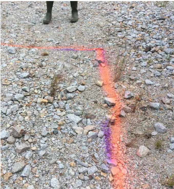
Figure 4: Layout of soil placement on Pads
