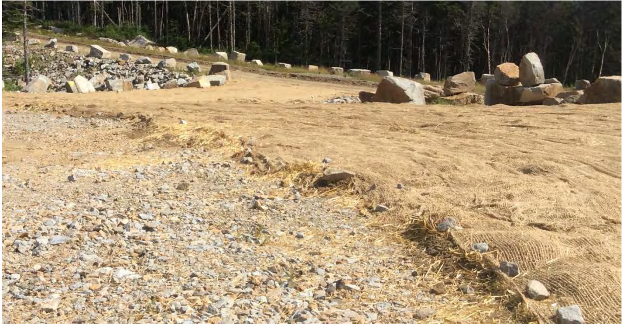
Figure 6: Pad 13- Ready for planting with 4 inches of soil, straw and Jute erosion cloth
