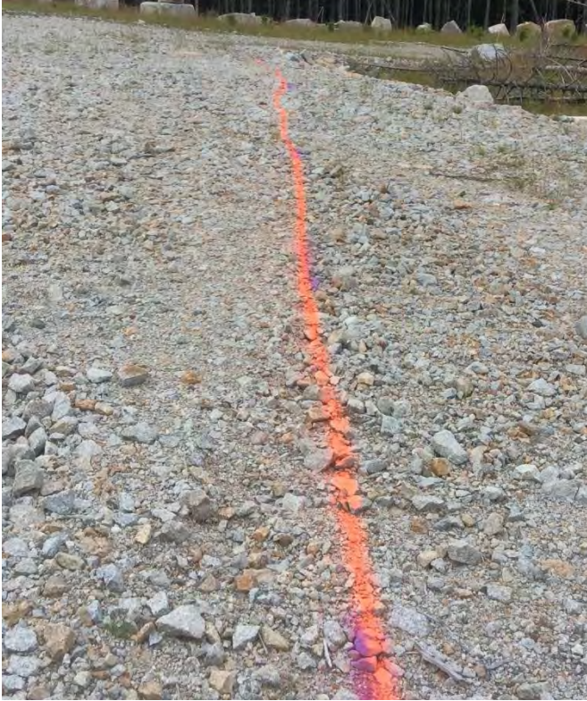
Figure 3: Layout of soil placement on Pads
