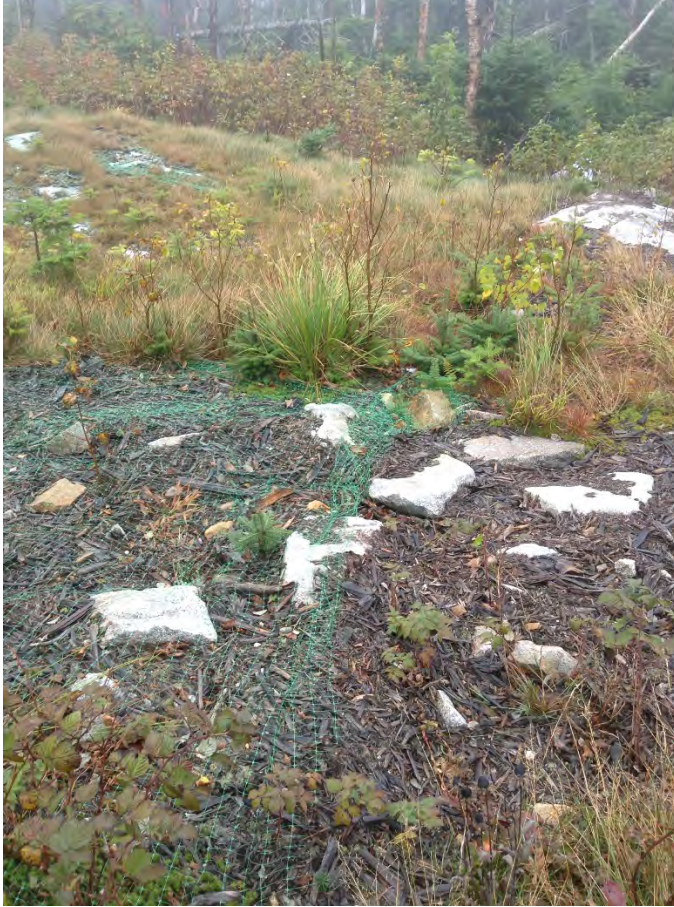
Figure 18: Green mesh: Continues to be present on the landscape. This shows the importance of using something like Jutte which is flexible and breaks down over time
