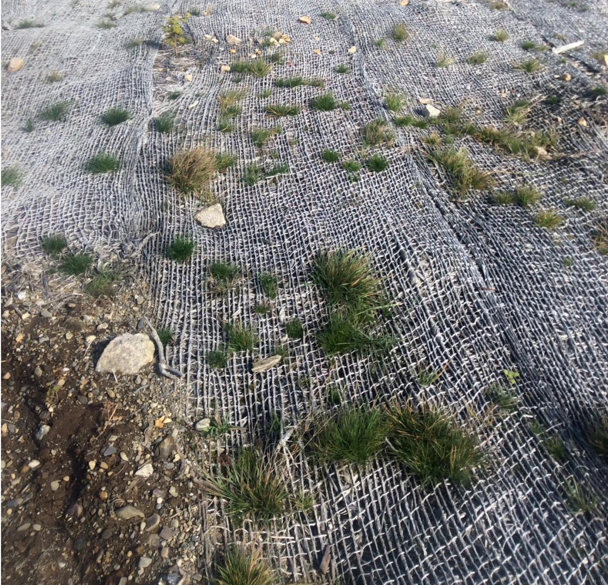
Figure 14: Jute Erosion mesh. After one growing season grass is already establishing itself
