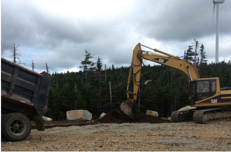
Figure 1: Pad 10: soil spread with excavator (to decrease soil compaction), Dump truck placing soil on pad area delineated with paint. Excavator operator is spreading to specified soil depth for specific pad depths. Machine was then used to tread site once for soil stabilization.
