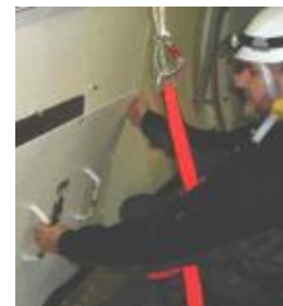
Remove evacuation hatch
