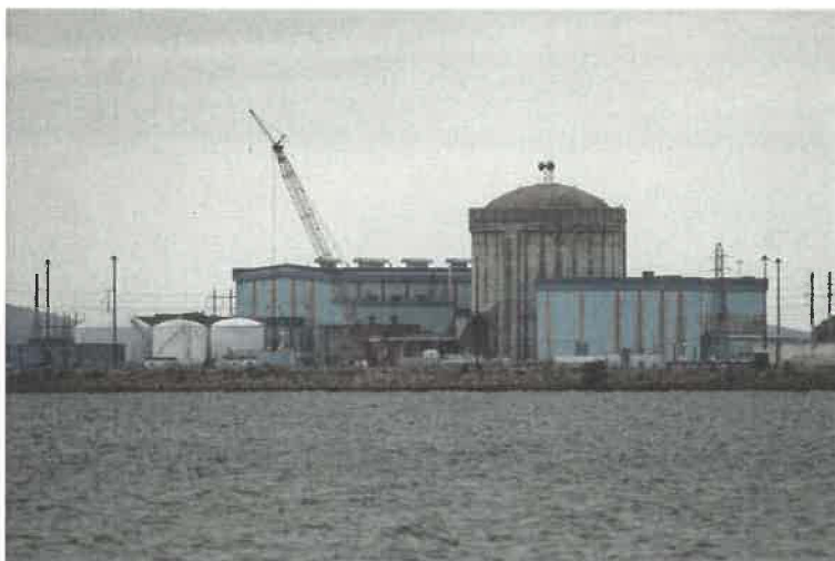
Unit one of the V.C. Summer Nuclear Stations near Jenkinsville, South Carolina, in 2106. Chuck Burton / AP
