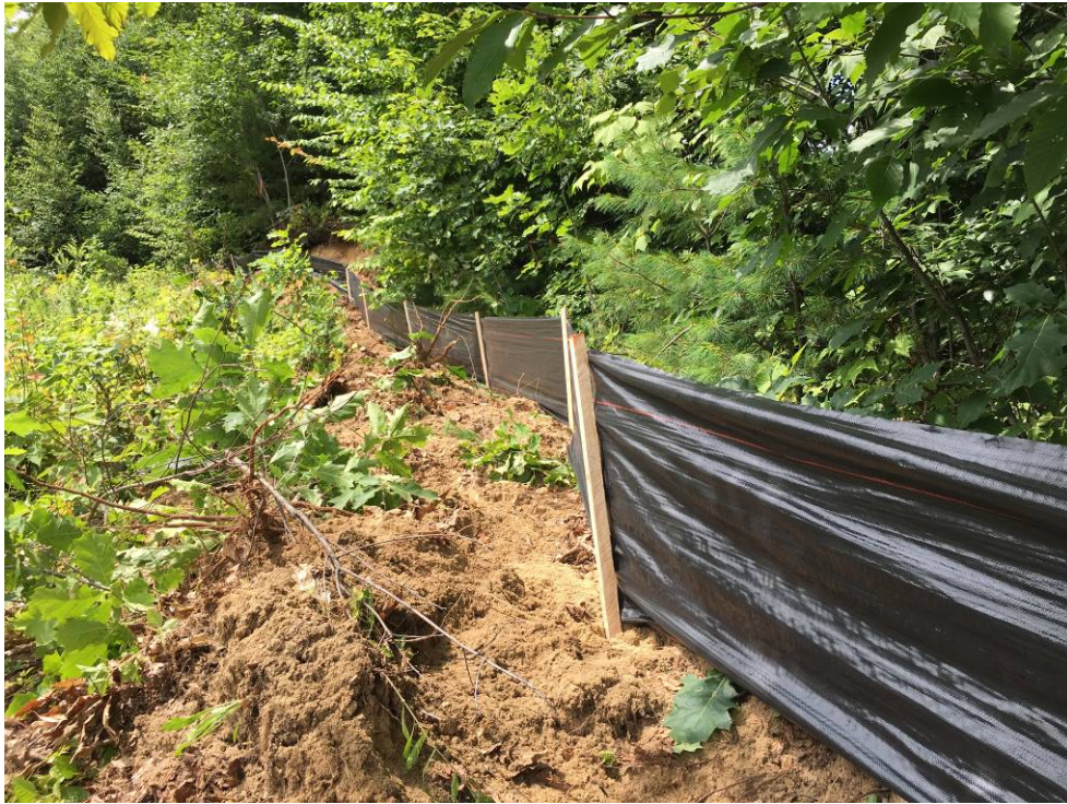
Outer silt fence installed.
