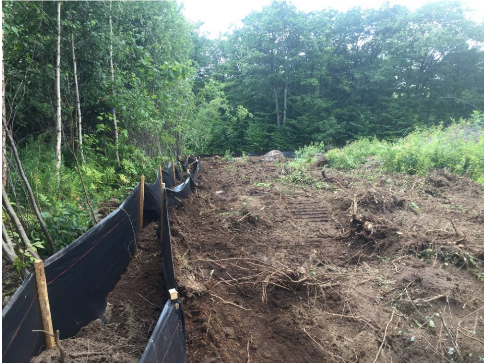
Double silt fence installed.
