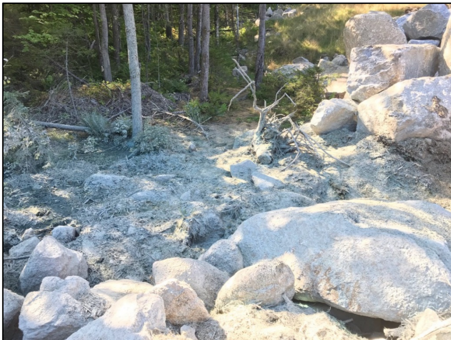
Photo 2: Image taken on 8/28/2019. Image showing the base of the rock slope adjacent to wetland AN-41 was hydroseeded prior to the inspection on 8/28/2019.
