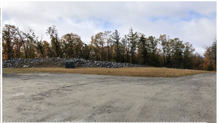
View of Turbine Pad 5 and vegetated area adjacent to Turbine Pad 5 at STA 95+00.
