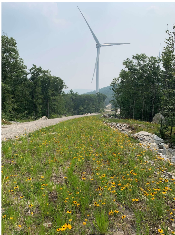
Photo 1. Typical revegetating access road corridor north of turbine T6. July 26, 2021, Stantec.
