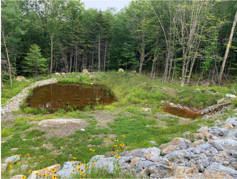
Photo 3. Typical stormwater retention basin north of turbine T1. July 26, 2021, Stantec.
