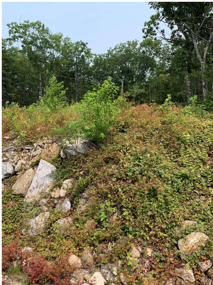
Photo 2. Stabilized and revegetated bank at turbine T8. July 26, 2021, Stantec.
