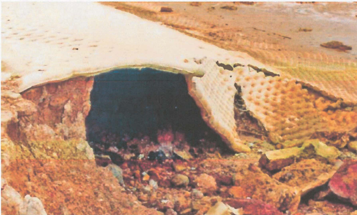
Example of failed concrete mattress
