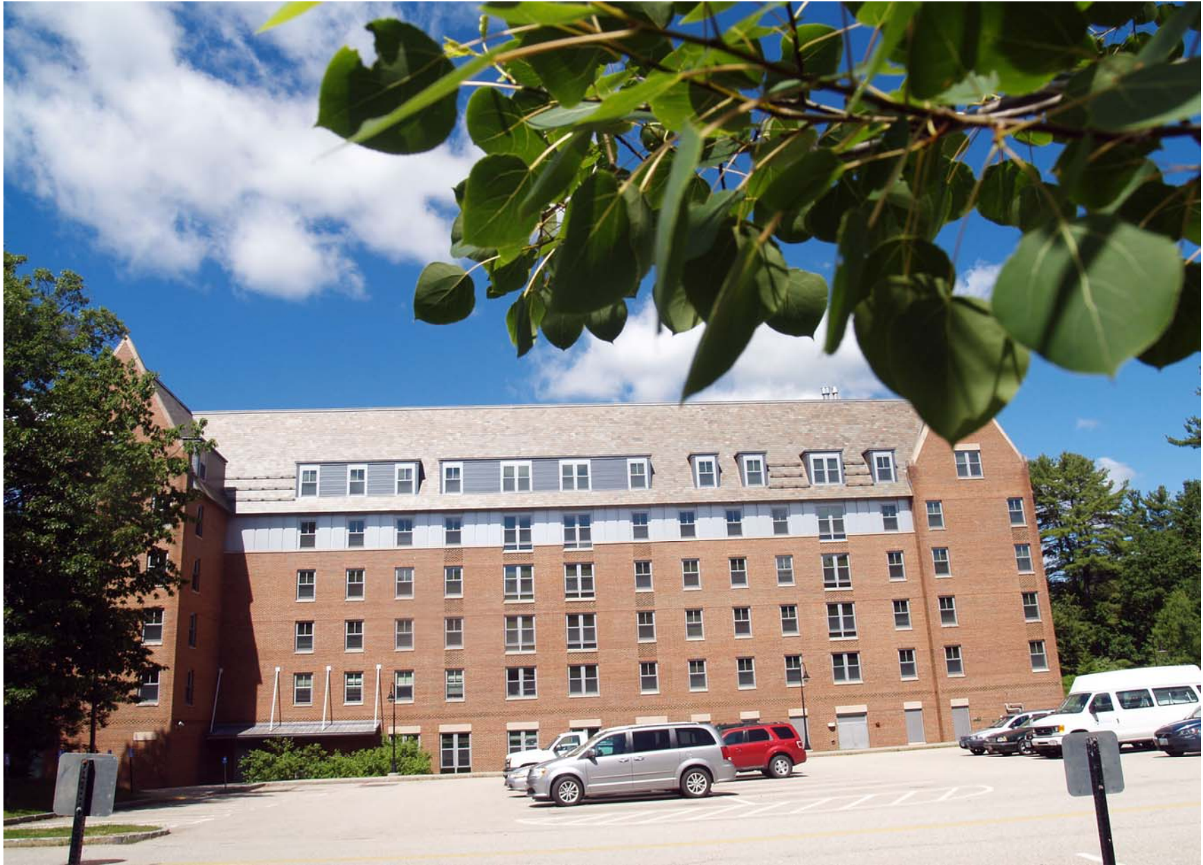
Photo #45—LOCATION L-1. (UNH—Gables North Parking-) looking west at Gables North Building from proposed project—June, 2017
