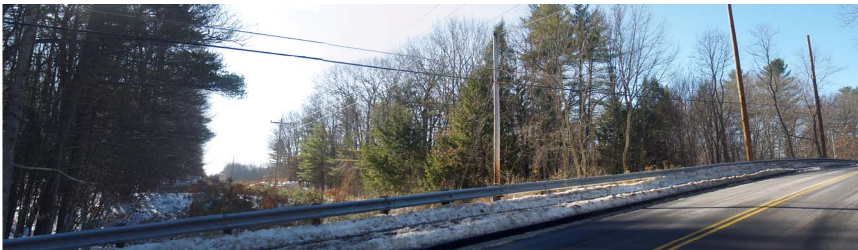
Photo #29—LOCATION H1 (Mill Road Crossing) looking south along proposed project—December, 2017—panorama
