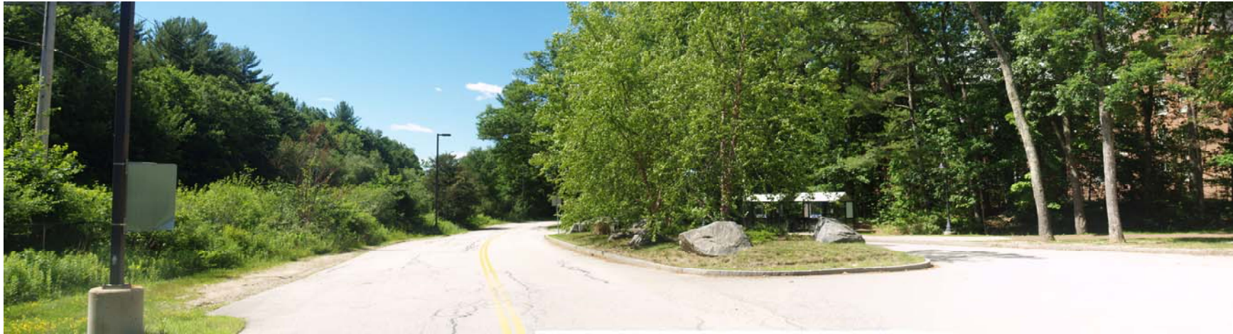
Photo #43—LOCATION K3 (UNH—Gables Apartment Complex) looking south along proposed project—June, 2017—panorama
