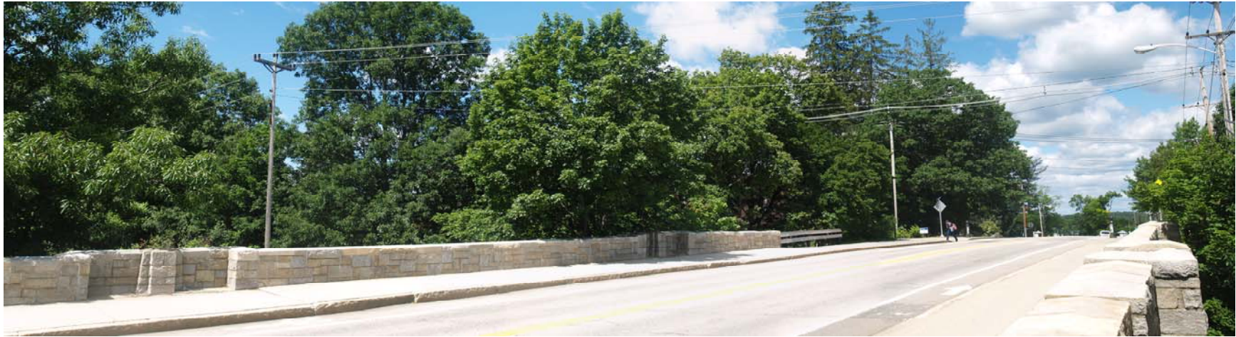
Photo #36—LOCATION J1. (UNH—Main Street Overpass) looking southwest toward proposed project—June, 2017—panorama
