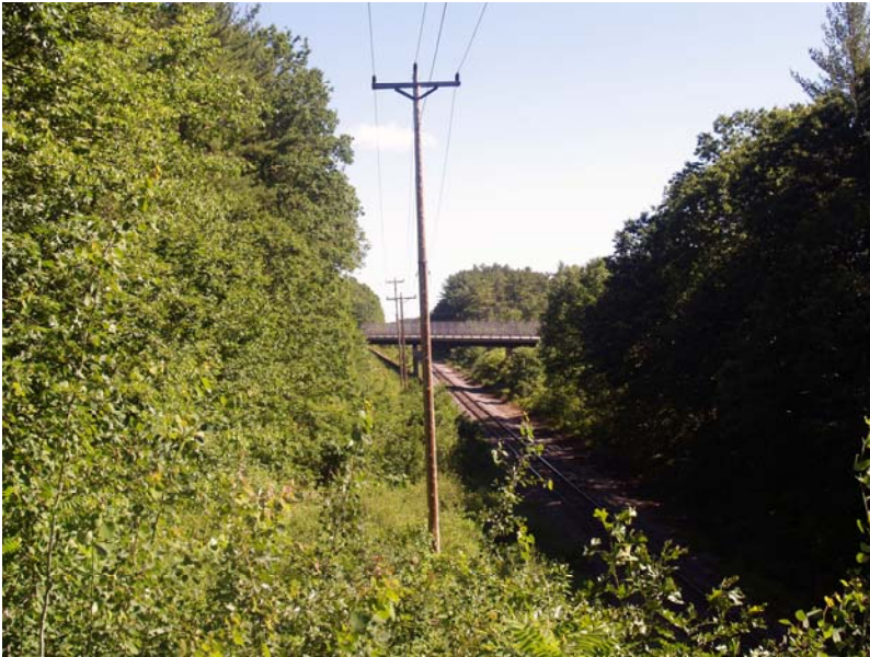
Photo #51—Location M-3. (Route 4 crossing) looking south from railroad overpass —June— 2017— 55mm eq. 60 ft. to be cleared left of existing pole
