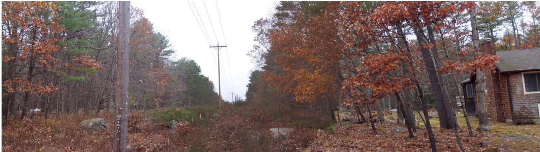
Photo #25—LOCATION F2 (Cutts Road) looking west along proposed project—November, 2016 panorama
