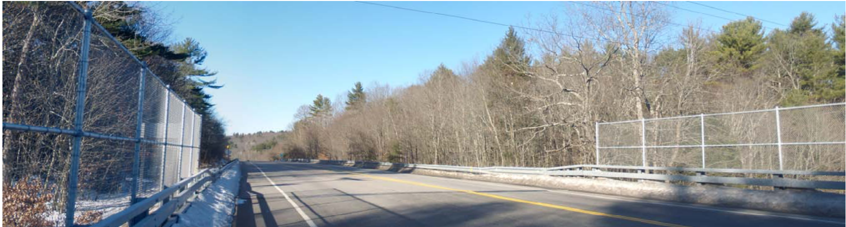
Photo #49—Location M-1. (Route 4 crossing) looking west —December— 2016— panorama
