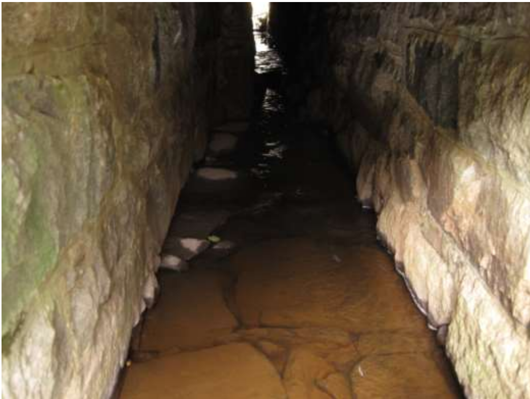
Image 34: Granite paving stones lining the floor of the culvert
