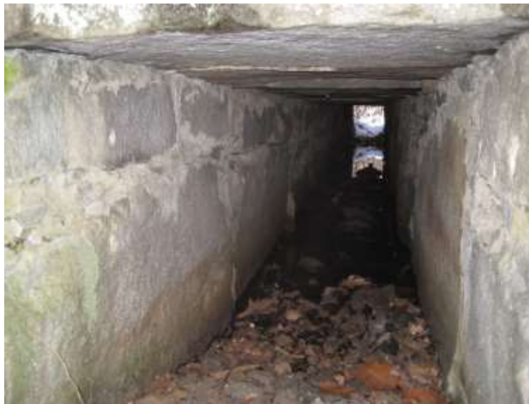
Image 36: granite culvert beneath the railroad embankment
