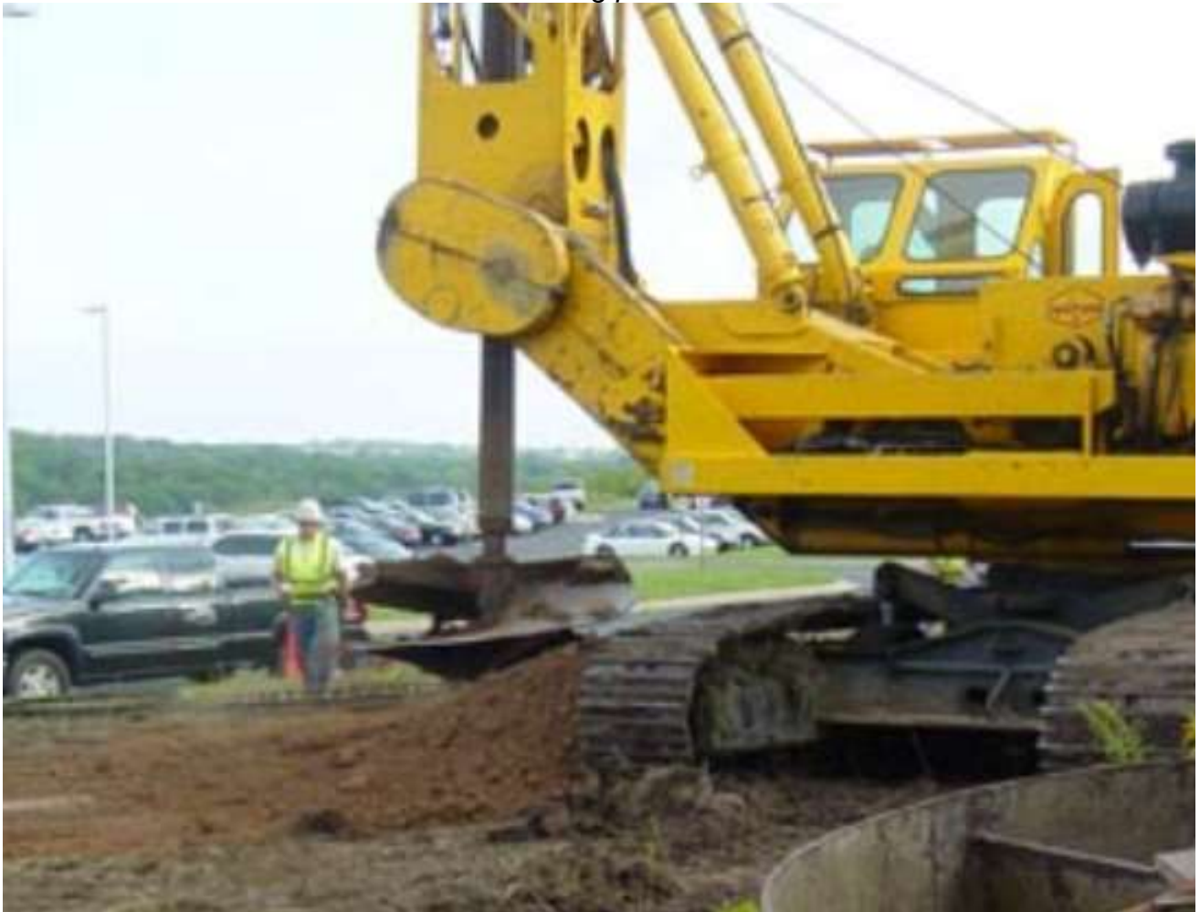
Auger on continuous-tracked equipment
