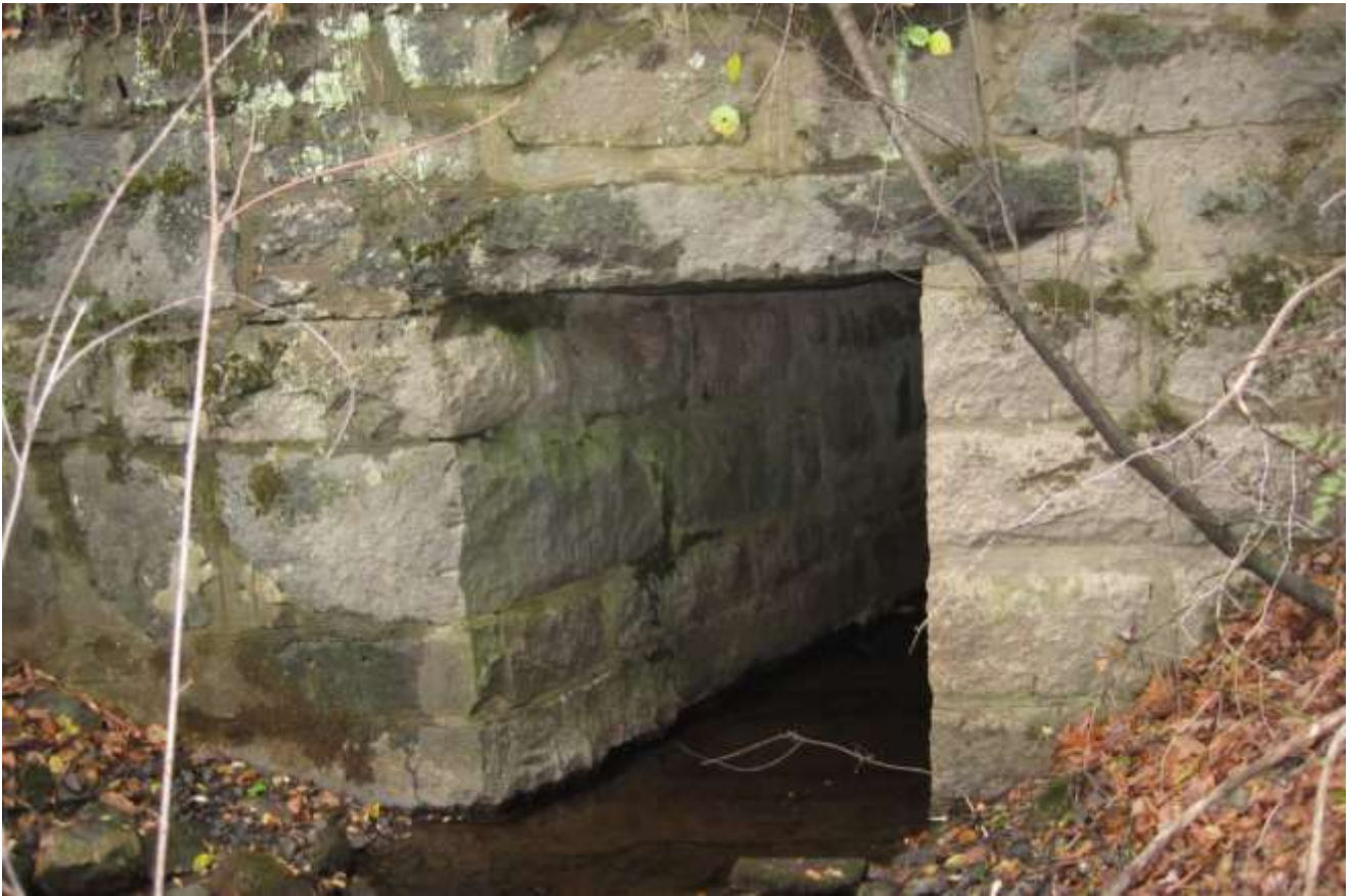
Image 33: 19 th century granite railroad bridge crossing LaRoche Brook
