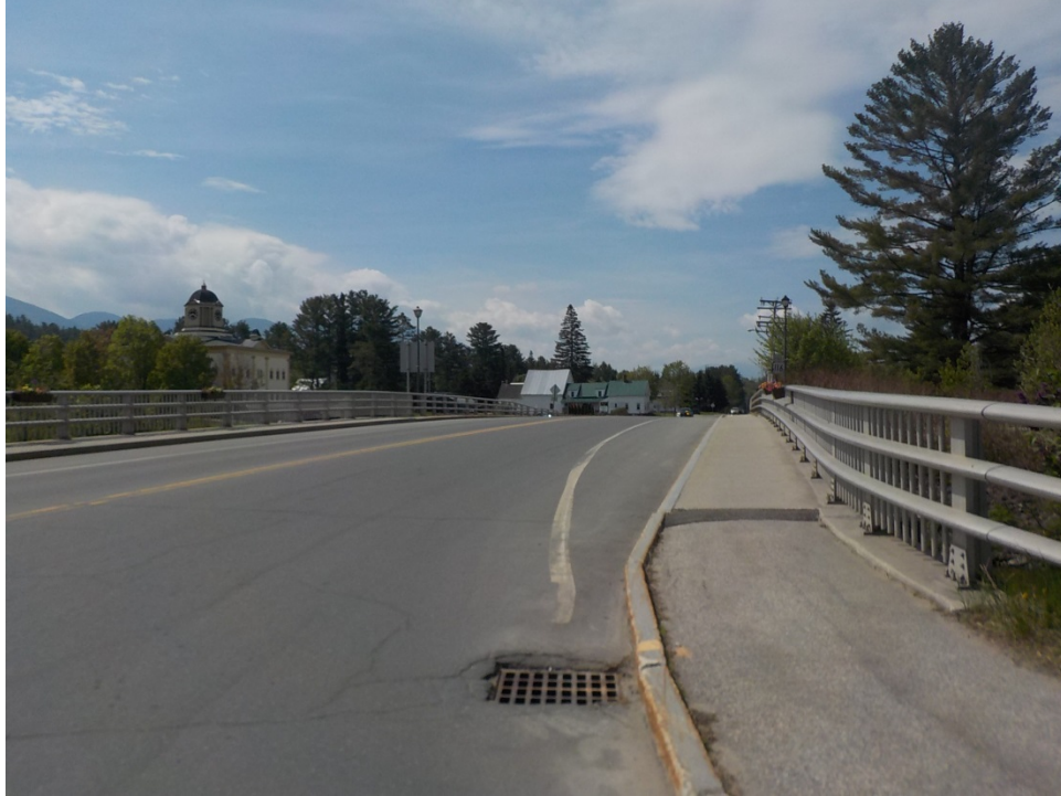
Photo 3. NPT line will be directionally-drilled under the Gale River in Franconia, NH as part of the Underground Line (UG1). This is the bridge over the Gale River in the location of rt 116 where the underground crossing will occur.
