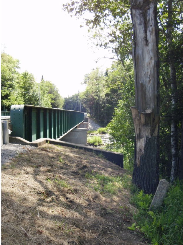
Photo 3. The Northwest quadrant of the Connecticut River/Route 3 Crossing, looking southwest. The underground cable will be directionally drilled under the river bed, river bank, and this portion of the Protected Shoreland.
