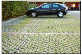
Paver grids in light-duty parking areas are installed with a soil medium that supports plant growth and infilitrates runoff.
