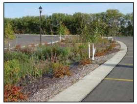
A depressed swale with plants tolerant of wet and dry conditions captures and treats runoff from the adajcent parking areas (examples above and below).
