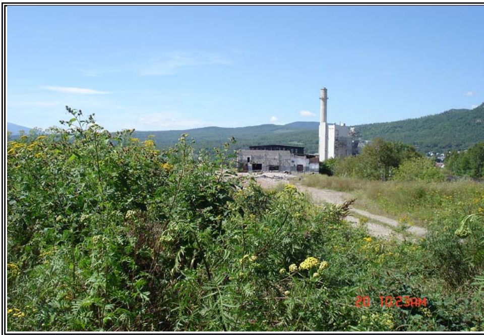
Photograph No. 10: View looking towards the west.
