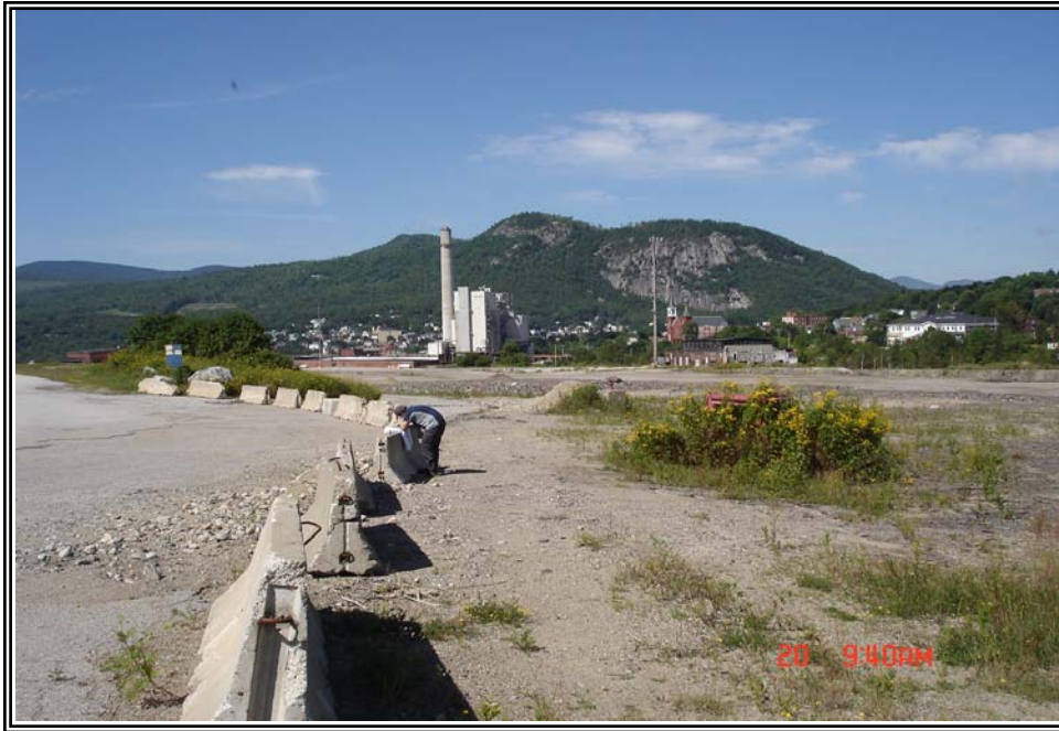
Photograph No. 3: View looking towards the west. Existing facility in foreground.
