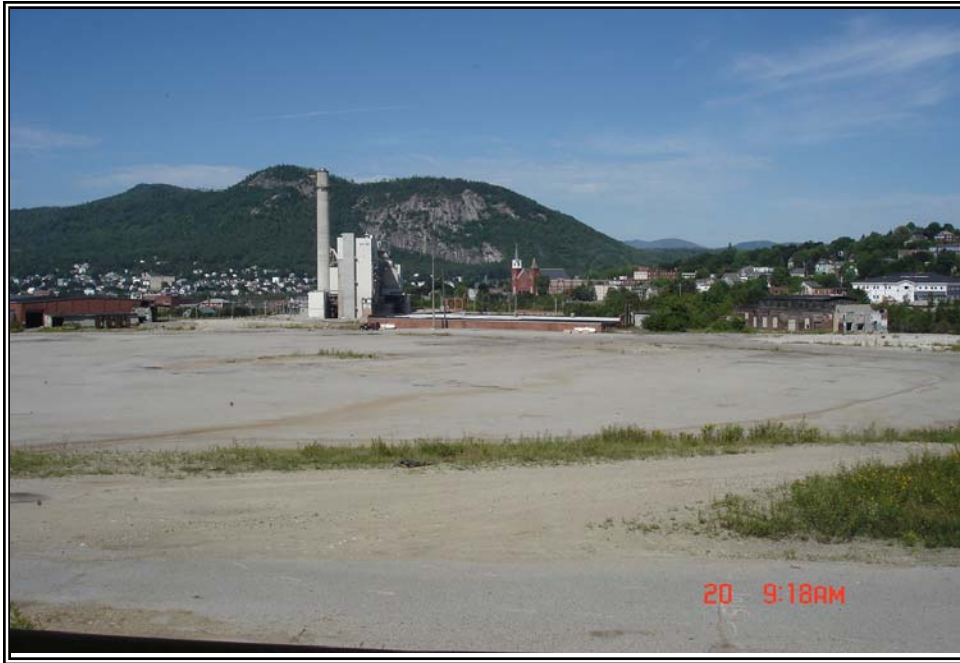
Photograph No. 1: View looking westerly towards existing stack and facility.
