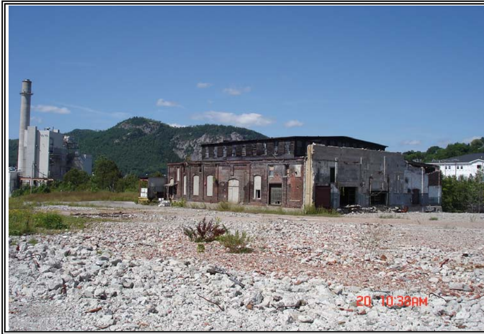
Photograph No. 7: View looking northerly towards the existing building along the Androscoggin River.
