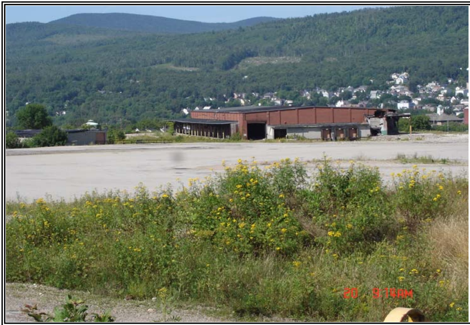
Photograph No. 2: View looking towards the west.
