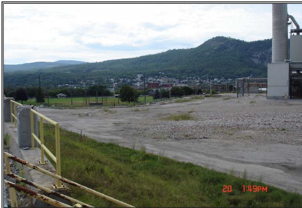
Photograph No. 6: View looking towards the southwest.
