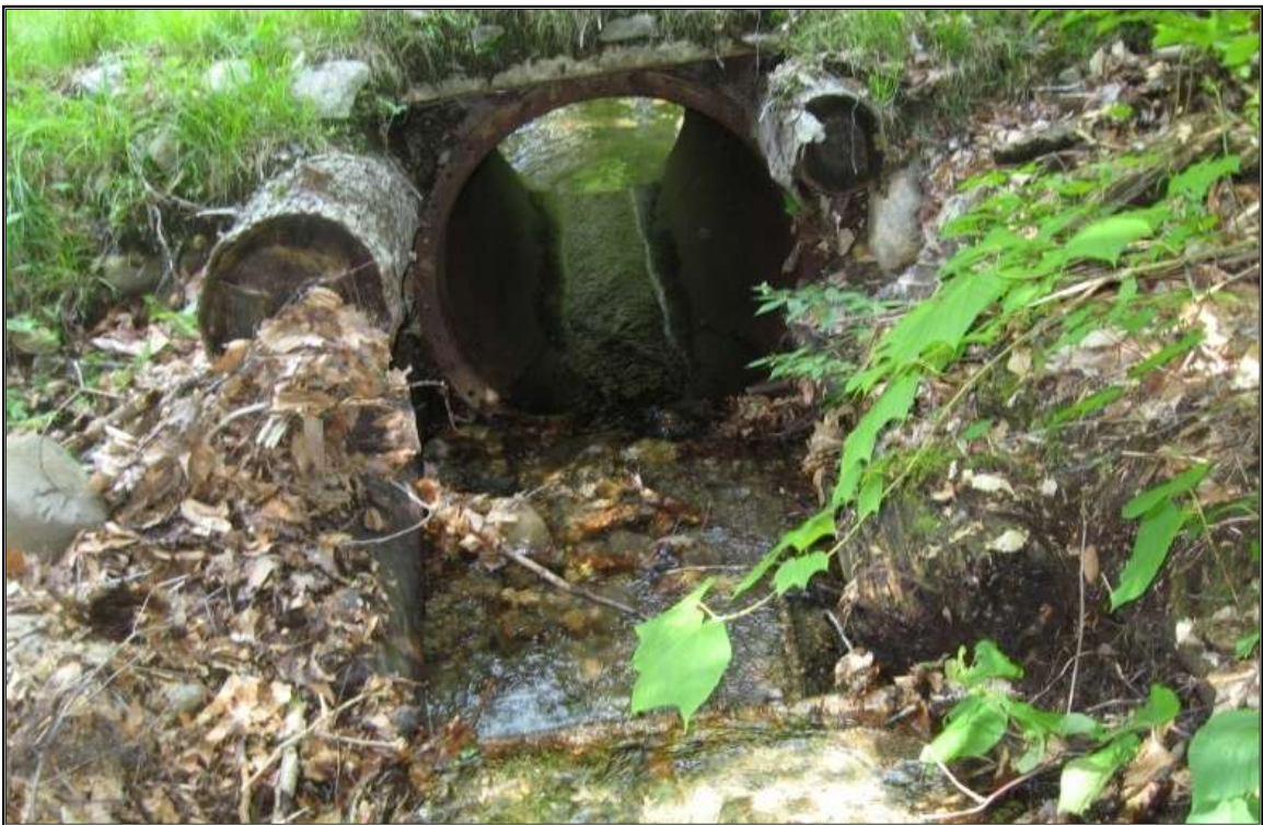
Photo 48: Unobstructed large culverts provide good passages/ corridors for a diverse species of wildlife.
