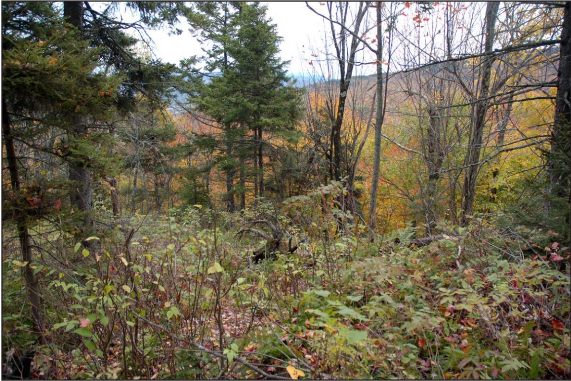
PLATE 15: Excess Slope Around Turbine W1
