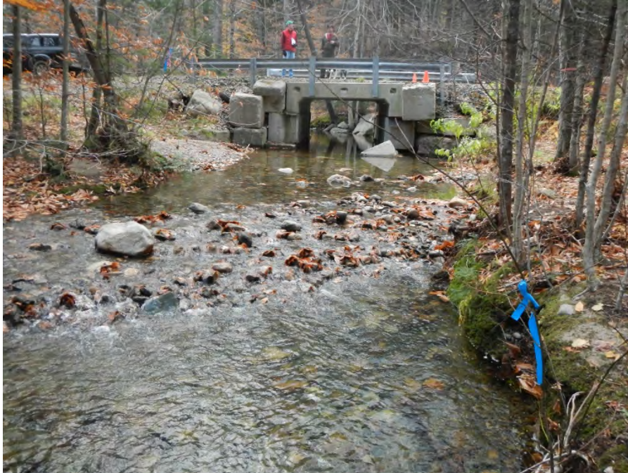
Photo 7. Pre- Emergency Authorization - Looking upstream toward bridge.
