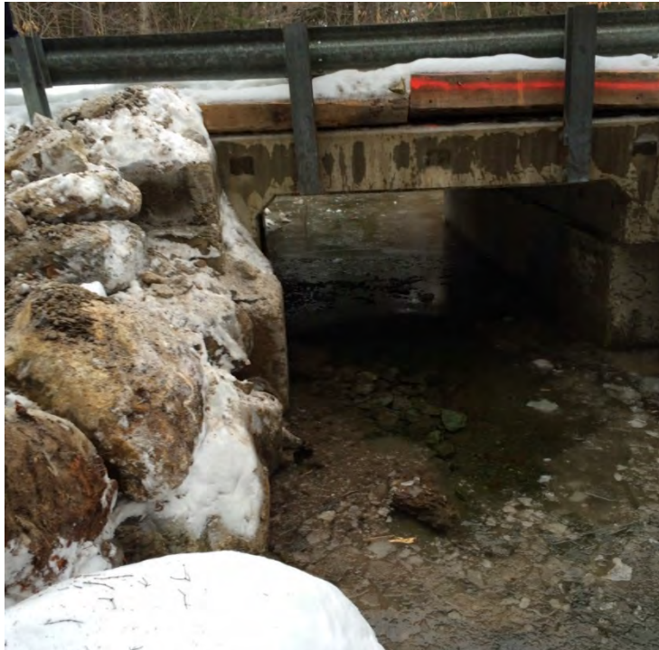
Photo 12. Post- Emergency Authorization – Looking downstream along abutment #1
