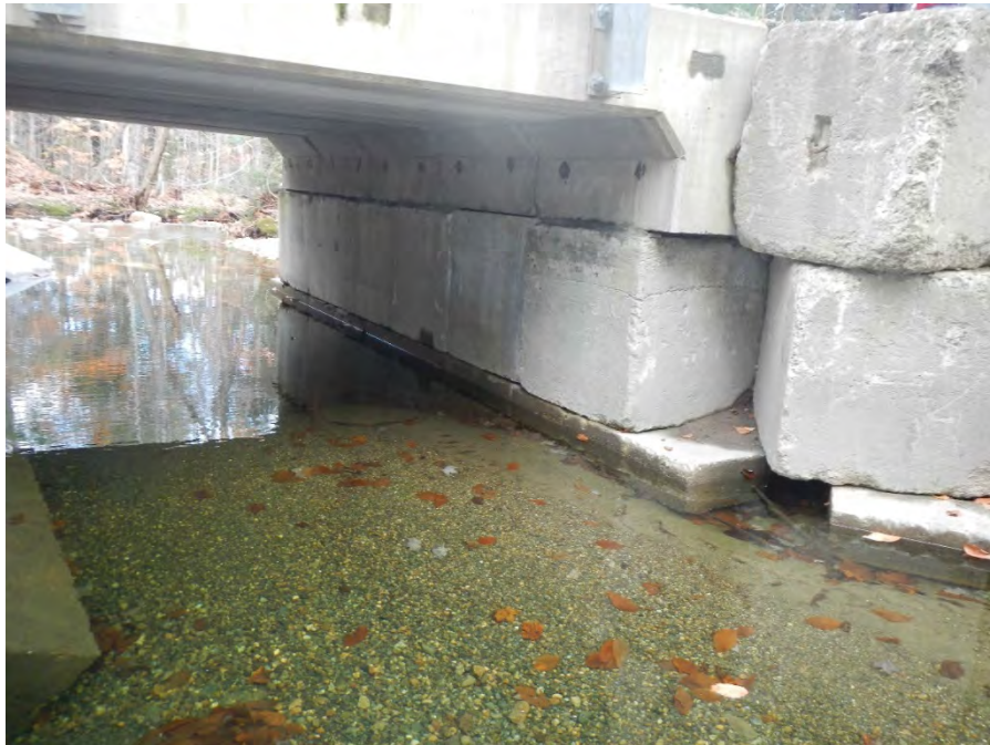
Photo 4. Pre- Emergency Authorization - Looking downstream along abutment #2
