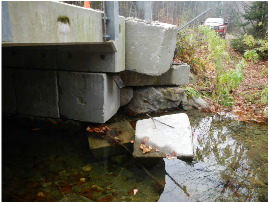
Photo 2: Pre-Emergency Authorization - Looking west at Northwest corner of abutment #1 (downstream side)
