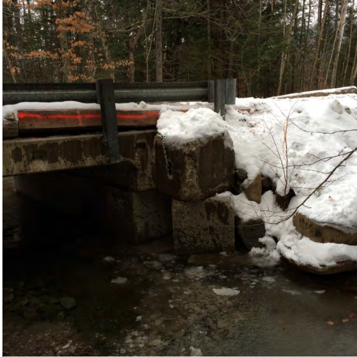
Photo 11. Post- Emergency Authorization - Looking downstream along abutment #2
