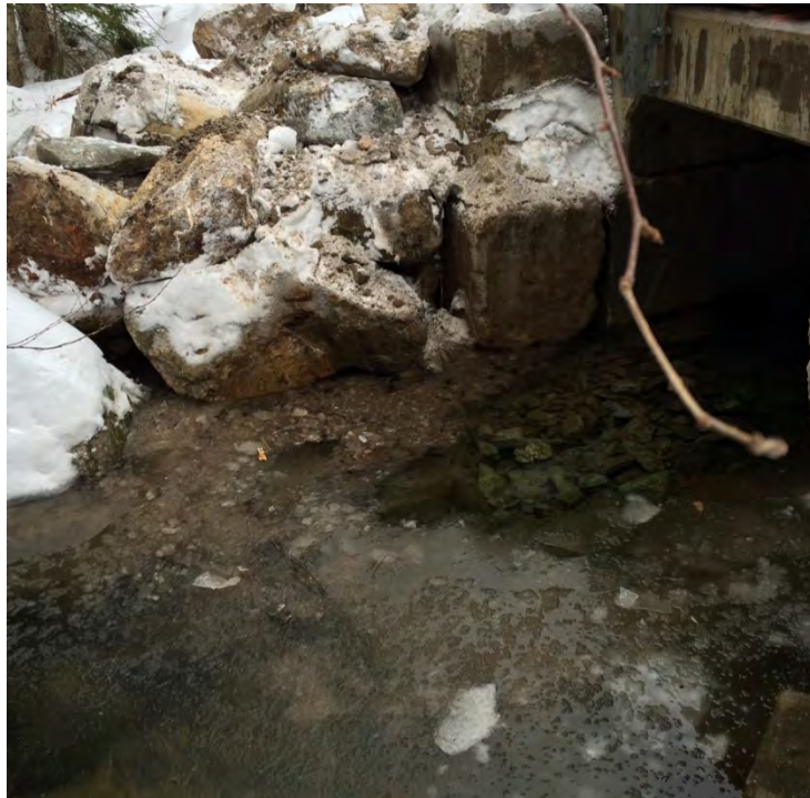
Photo 10. Post- Emergency Authorization - Looking north at the southwest corner of abutment #1 (upstream side)
