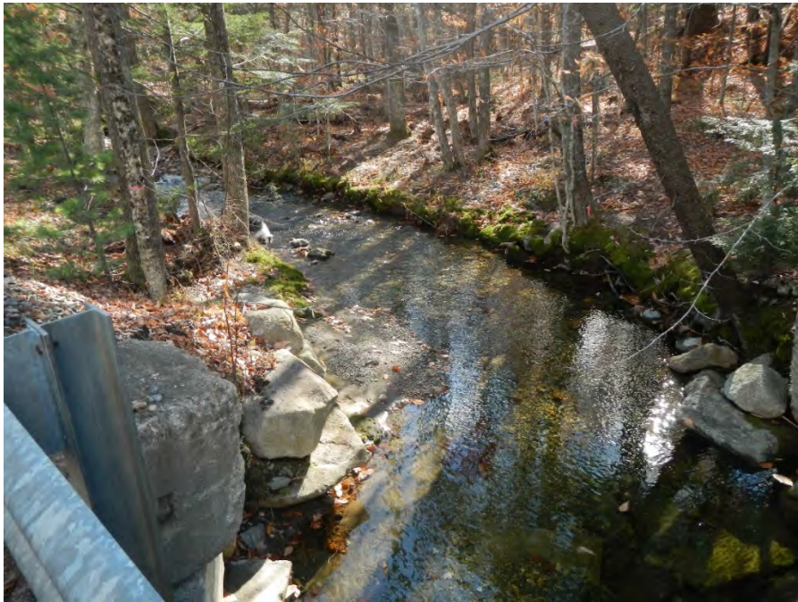
Photo 6. Pre- Emergency Authorization - Looking upstream from bridge.
