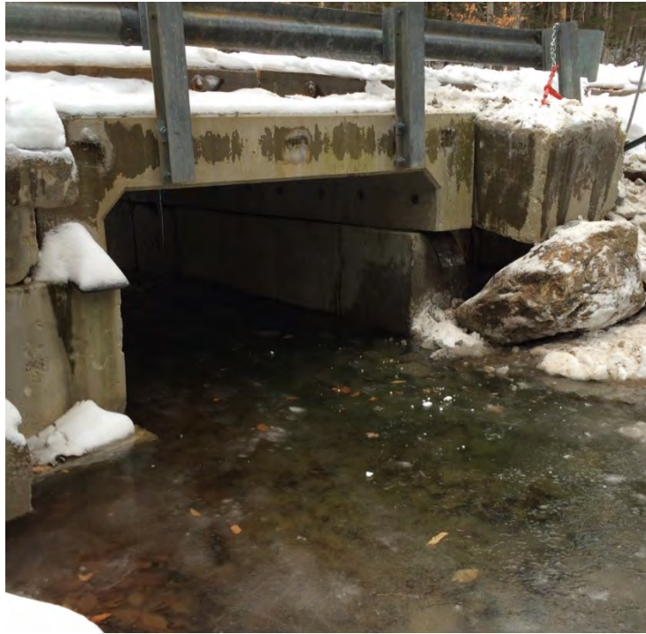
Photo 9. Post- Emergency Authorization - Looking west at Northwest corner of abutment #1 (downstream side).
