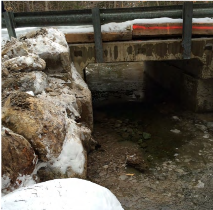
Photo 12. Post- Emergency Authorization – Looking downstream along abutment #1
