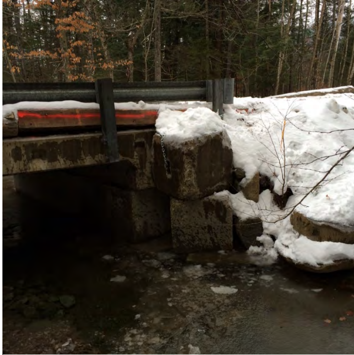
Photo 11. Post- Emergency Authorization - Looking downstream along abutment #2
