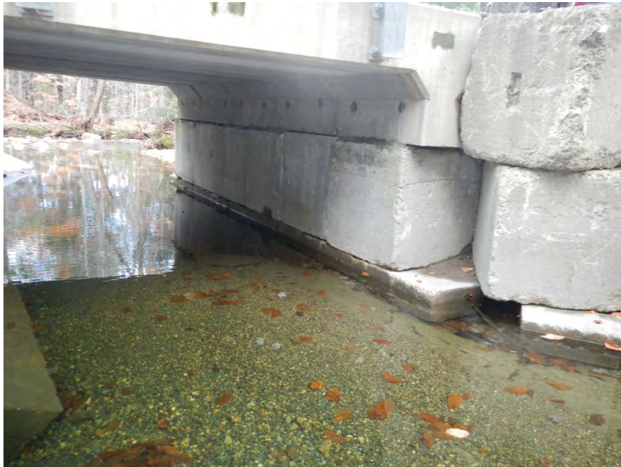
Photo 4. Pre- Emergency Authorization - Looking downstream along abutment #2
