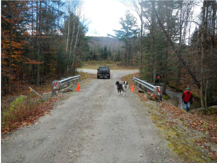
Photo 1: Pre-Emergency Authorization- Looking southeast along Groton Hollow Road, Upper Bridge Crossing of Clark Brook.
