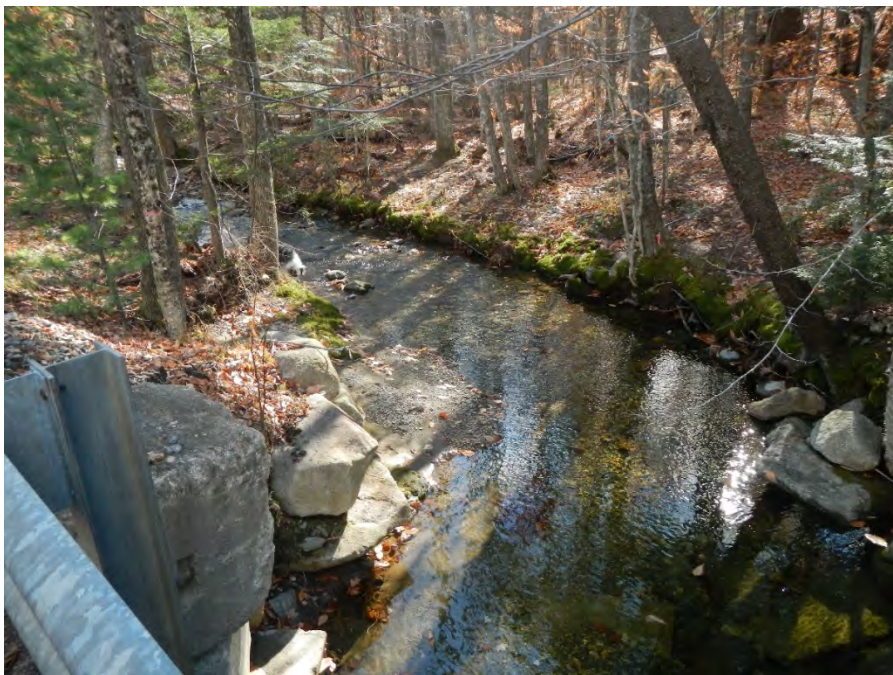
Photo 6. Pre- Emergency Authorization - Looking upstream from bridge.
