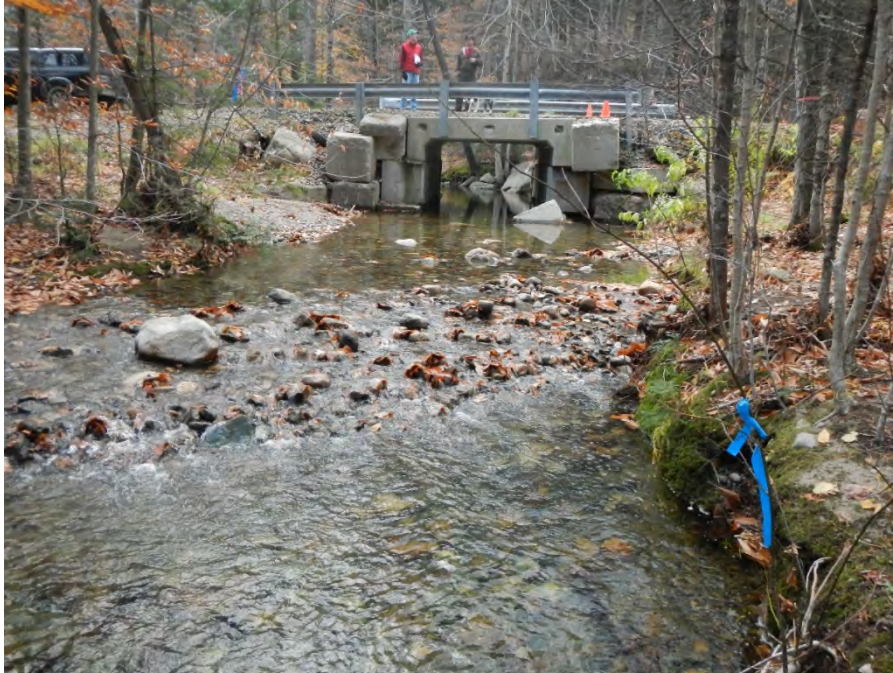
Photo 7. Pre- Emergency Authorization - Looking upstream toward bridge.
