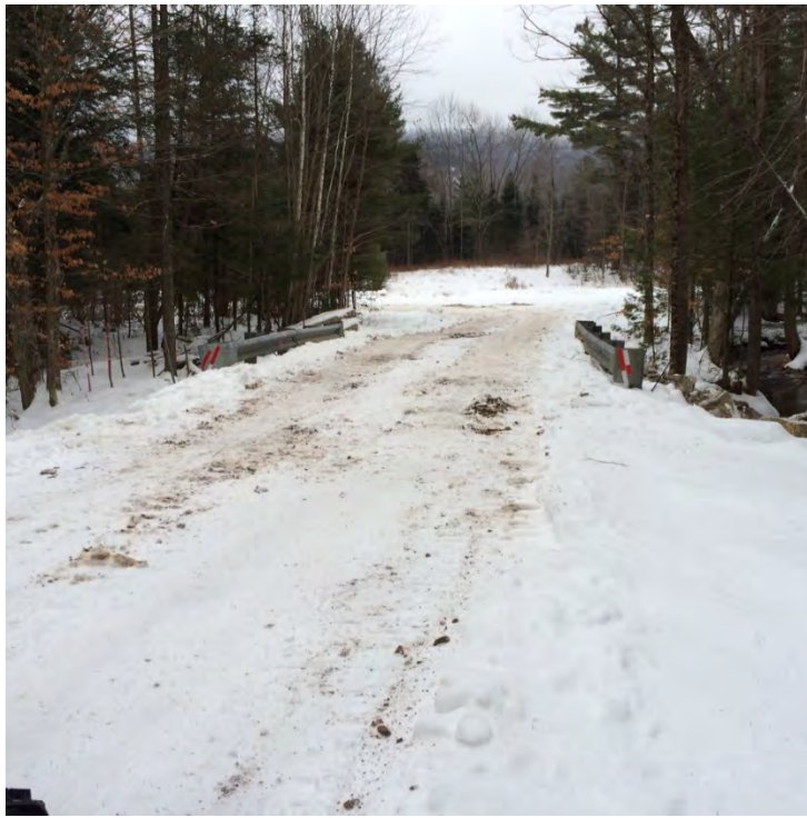
Photo 8. Post- Emergency Authorization - Looking southeast along Groton Hollow Road, Upper Bridge Crossing of Clark Brook
