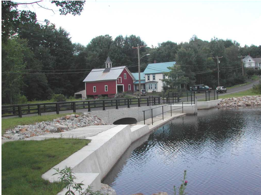
Summer Street Bridge
