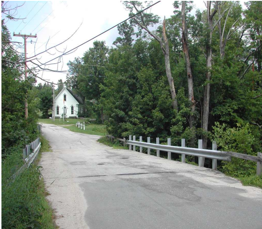
The oldest bridge in Antrim, on Old North Branch Road
