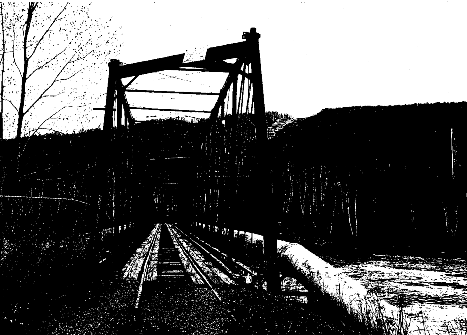
PHOTO # 15 Subject: Whipple Truss Bridge - Cascade Berlin Mills Railway, GORHAM West Portal Photographer facing: NE Roll # 1 Frame # 23
