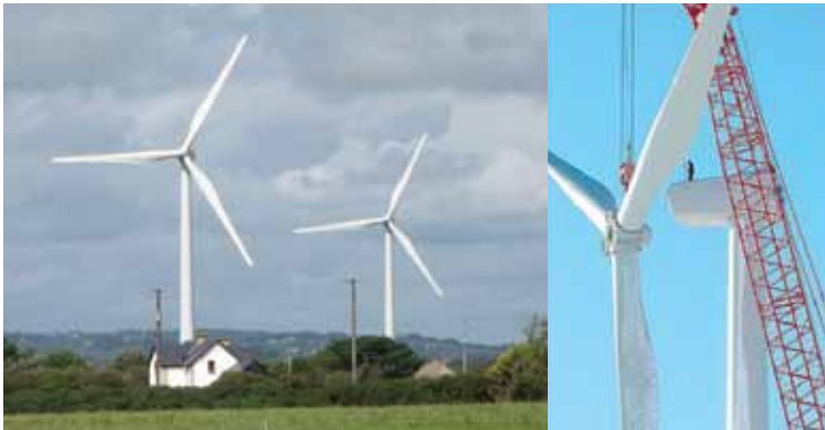
LEFT: Wind Power in Residential Area. RIGHT: Turbine Construction
