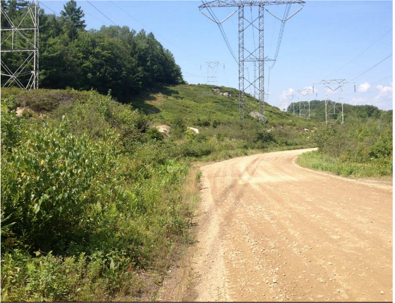
PHOTO WAS TAKEN FROM BOG ROAD. PHOTO IS OF THE ENTRANCE AREA TO THE PROPOSED SUBSTATION AND INTERCONNECTION STATION. PHOTO LOCATION IS JUST TO THE SOUTH OF THE ENTRANCE. PHOTO WAS TAKEN LOOKING NORTHERLY.
