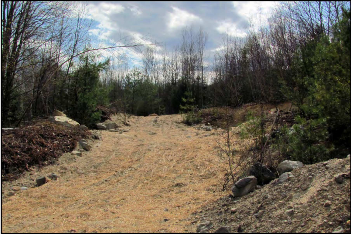
PLATE 26: Current Conditions Along Proposed Overhead Collector. View East
