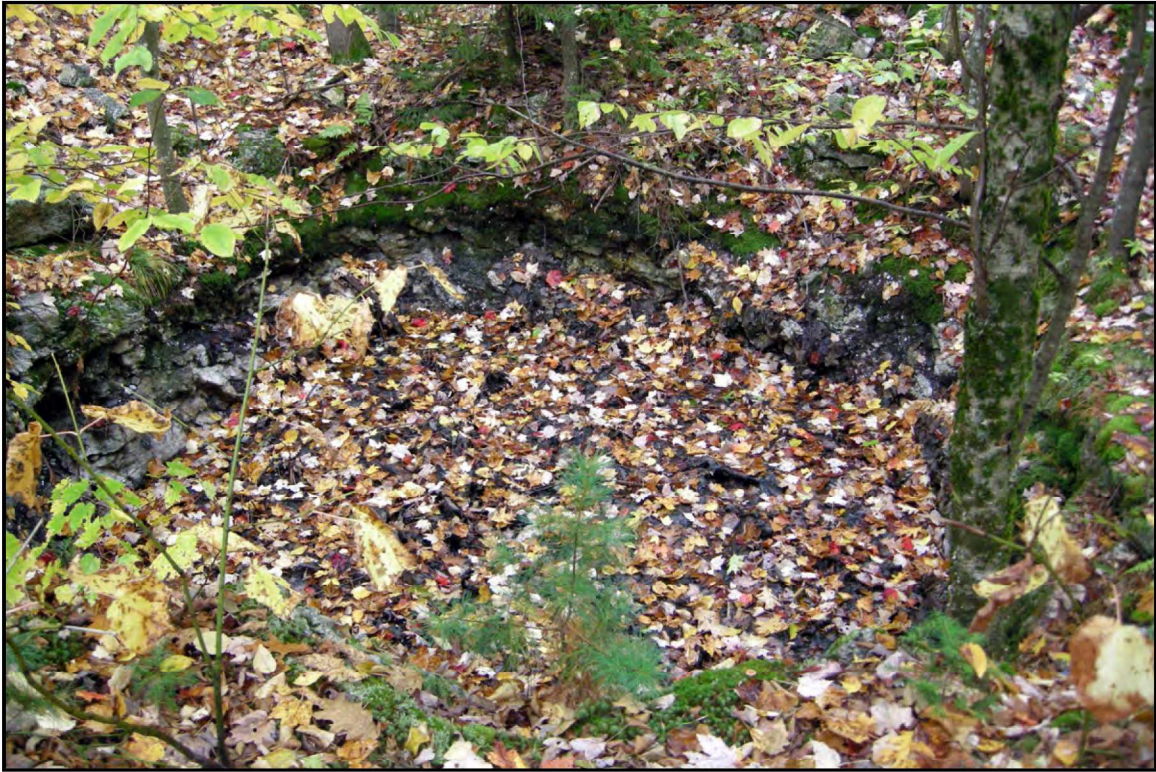
PLATE 13: Stone Foundation, TS-4980-08. View Northwest
