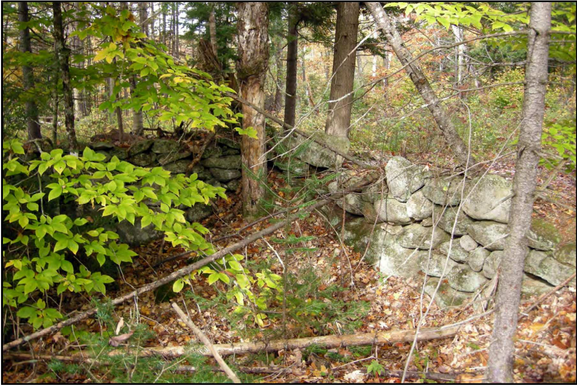
PLATE 7: Stone Foundation, TS-4980-03. View Southwest
