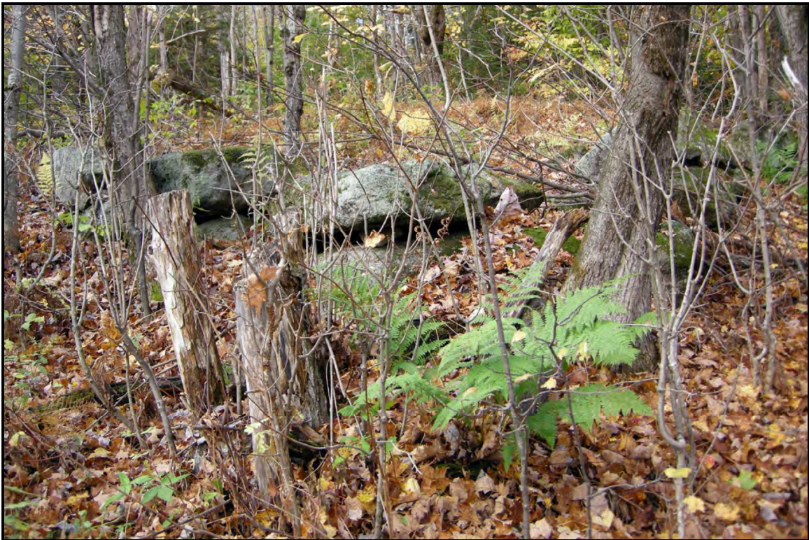
PLATE 19: Stone Retaining Wall, TS-4980-04. View West
