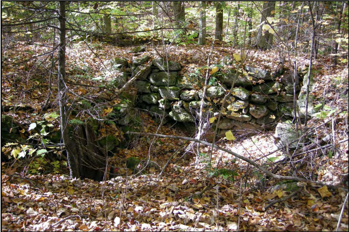
PLATE 15: Stone Foundation, TS-4980-07. View North
