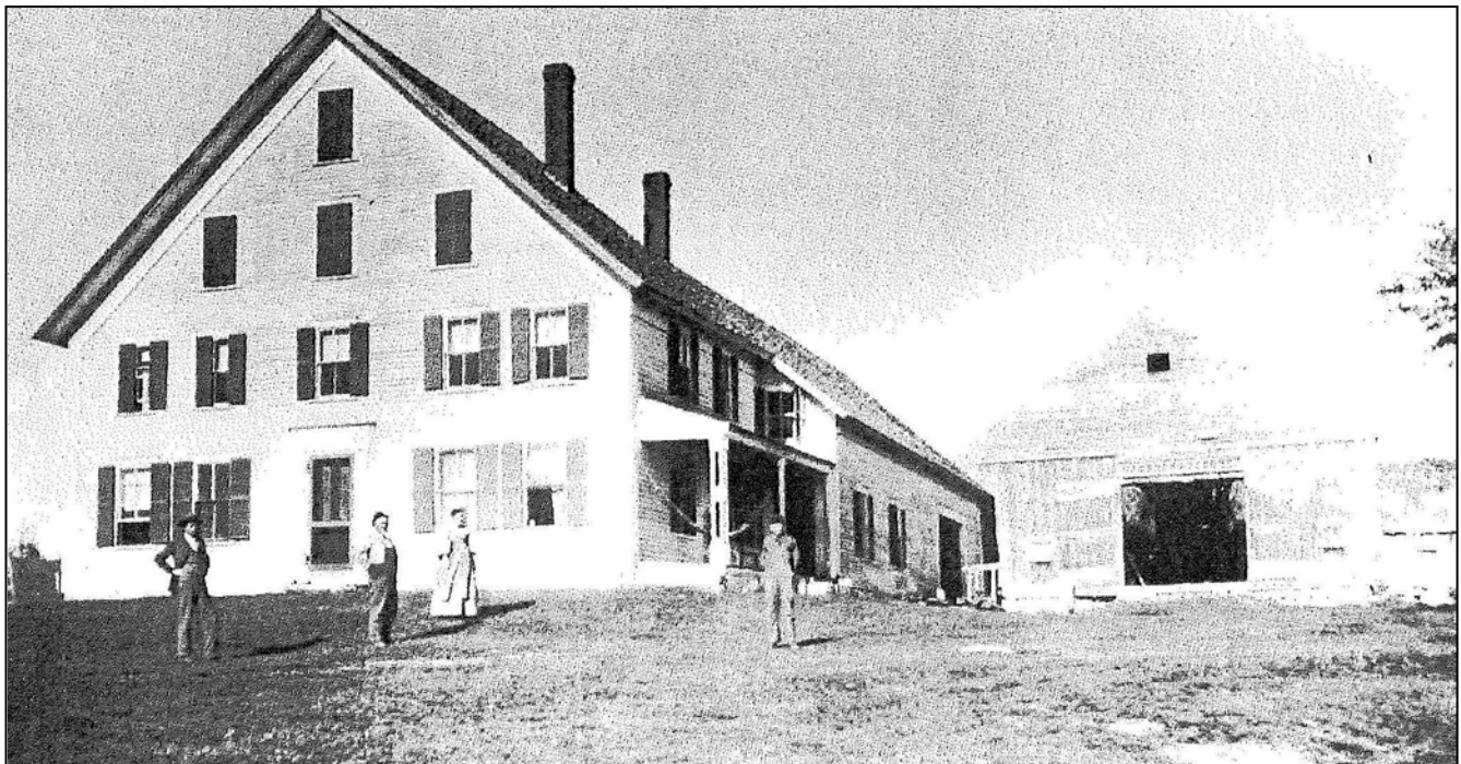
Danbury, Grace Ford House, 383 Eastern District Road, located near 3-Mile APE. Barn is not extant. Photograph date unknown. Danbury Bicentennial Committee, pg. 73.
