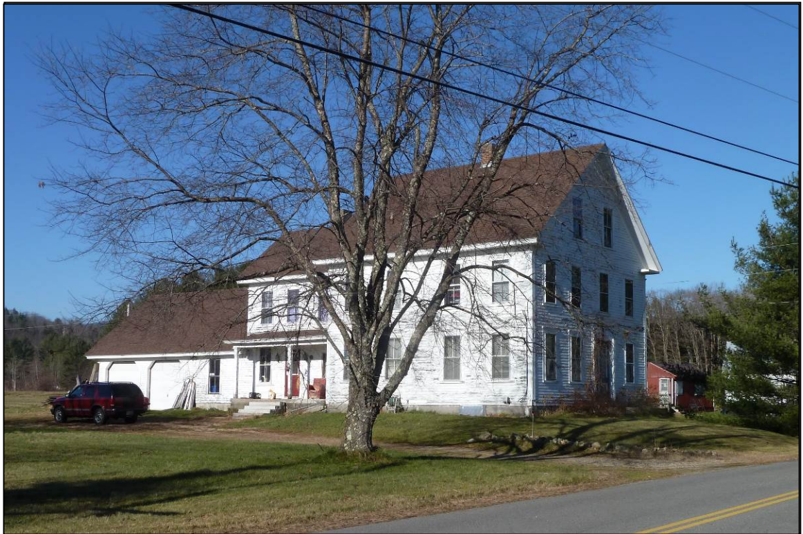
Photo 53 description: 517 Fowler River Road, Alexandria Roll: _____ Frame: _____ Direction: NW Date taken: 11-2012 Negative stored: _____
