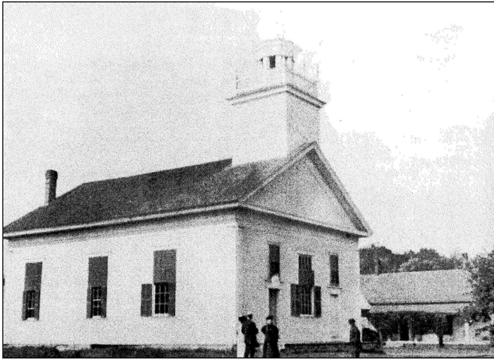
Danbury Center, Baptist Church of Danbury, constructed c. 1830, located outside 3-Mile APE. Photograph date unknown. Danbury Bicentennial Committee, pg. 16.
