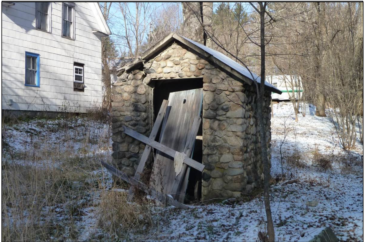
Photo 79 description: 54 Turnpike Road (springhouse), Grafton
