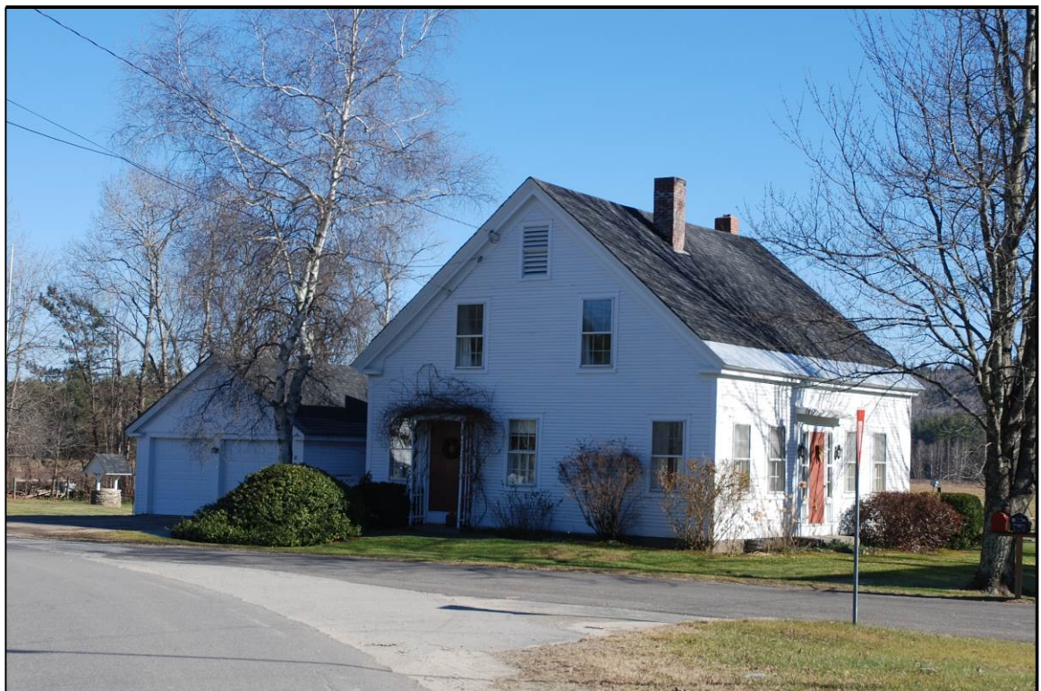
Photo 12 description: 10 North Road, Alexandria
