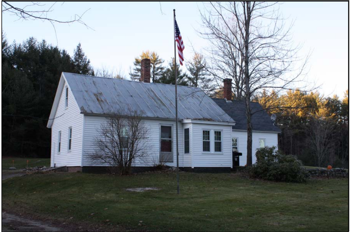
Photo 5 description: Karl Gordon Road, VHB-ALX-002, Alexandria
