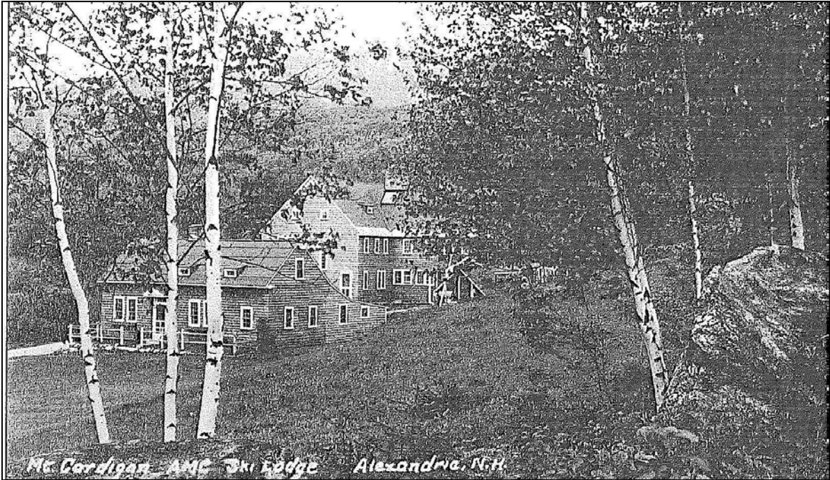
Alexandria, Cardigan Lodge, Shem Valley Road, constructed 1939 by Appalachian Mountain Club. Photograph date unknown. Lodge extensively renovated 2005. Hoflen and Hoflen, pg. 106.
