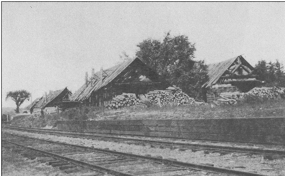
Grafton Village, Charcoal Kilns along railroad, located west of rail yard. No longer extant. Photograph date unknown. Cushing, pg. 206.
