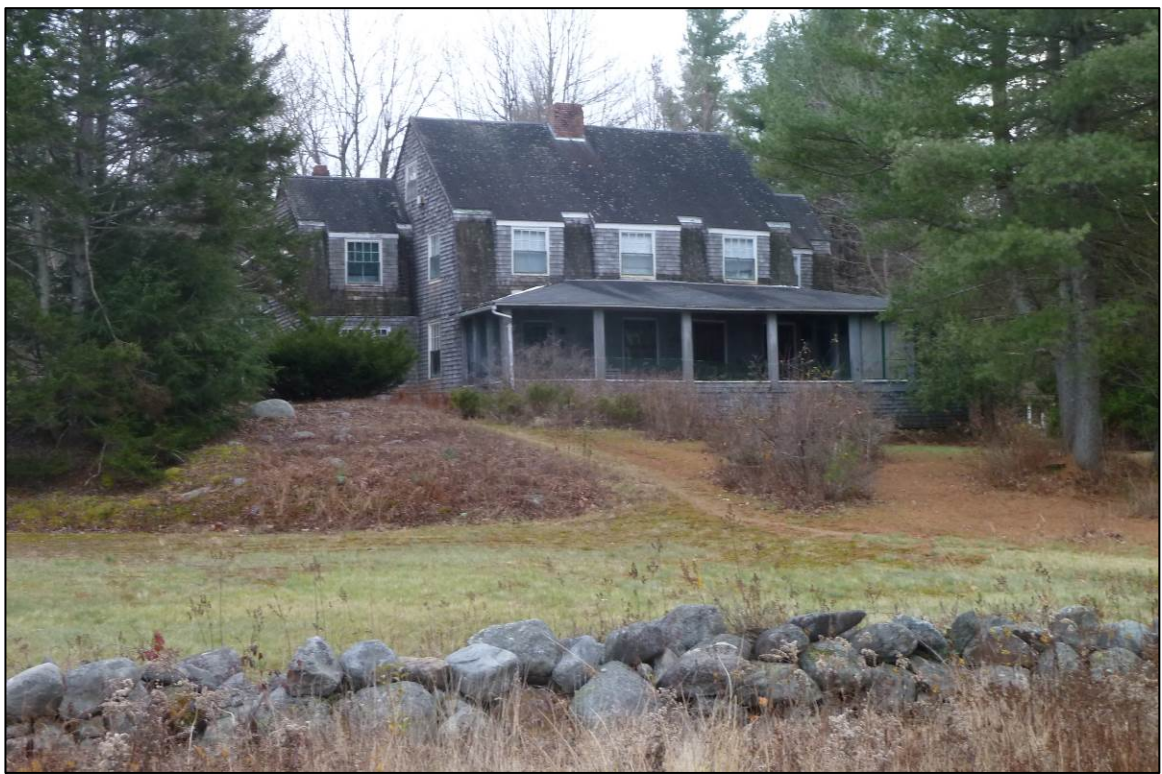
Photo 70 description: Murray Hill Road, VHB-HIL-003, Hill (Murray Hill Summer Home District) Roll: _____ Frame: _____ Direction: S Date taken: 11-2012 Negative stored: _____
