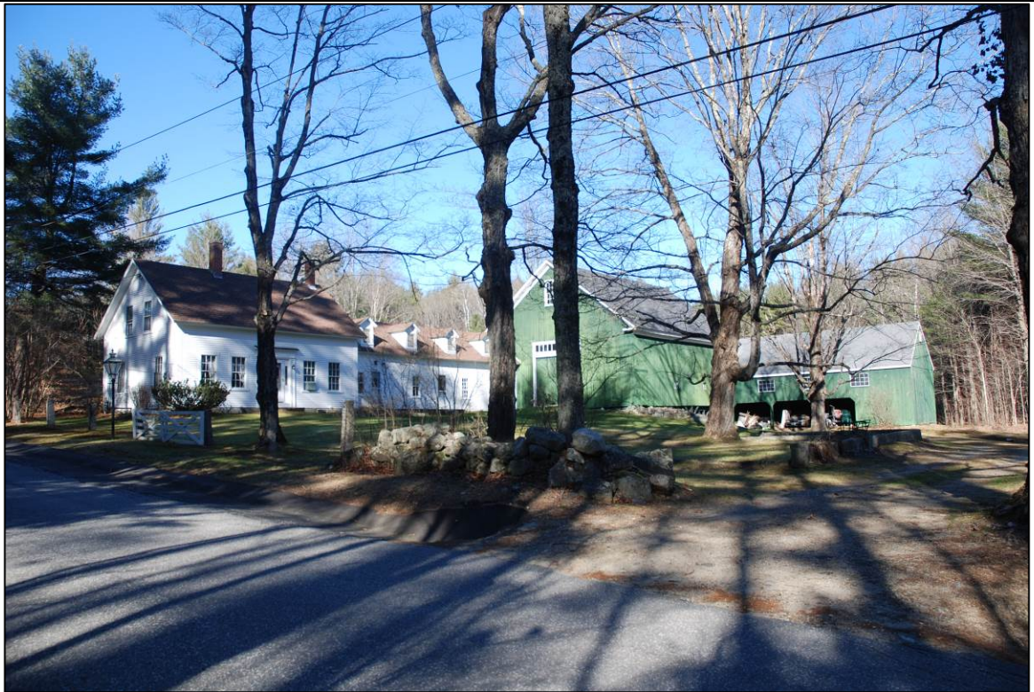
Photo 75 description: Mount Cardigan Road (barn), VHB-ALX-005, Alexandria Roll: _____ Frame: _____ Direction: N Date taken: 11-2012 Negative stored: _____
