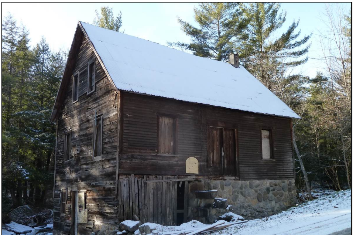
Photo 42 description: Hinkson's Carding Mill, Turnpike Road, VHB-GRA-005 (GRA0017), Grafton Roll: _____ Frame: _____ Direction: W Date taken: 12-2012 Negative stored: _____
