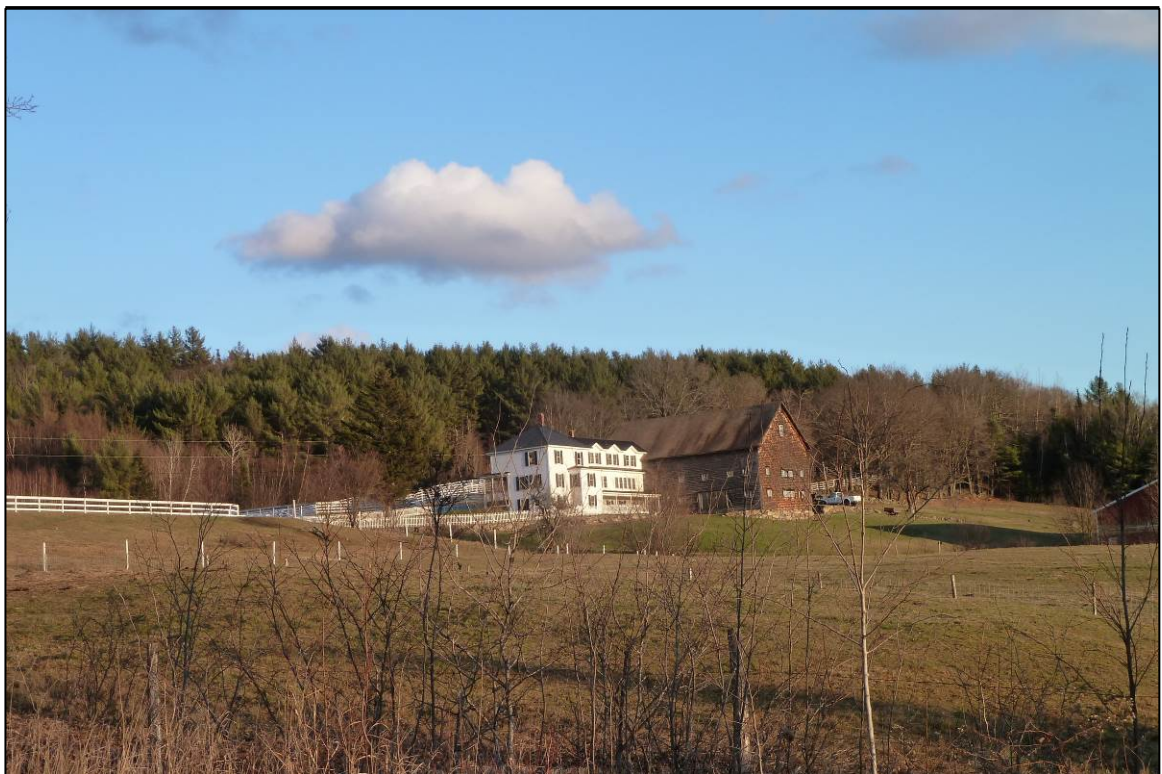
Photo 72 description: Eastern District Road, view of rear (SW elevation), VHB-DNB-005, Danbury Roll: _____ Frame: _____ Direction: E Date taken: 11-2012 Negative stored: _____
