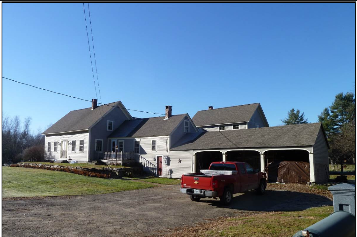
Photo 15 description: 178 Bailey Road, Alexandria
