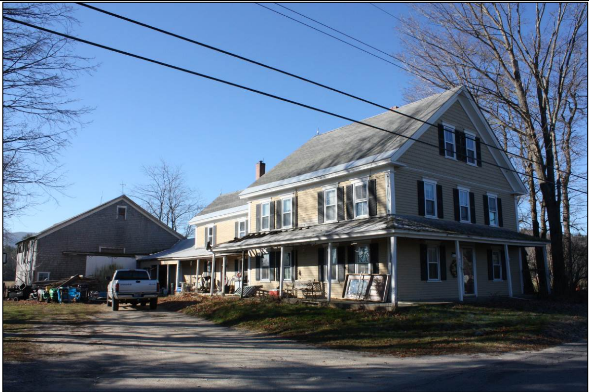
Photo 69 description: 441 Fowler River Road, Alexandria Roll: _____ Frame: _____ Direction: SW Date taken: 11-2012 Negative stored: _____
