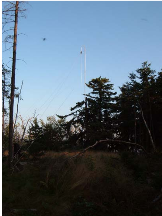
Photo 1. Melvin Mountain portable tower at the Wild Meadows Wind Project, 2010.
