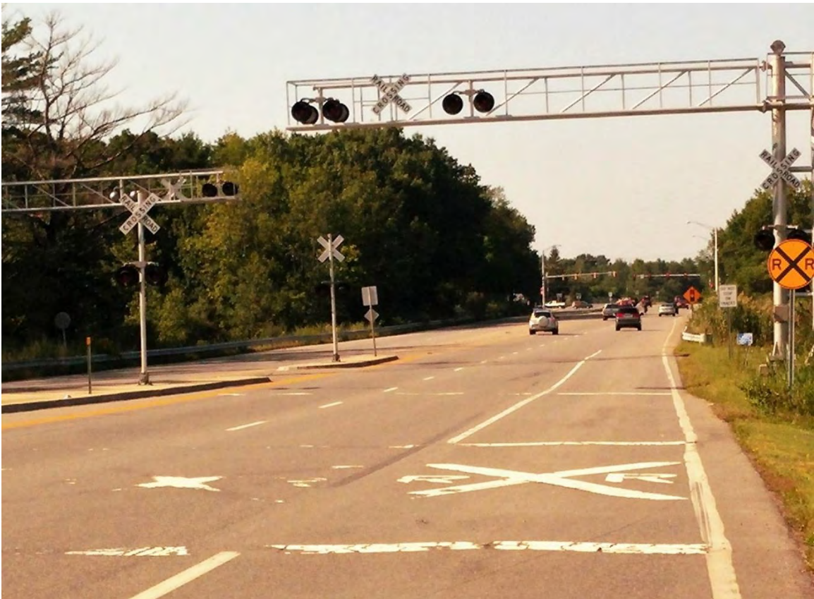
Greenland Rd - USDOT 054416P (no gates)
