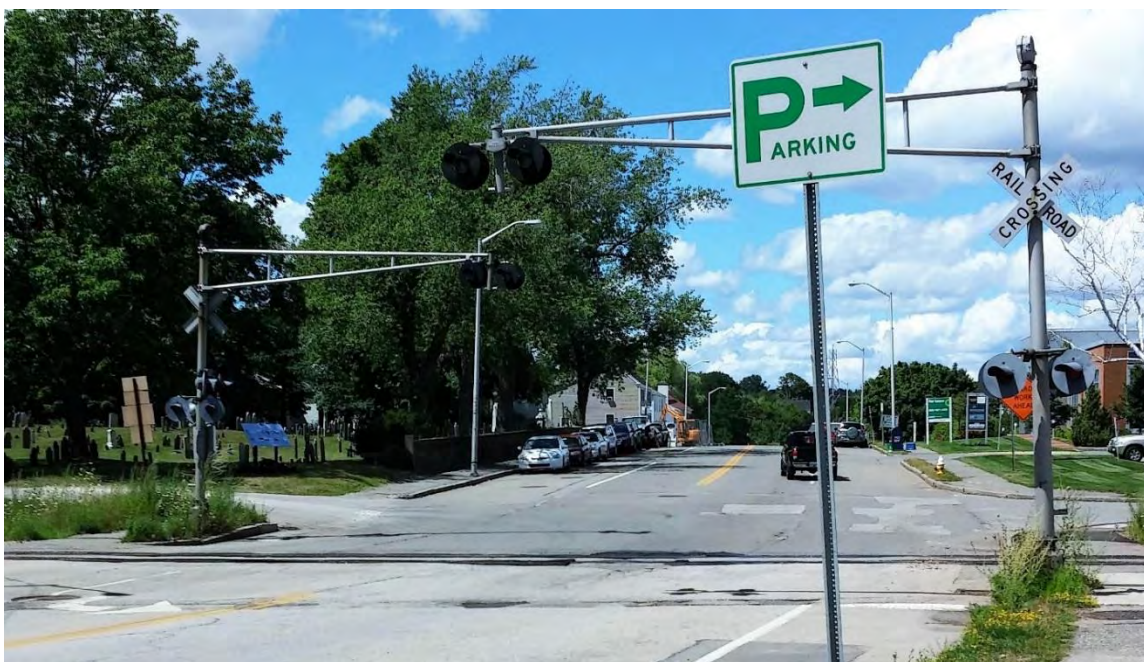
Maplewood Ave. – USDOT 054122E (no gates)
