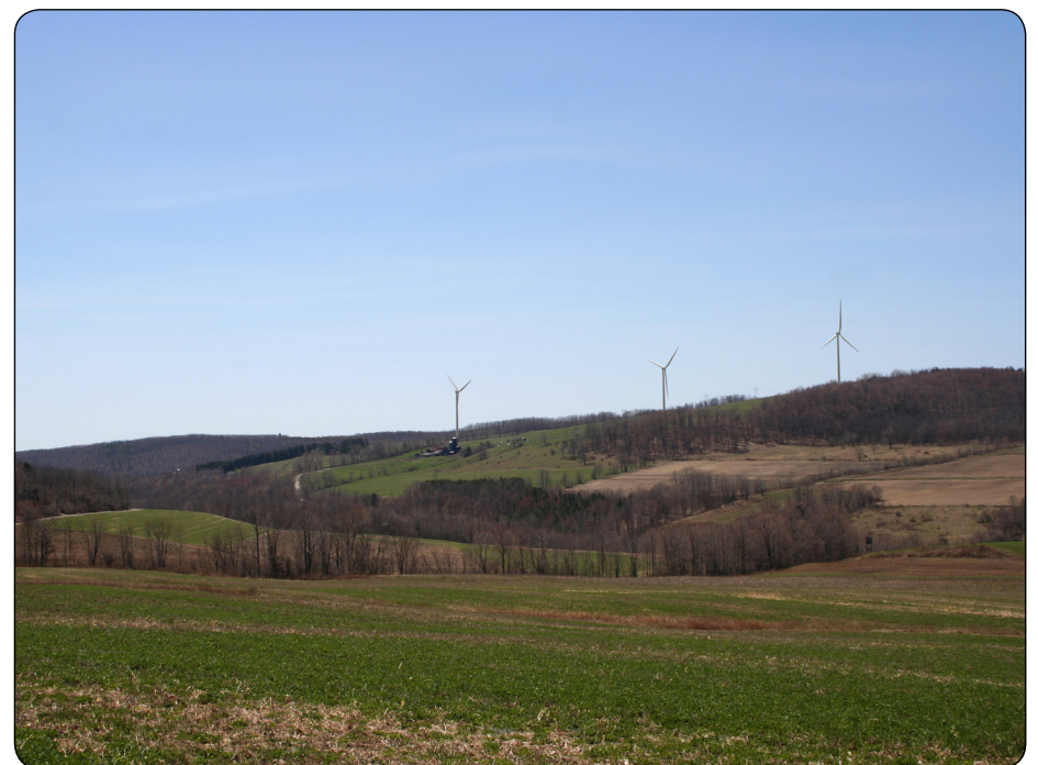
The proposed exterior color/finish of the turbines was then added to the model and the appropriate sun angle is simulated based on the specific date, time and location (latitude and longitude) at which each photo was taken.
