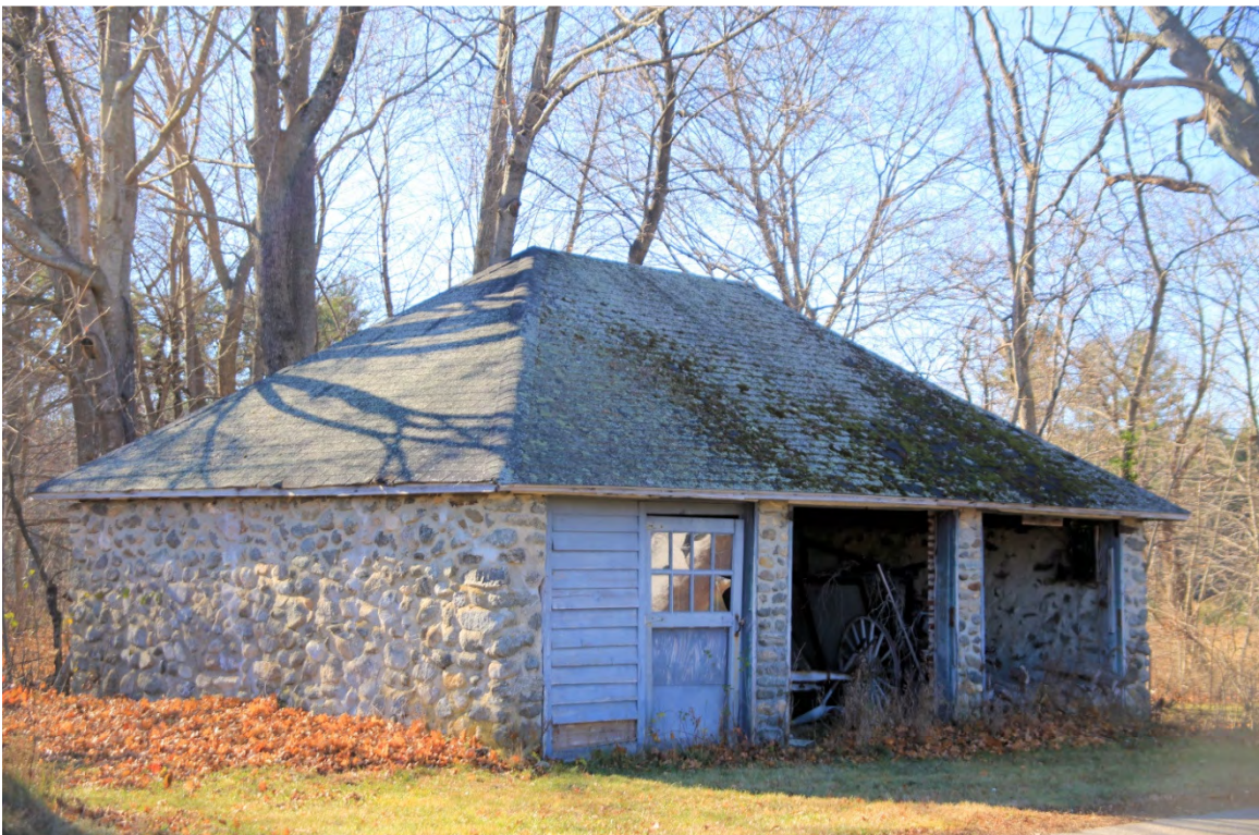
Photo 016) Perkins Road – Garage, Roselawn Farm ID: M-20, photo taken November 2015
