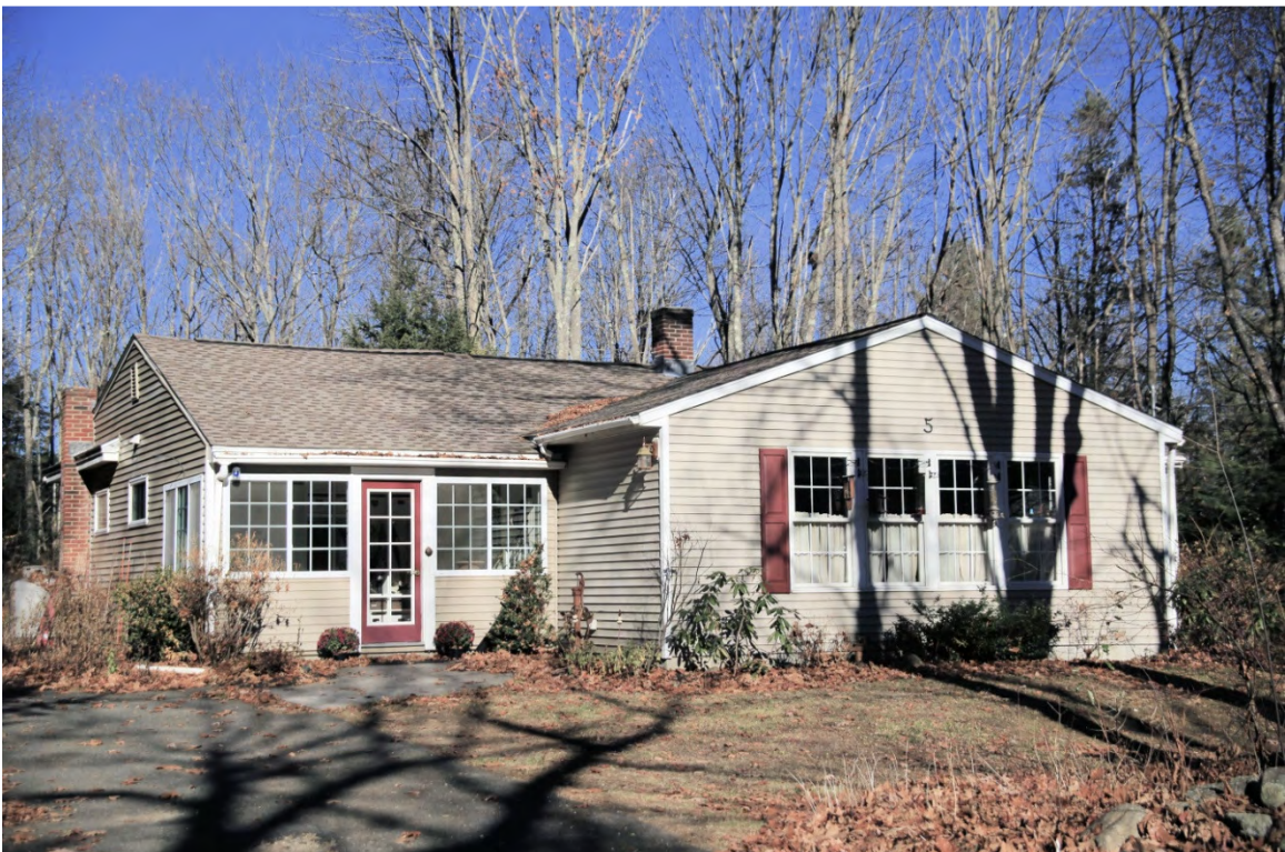
Photo 023) Pendexter Road Area – 5 Pendexter Road ID: D-06, photo taken November 2015
