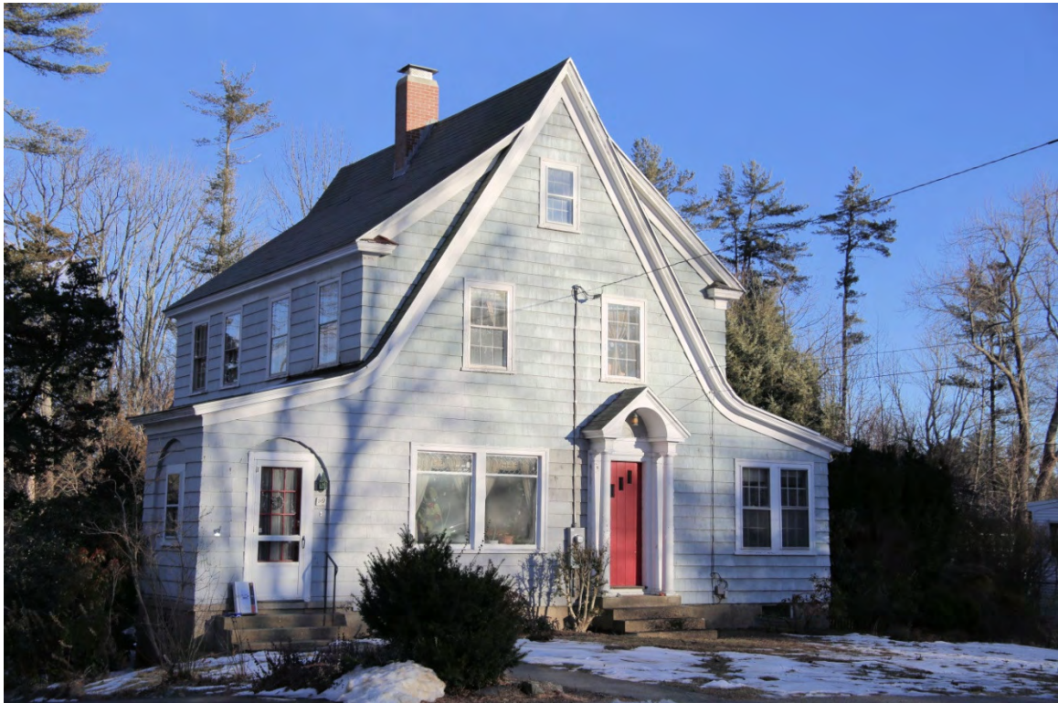
Photo 066) Madbury-Bagdad Road Area – Madbury Road ID: D-11, photo taken January 2016
