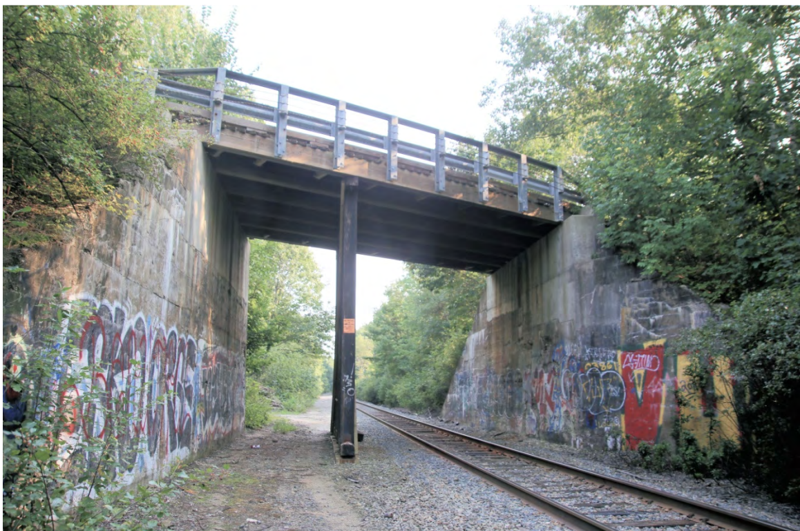
Photo 161) Bennett Road Railroad Bridge, B&M Railroad Western Division Historic District
