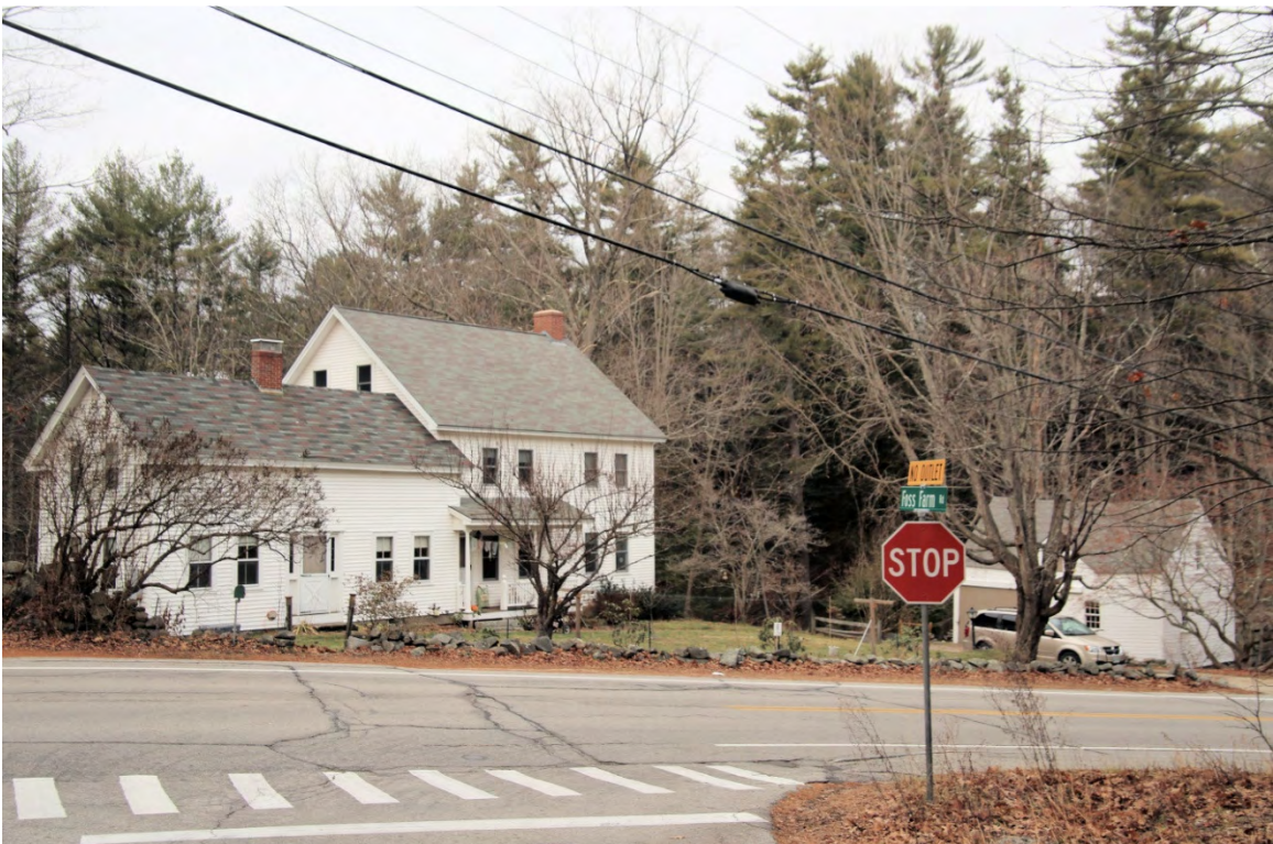
Photo 137) 74 Mill Road ID: D-29, photo taken December 2015
