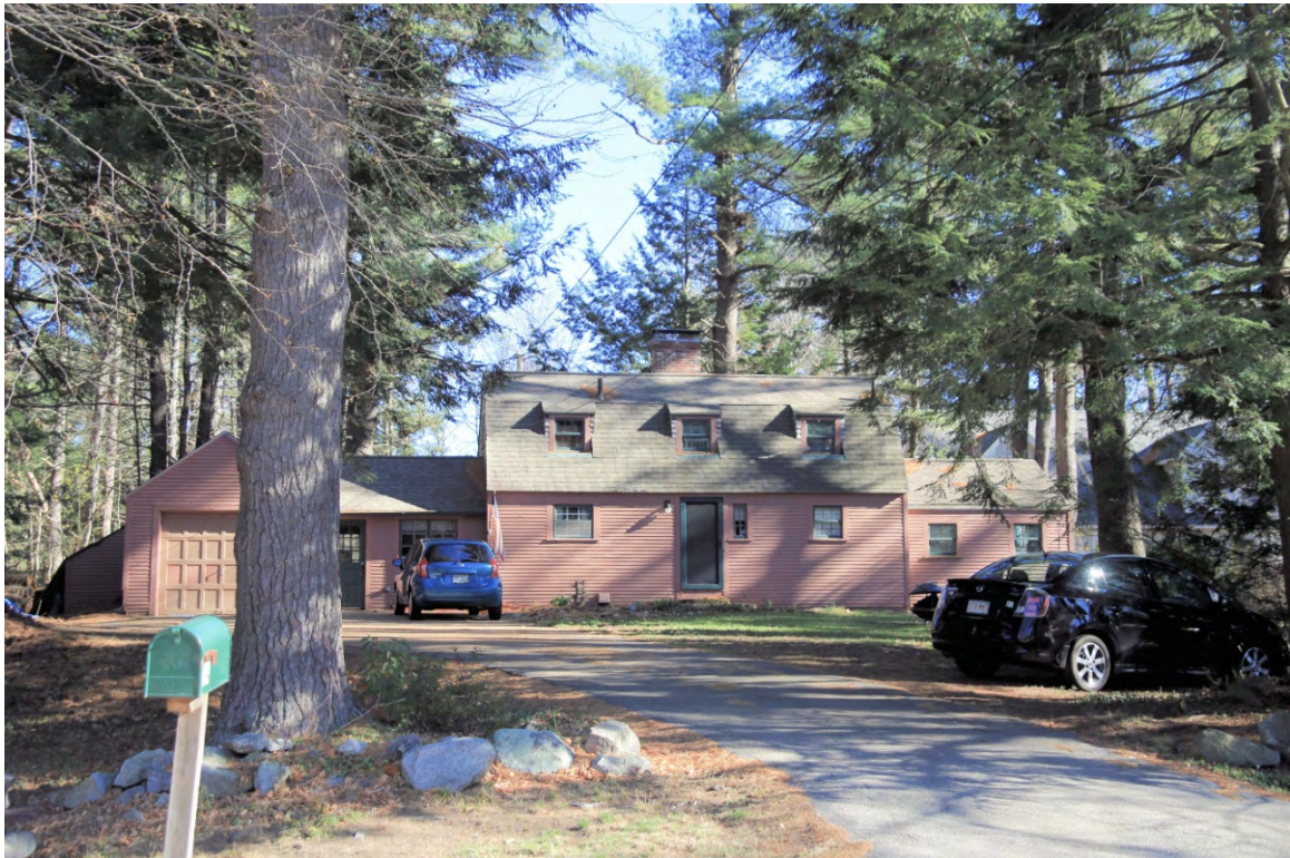
Photo 032) Madbury Road-Emerson Road Neighborhood – 114 Madbury Road ID: D-07, photo taken November 2015
