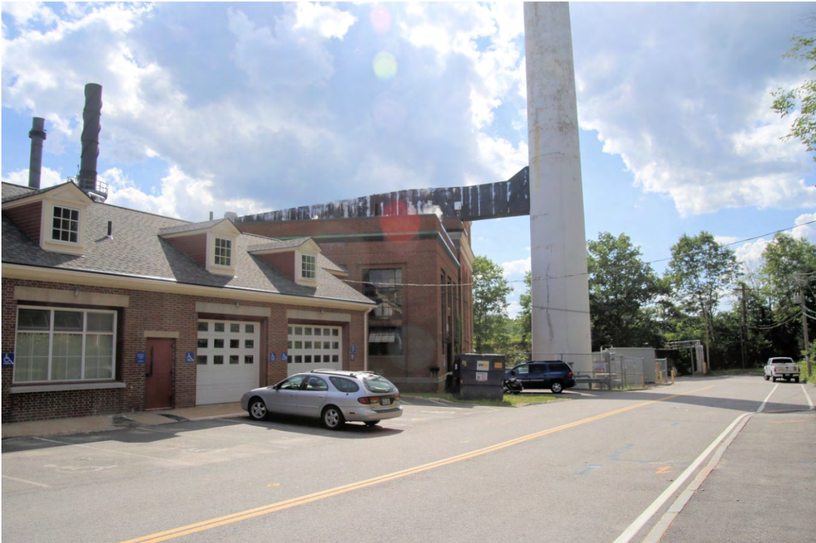
Photo 108) UNH – Library Way – Service Building and Heating Plant ID: D-21, photo taken June 2015
