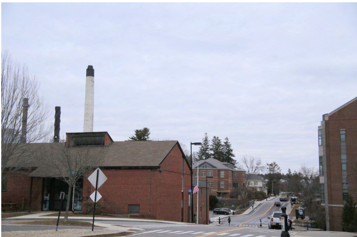
Photo 113) UNH – College Road – Zais Hall to left, Rudman right ID: D-21, photo taken December 2015
