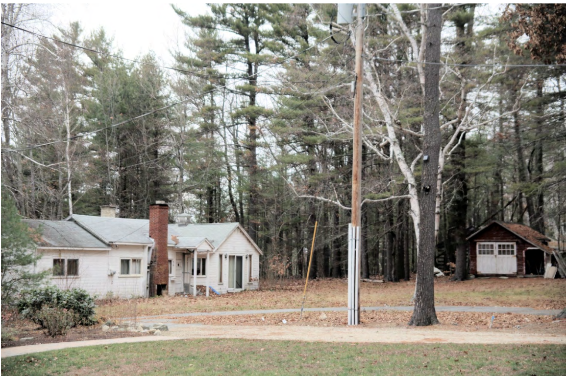
Photo 198) 76 Little Bay Road – Ira J. Witham Cottage (#84) Direction: W ID: N-02, photo taken December 2015
