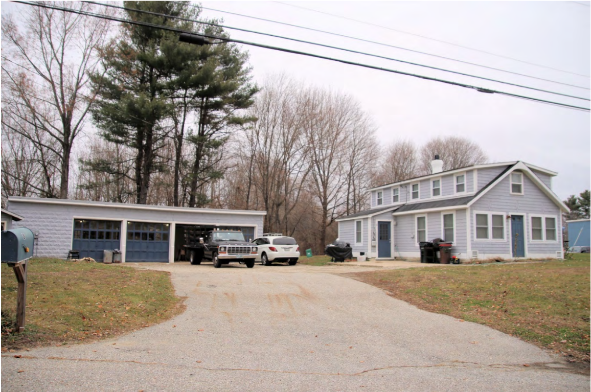
Photo 265) 436 Shattuck Way (NWN0172) Outside Project Area, photo taken December 2015
