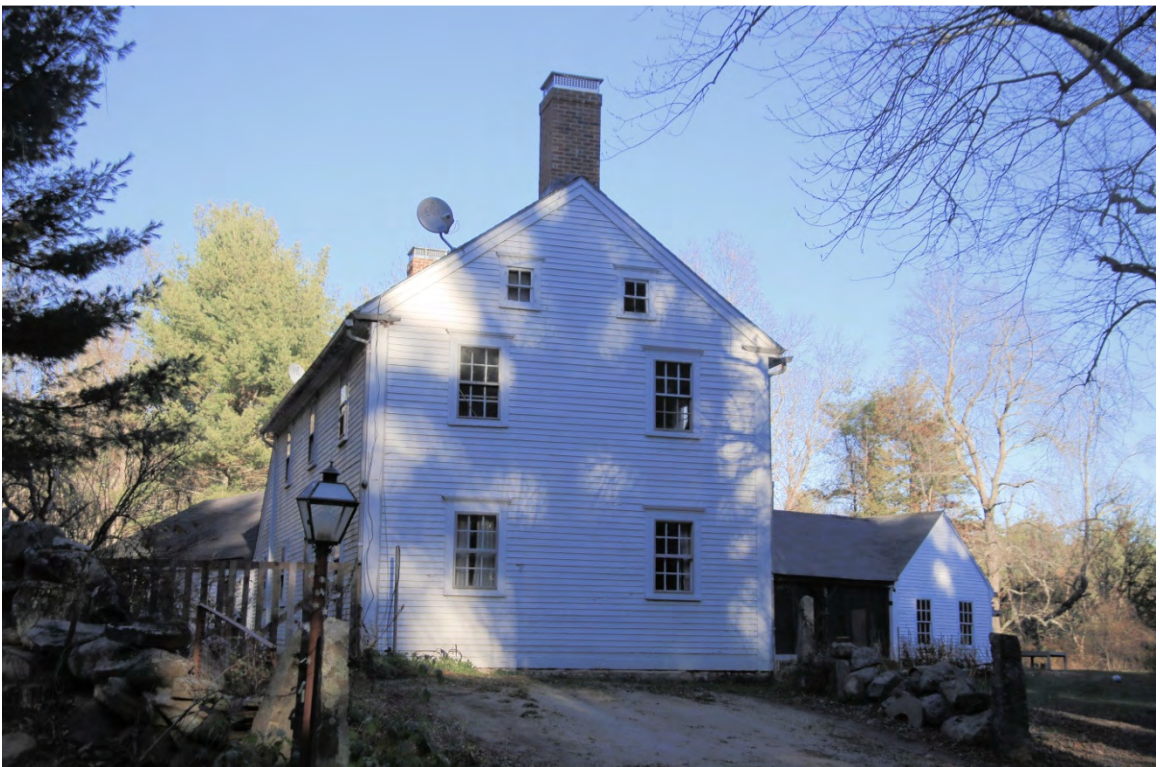
Photo 195) 345 Durham Point Road ID: D-70, photo taken November 2015
