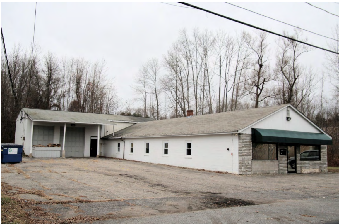
Photo 270) 34 Patterson Lane (#202) ID: N-65, photo taken December 2015
