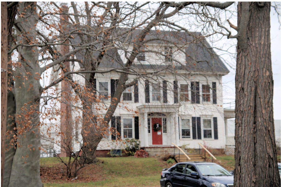
Photo 284) 2061 Woodbury Avenue – Great Bay Services, deRochemont House (#226)
