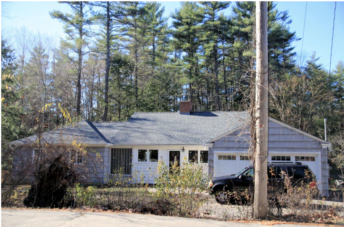
Photo 031) Madbury Road-Emerson Road Neighborhood – 115 Madbury Road ID: D-07, photo taken November 2015
