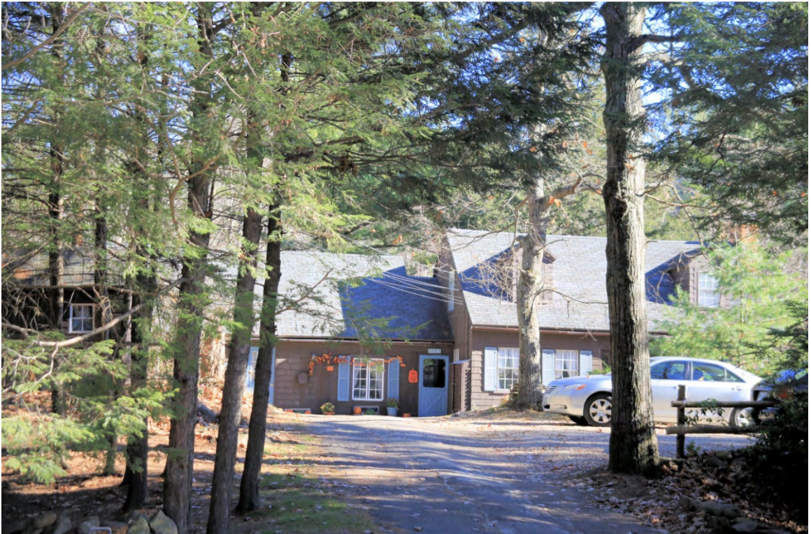
Photo 029) Madbury Road-Emerson Road Neighborhood – 124 Madbury Road ID: D-07, photo taken November 2015
