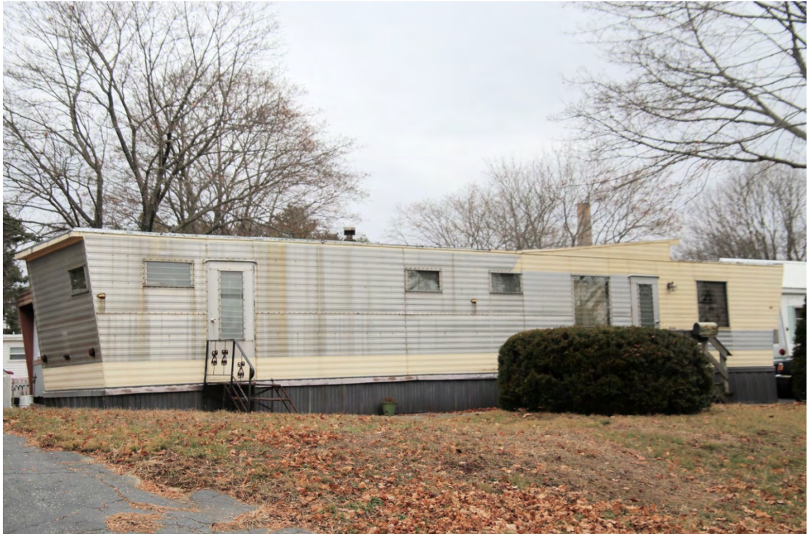
Photo 299) Oriental Gardens Area ID: P-05, photo taken December 2015
