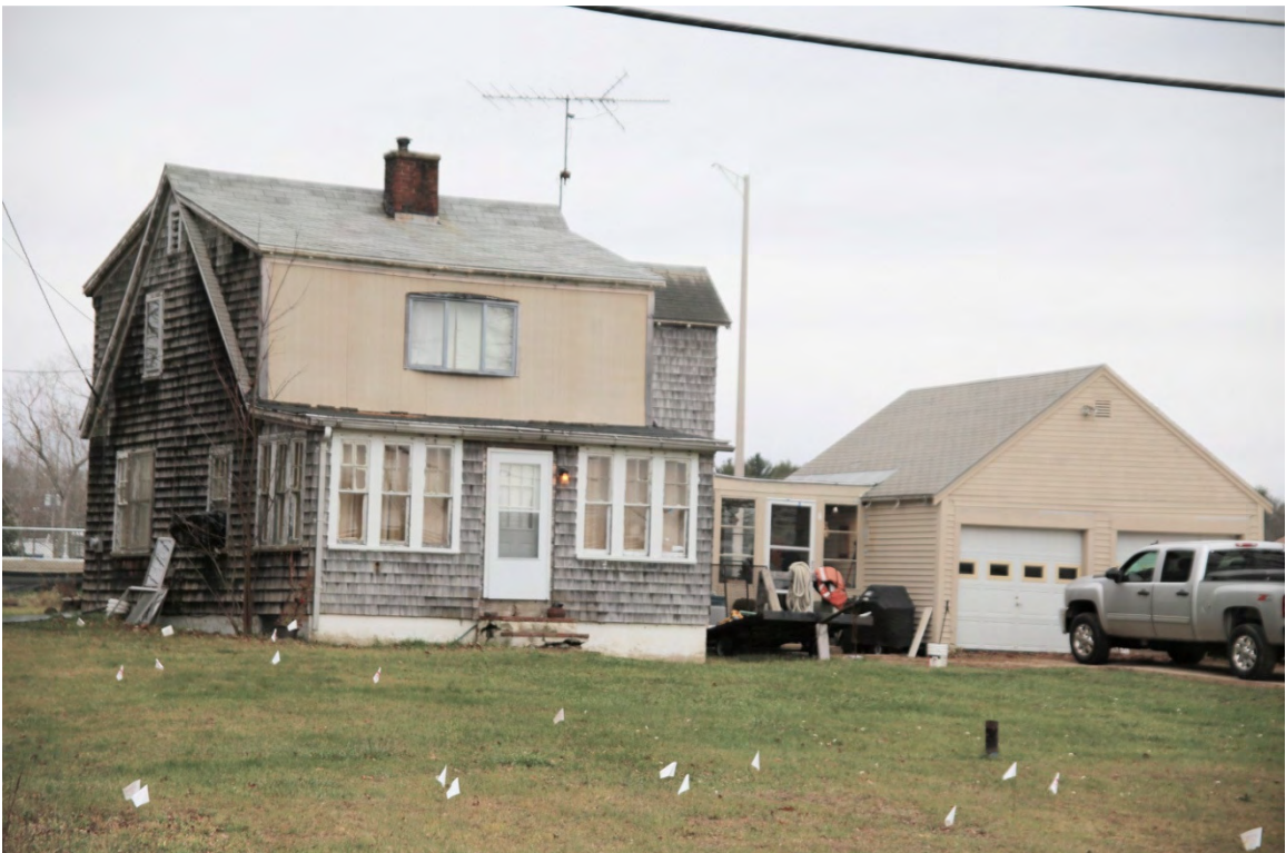
Photo 262) 399 Shattuck Way – Kershaw/Johnson House (NWN0177) Direction: W ID: N-57, photo taken December 2015
