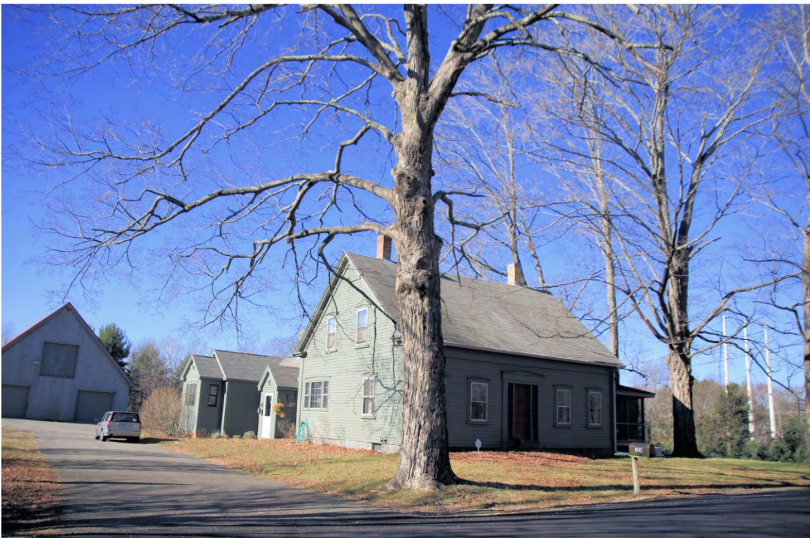
Photo 012) 124 Perkins Road ID: M-18, photo taken November 2015
