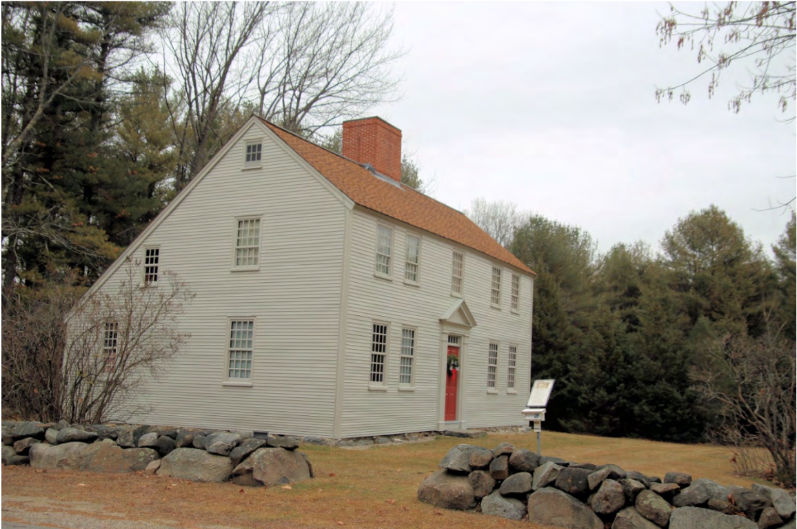
Photo 225) Newington Center Historic District – 337 Nimble Hill – Old Parsonage (#50)
