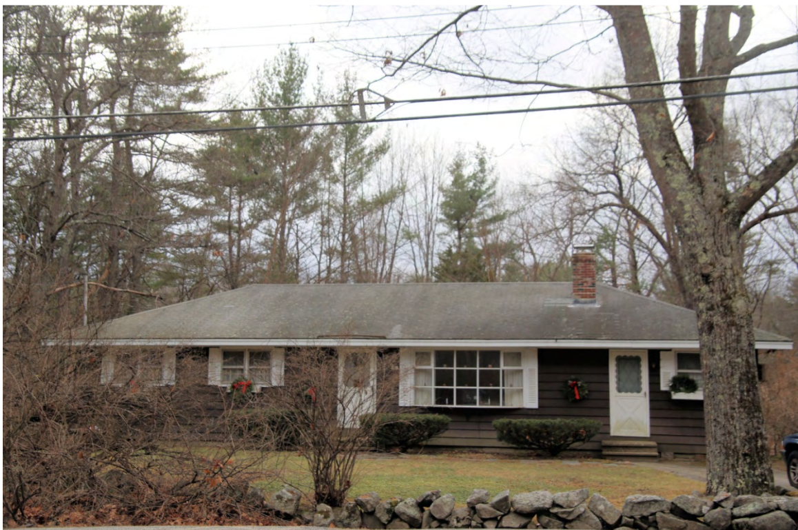
Photo 149) Mill Road/Woodridge Development – 87 Mill Road ID: D-32, photo taken December 2015
