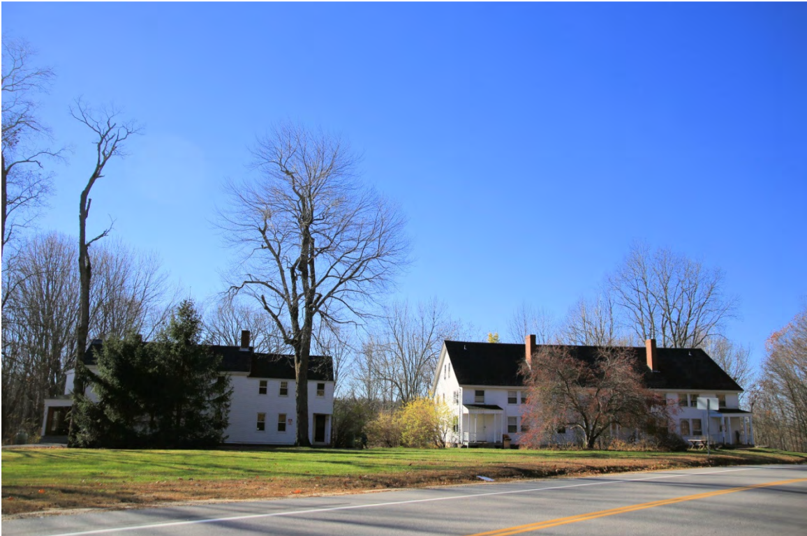
Photo 003) 10 Lee Road – Demerritt Homestead and apartments ID: M-02, photo taken November 2015
