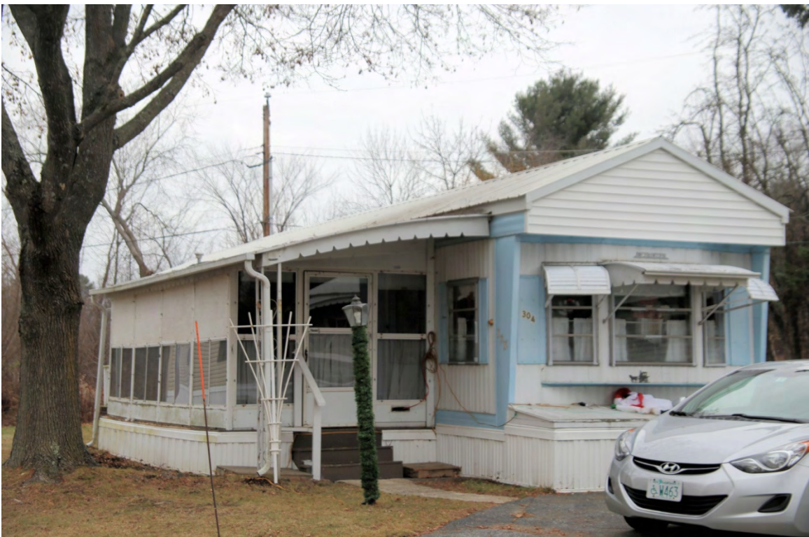
Photo 298) Oriental Gardens Area ID: P-05, photo taken December 2015
