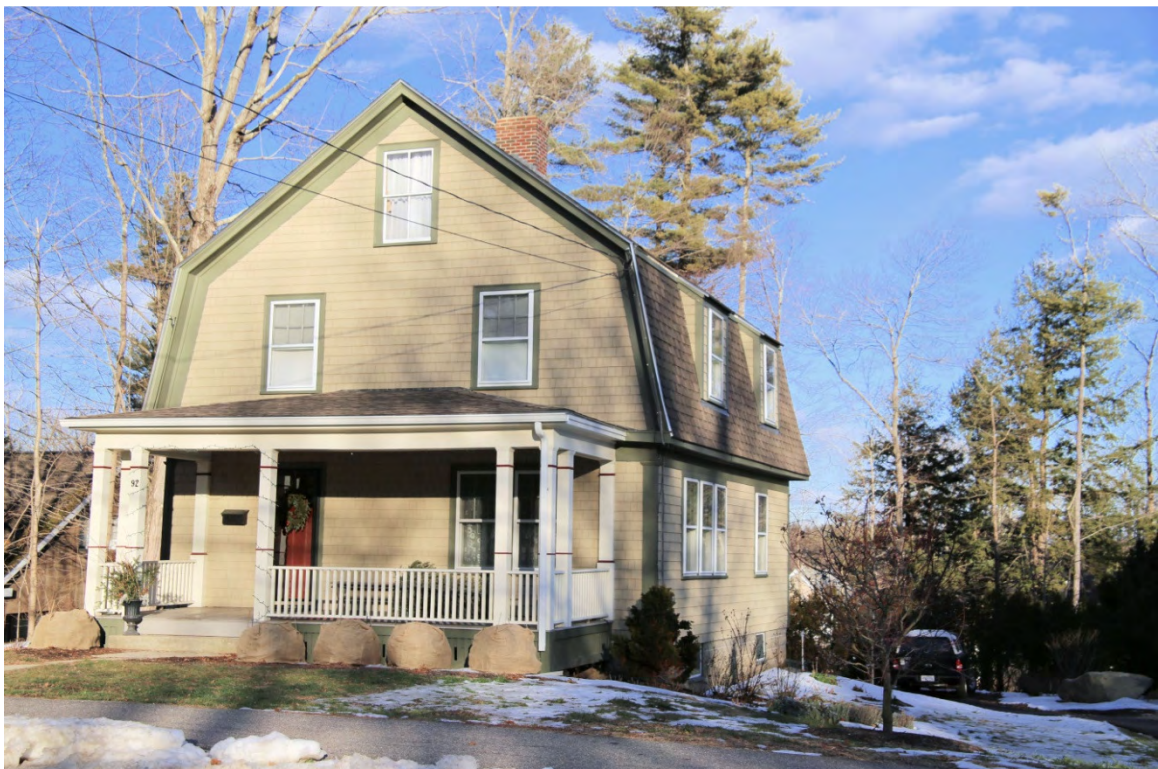
Photo 067) Madbury-Bagdad Road Area – Madbury Road ID: D-11, photo taken January 2016
