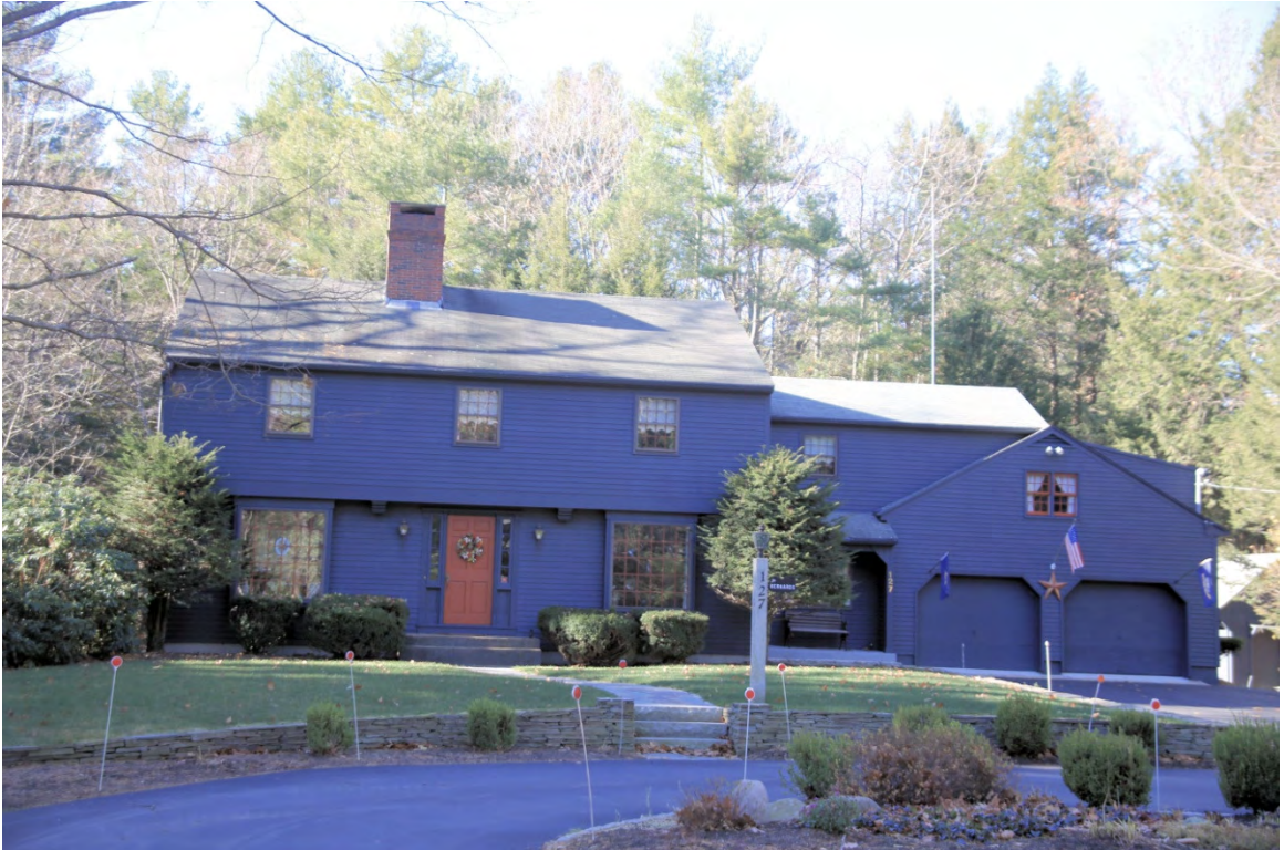
Photo 028) Madbury Road-Emerson Road Neighborhood – 127 Madbury Road ID: D-07, photo taken November 2015
