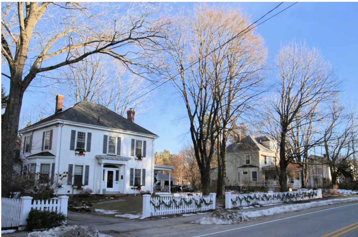
Photo 069) Madbury-Bagdad Road Area – Madbury Road ID: D-11, photo taken January 2016
