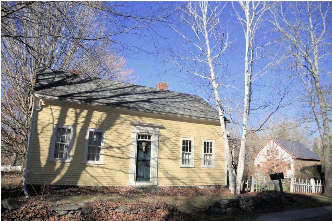
Photo 160) 62 Bennett Road ID: D-41, photo taken November 2015
