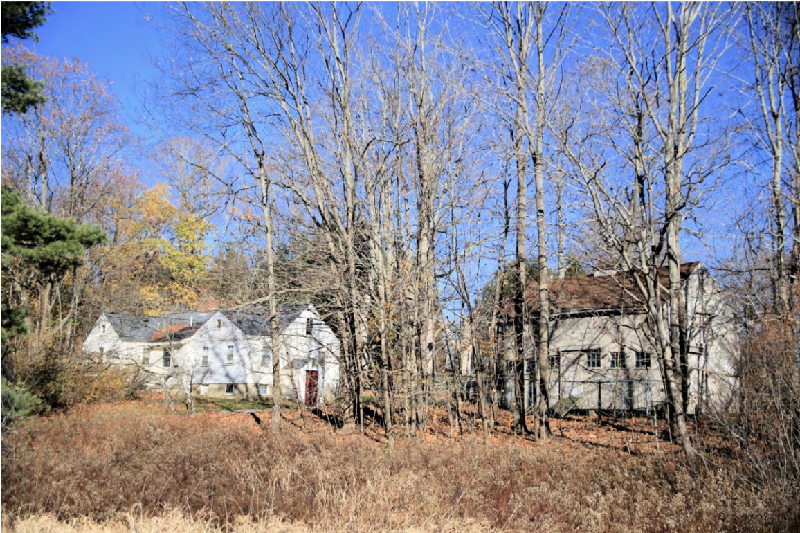
Photo 009) 171 Madbury Road ID: M-13, photo taken November 2015
