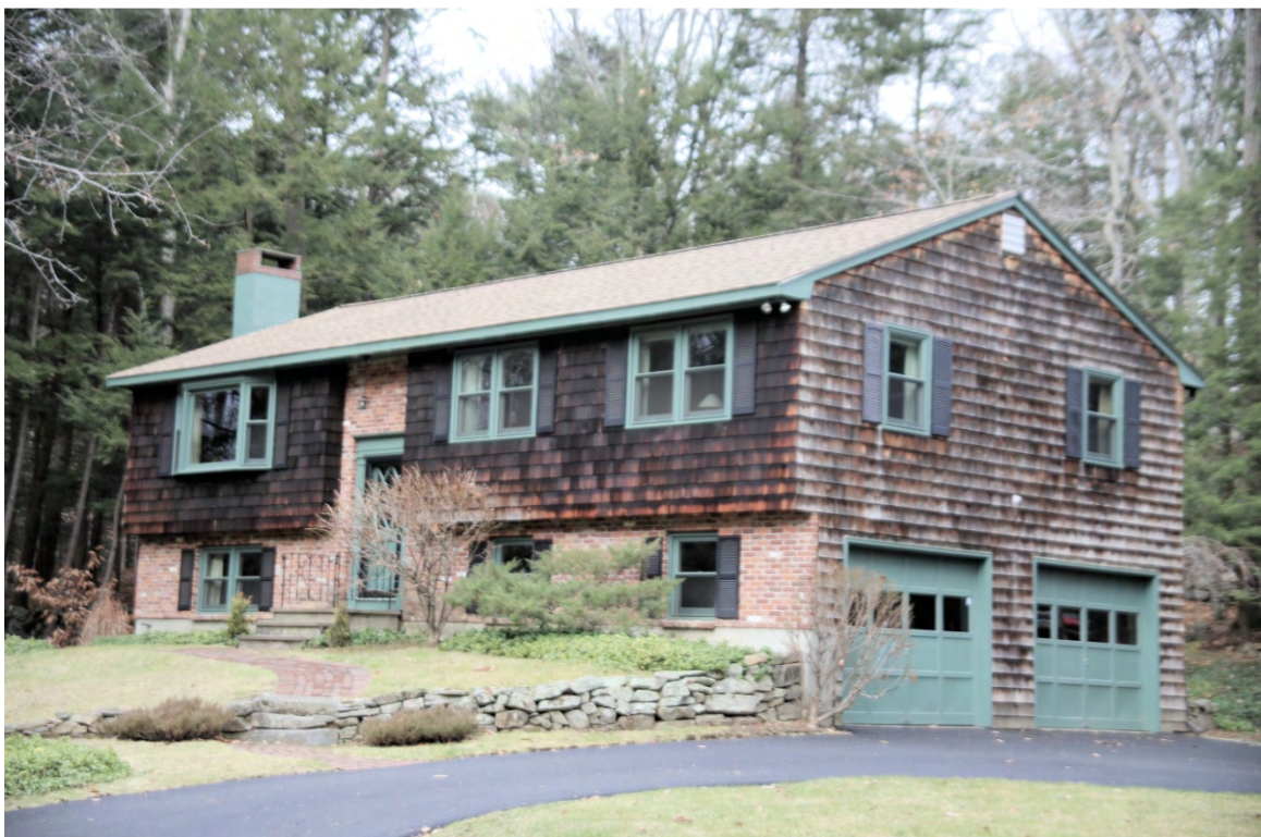
Photo 153) Mill Road/Woodridge Development – 33 Woodridge Road ID: D-32, photo taken December 2015
