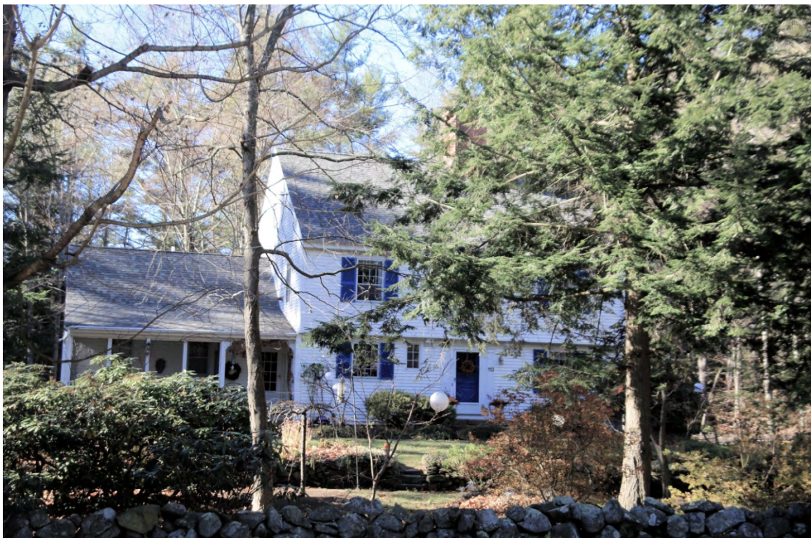
Photo 033) Madbury Road-Emerson Road Neighborhood – 113 Madbury Road ID: D-07, photo taken November 2015
