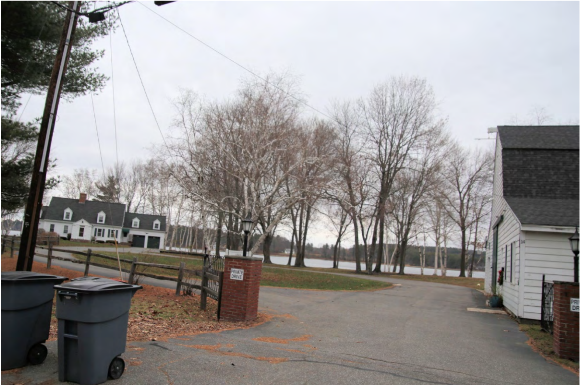
Photo 261) 22 Bloody Point Road – Holden House/Alex Johnson Conference Center (#169, part of Area NWN-Sprague) Direction: N Outside Project Area, photo taken December 2015
