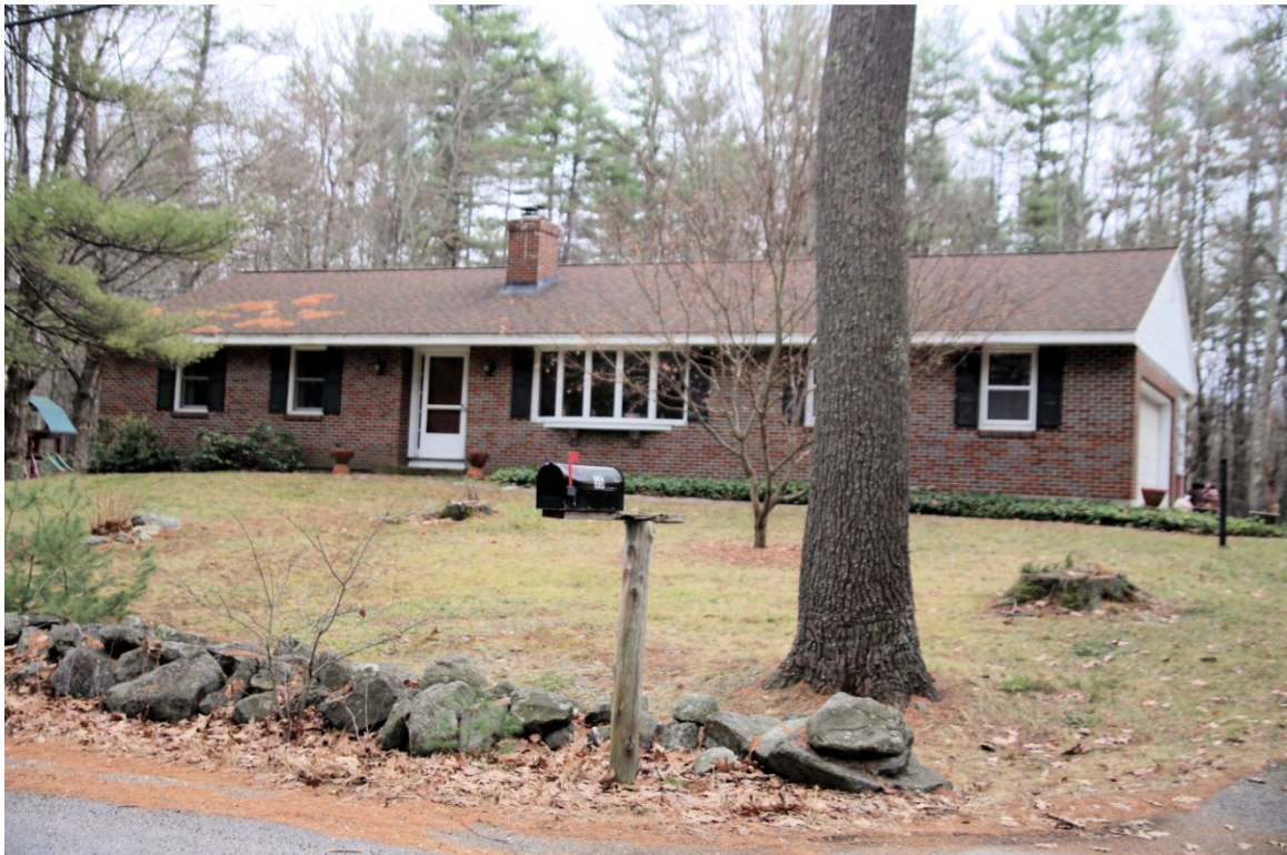
Photo 156) Mill Road/Woodridge Development – 95 Mill Road ID: D-32, photo taken December 2015
