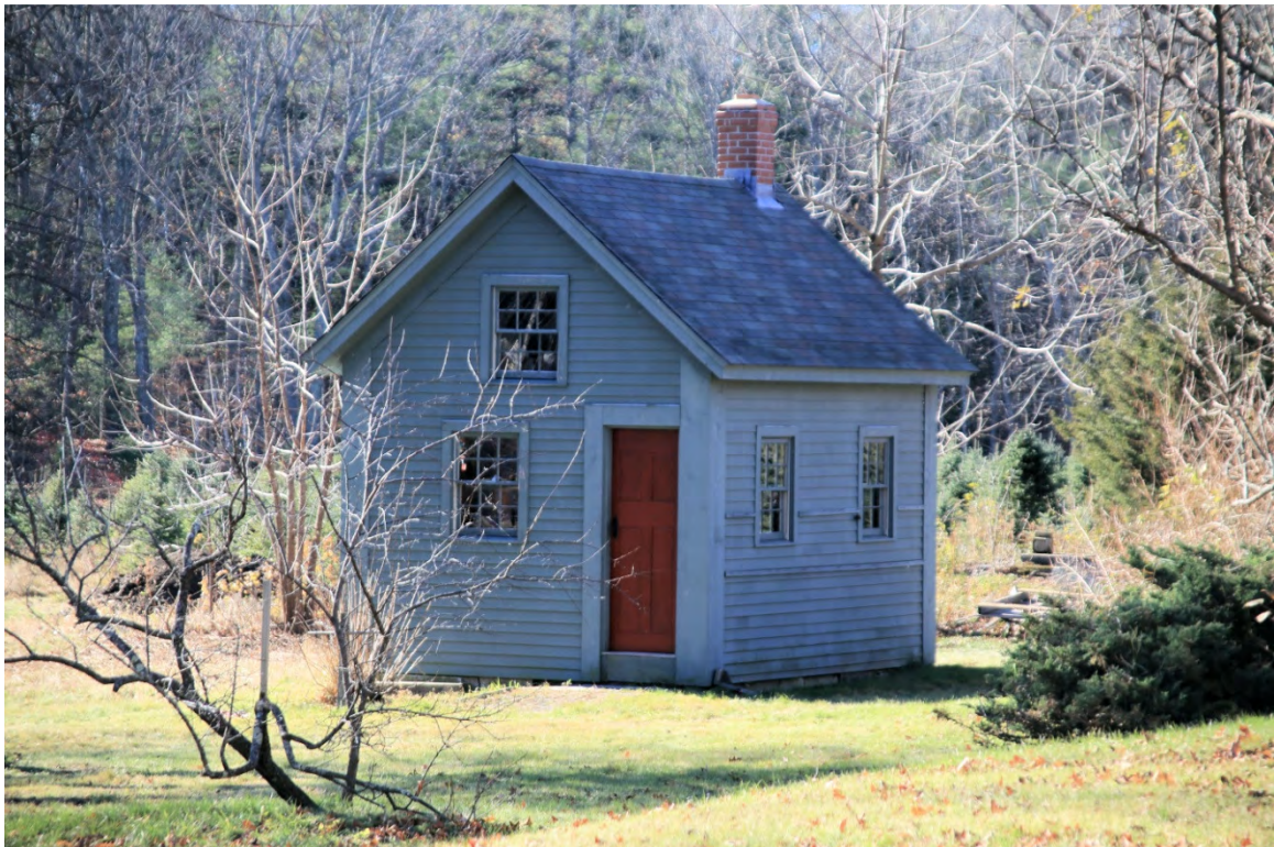
Photo 013) 124 Perkins Road outbuilding ID: M-18, photo taken November 2015
