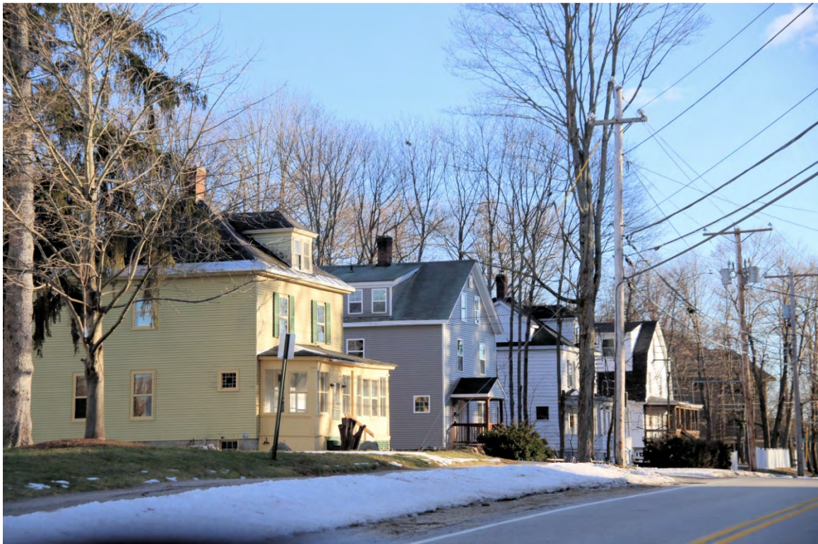
Photo 070) Madbury-Bagdad Road Area – Madbury Road ID: D-11, photo taken January 2016
