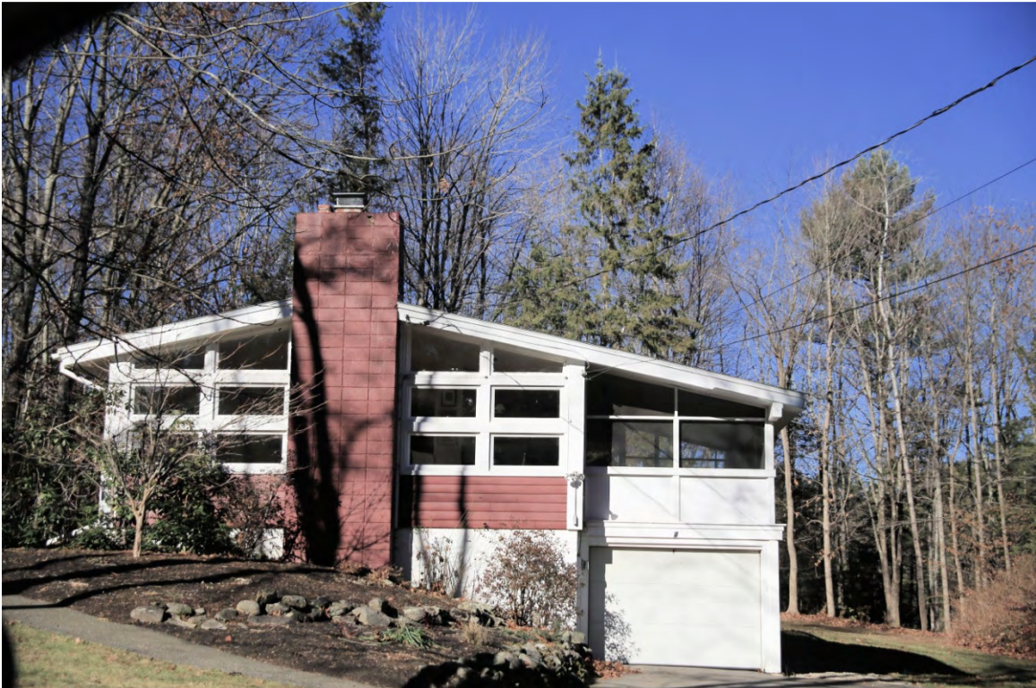
Photo 022) Pendexter Road Area – 7 Pendexter Road ID: D-06, photo taken November 2015
