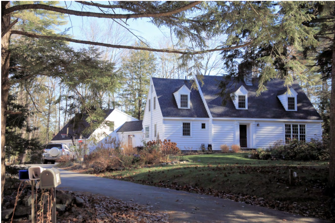
Photo 036) Madbury Road-Emerson Road Neighborhood – 102 Madbury Road ID: D-07, photo taken November 2015
