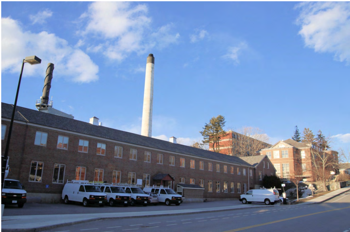
Photo 112) UNH – College Road – Service Building ID: D-21, photo taken January 2016
