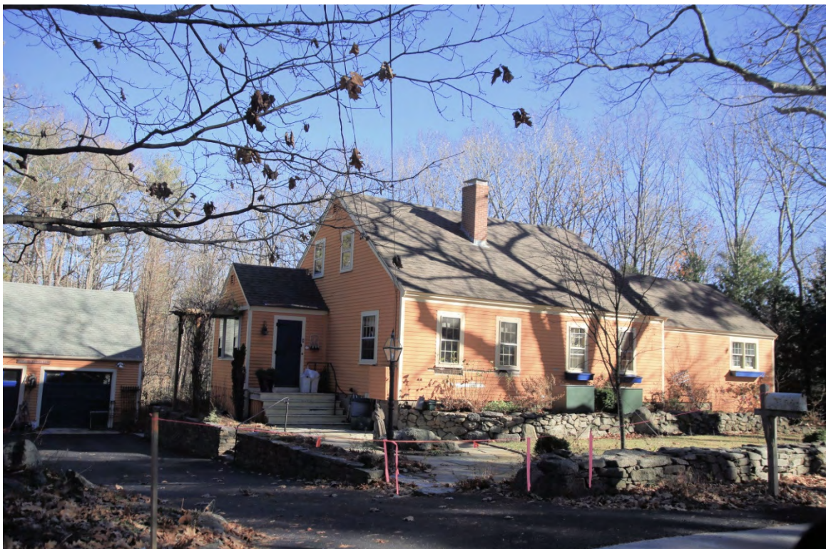
Photo 049) Madbury Road-Emerson Road Neighborhood – 5 Emerson Road ID: D-07, photo taken November 2015
