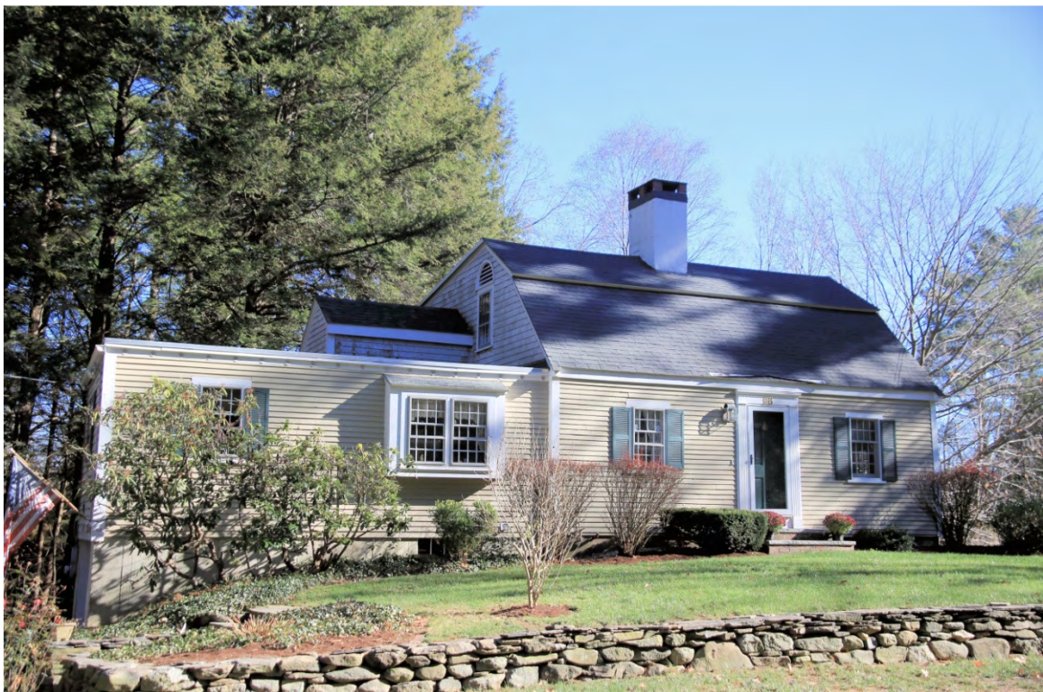
Photo 037) Madbury Road-Emerson Road Neighborhood – 98 Madbury Road ID: D-07, photo taken November 2015
