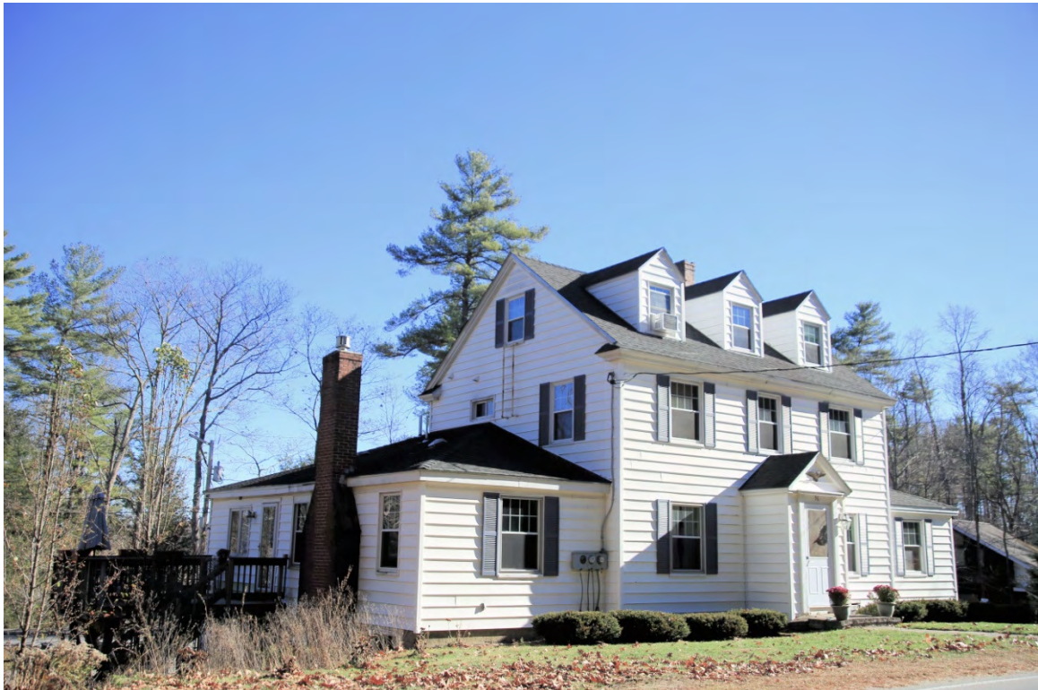
Photo 038) Madbury Road-Emerson Road Neighborhood – 96 Madbury Road ID: D-07, photo taken November 2015
