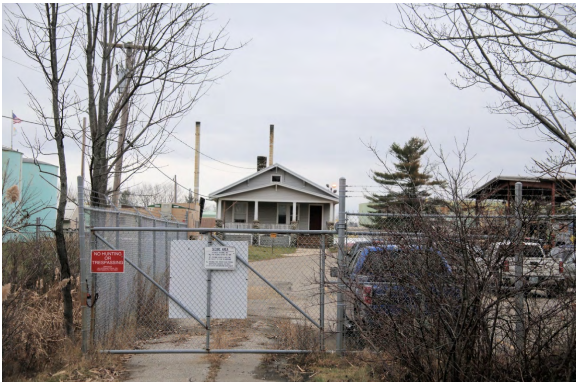
Photo 264) 372 Shattuck Way – Sprague Energy Plant (#178, Area NWN-SP) ID: N-58, photo taken December 2015
