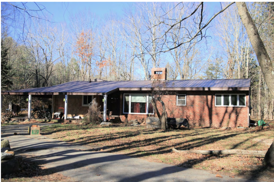
Photo 025) Pendexter Road Area – 1 Pendexter Road ID: D-06, photo taken November 2015
