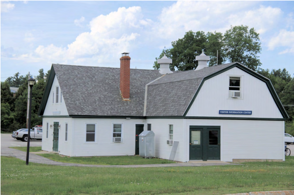
Photo 080) Mast Road Extension – UNH Transit and Visitor Center ID: D-17, photo taken June 2015
