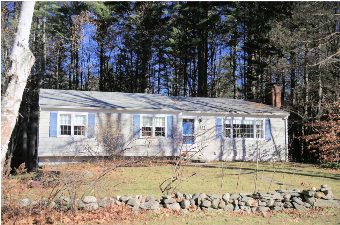
Photo 051) Madbury Road-Emerson Road Neighborhood – 17 Emerson Road ID: D-07, photo taken November 2015
