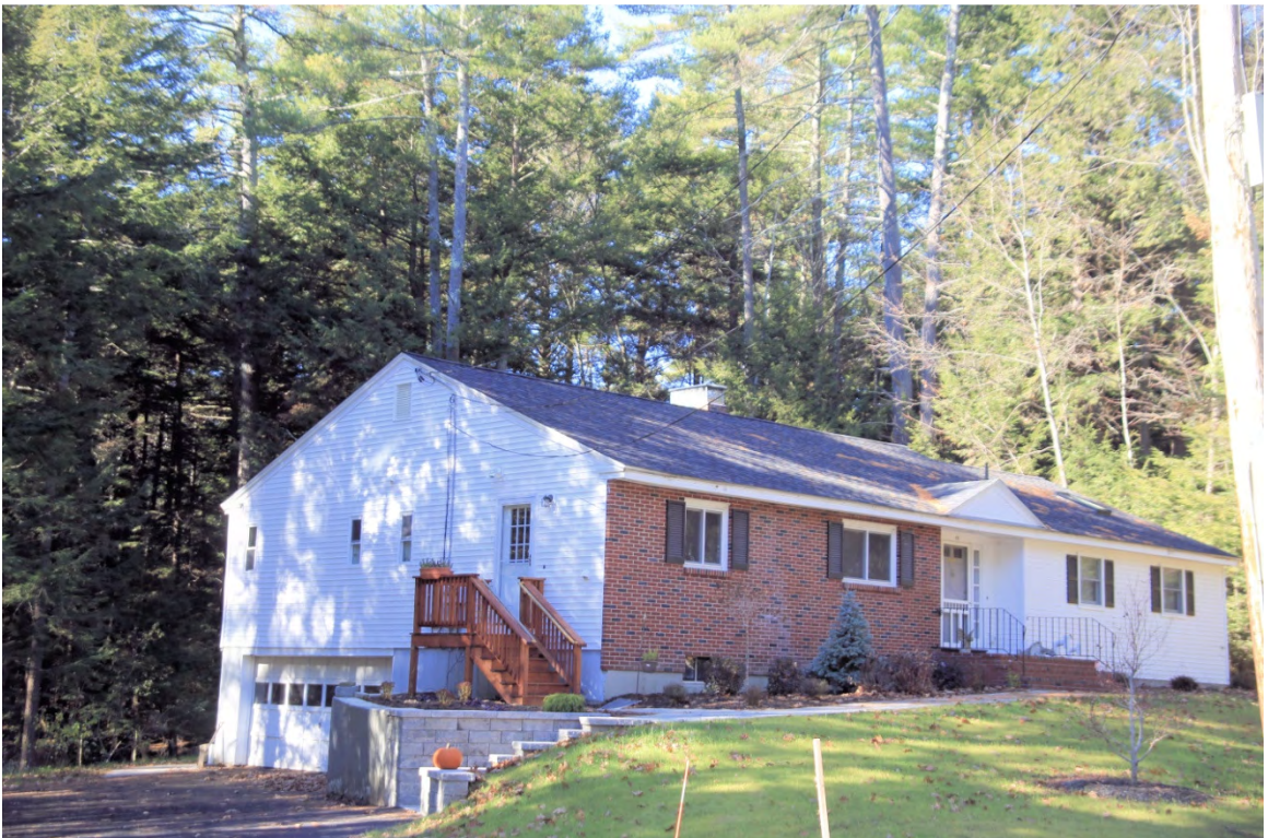
Photo 035) Madbury Road-Emerson Road Neighborhood – 108 Madbury Road ID: D-07, photo taken November 2015
