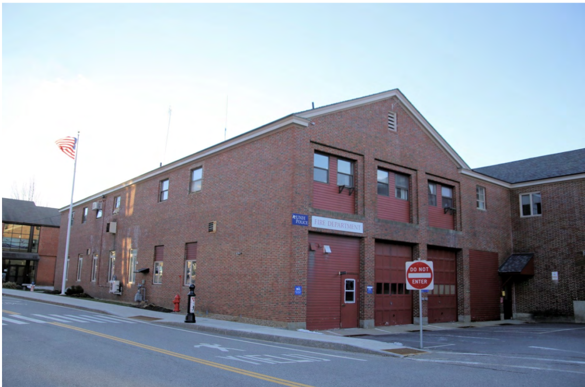
Photo 111) UNH – College Road – Service Building ID: D-21, photo taken January 2016
