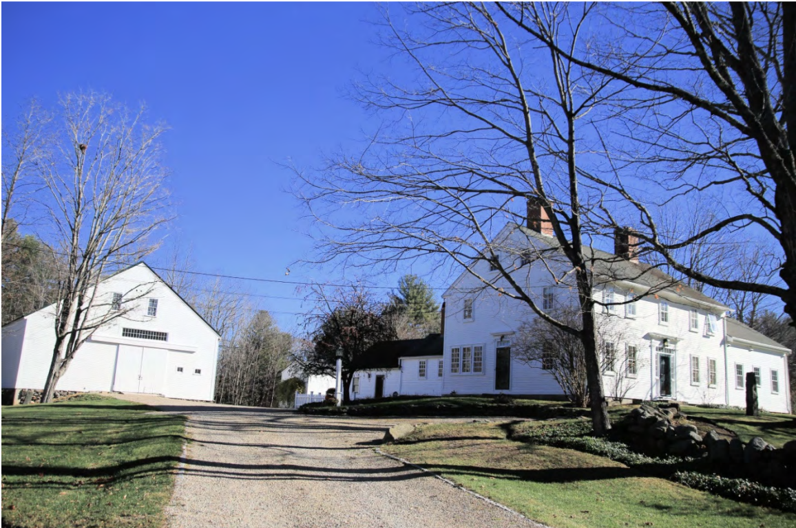
Photo 017) 12 Pendexter Road ID: M-21, photo taken November 2015
