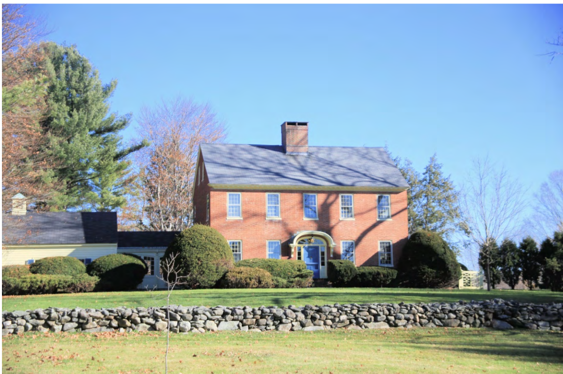
Photo 008) 173 Madbury Road (MAD0047) ID: M-12, photo taken November 2015
