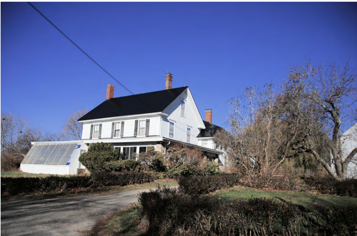
Photo 014) 105 Perkins Road – Roselawn Farm ID: M-19, photo taken November 2015
