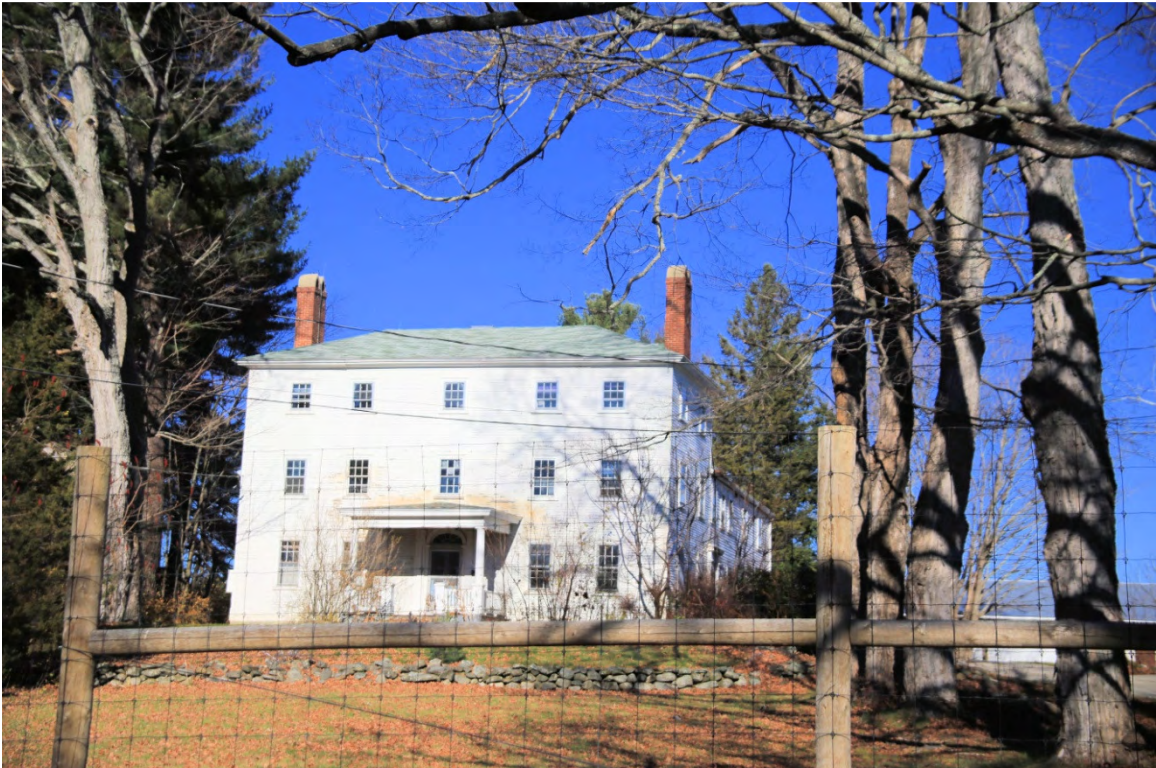
Photo 005) 333 Knox Marsh Road – UNH Kingman Farm, (#51, MAD0051) Outside Project Area, photo date November 2015
