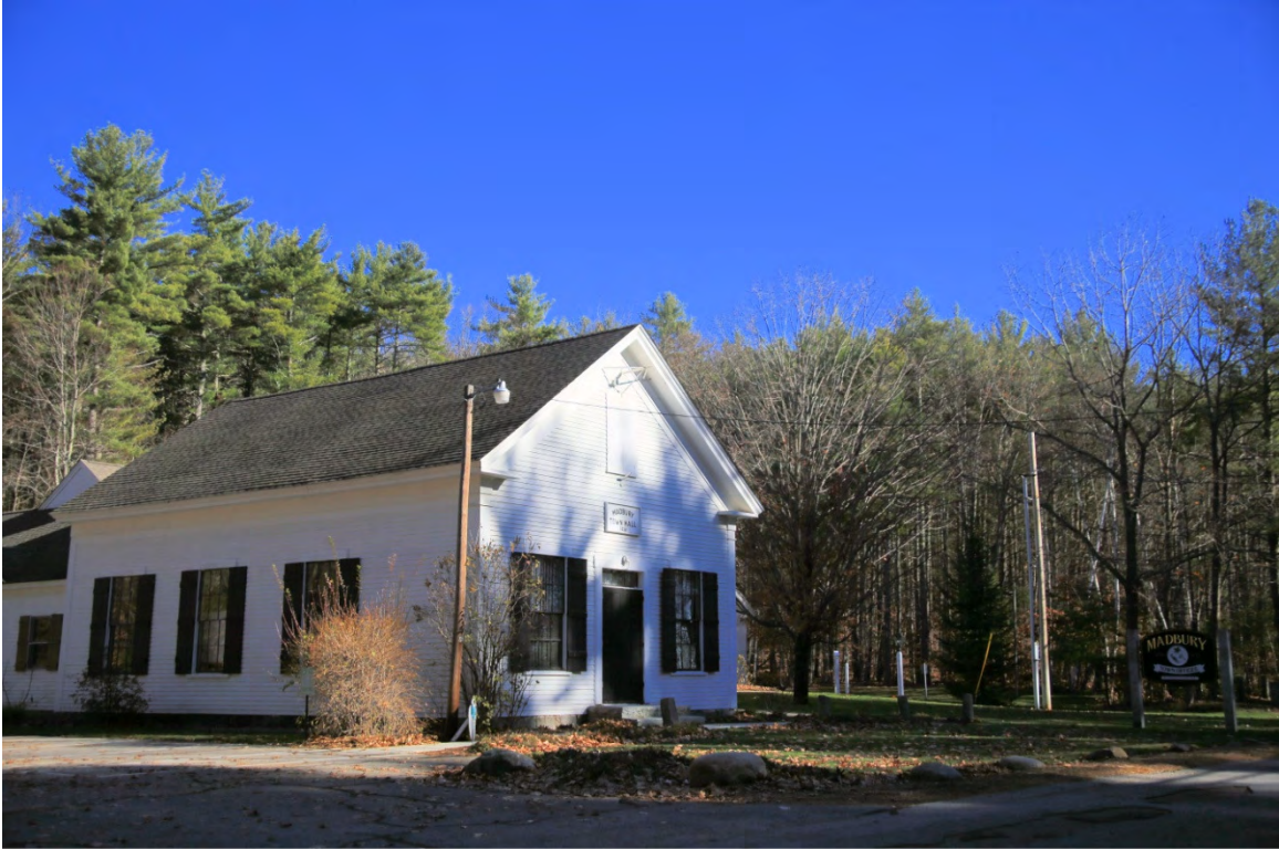
Photo 001) 13 Town Hall Road – Madbury Town Hall ID: M-01, photo taken November 2015
