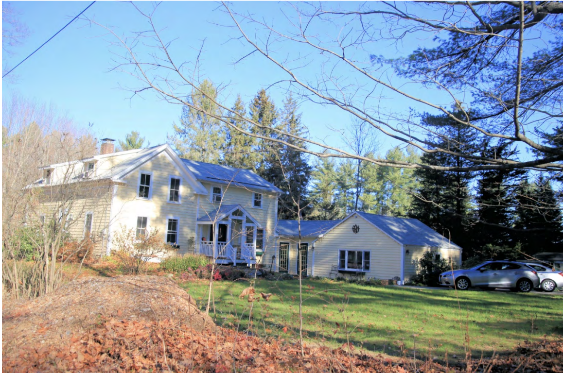
Photo 020) 8 Beech Hill Road ID: D-02, photo taken November 2015
