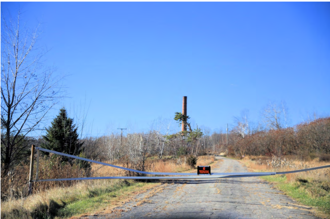
Photo 004) off Nicco Road – Elliott Greenhouses boiler stack (MAD0050) ID: M-04, photo taken November 2015
