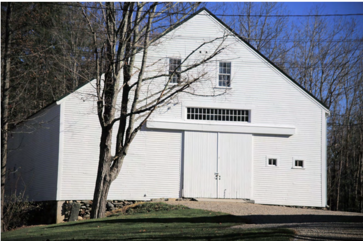
Photo 018) 12 Pendexter Road ID: M-21, photo taken November 2015
