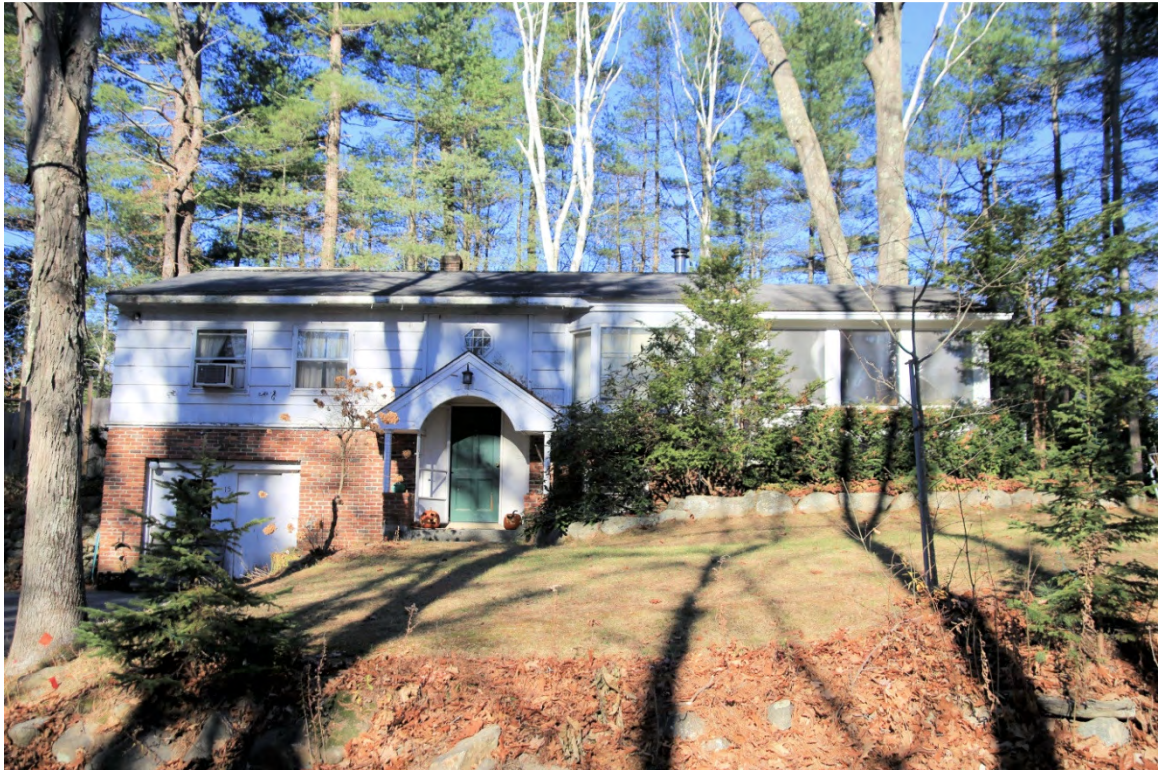
Photo 019) 15 Pendexter Road ID: M-22, photo taken November 2015
