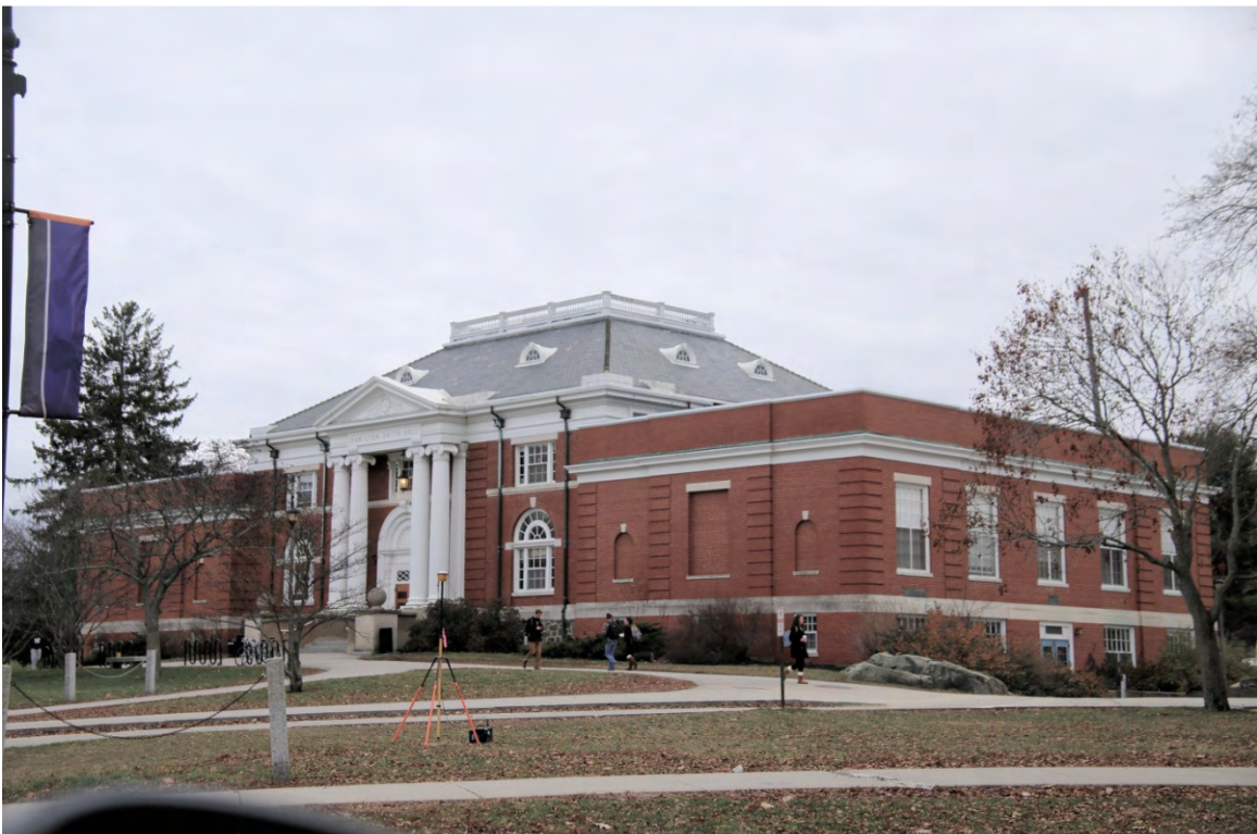
Photo 105) UNH – Main Street – Hamilton Smith Hall ID: D-21, photo taken December 2015
