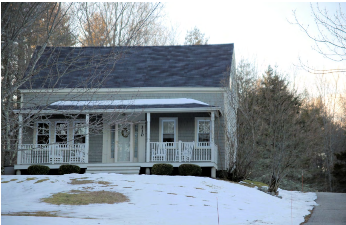
Photo 167) Newmarket-Bennett Road Farms Historic District – 110 Newmarket Road (DUR0012)
