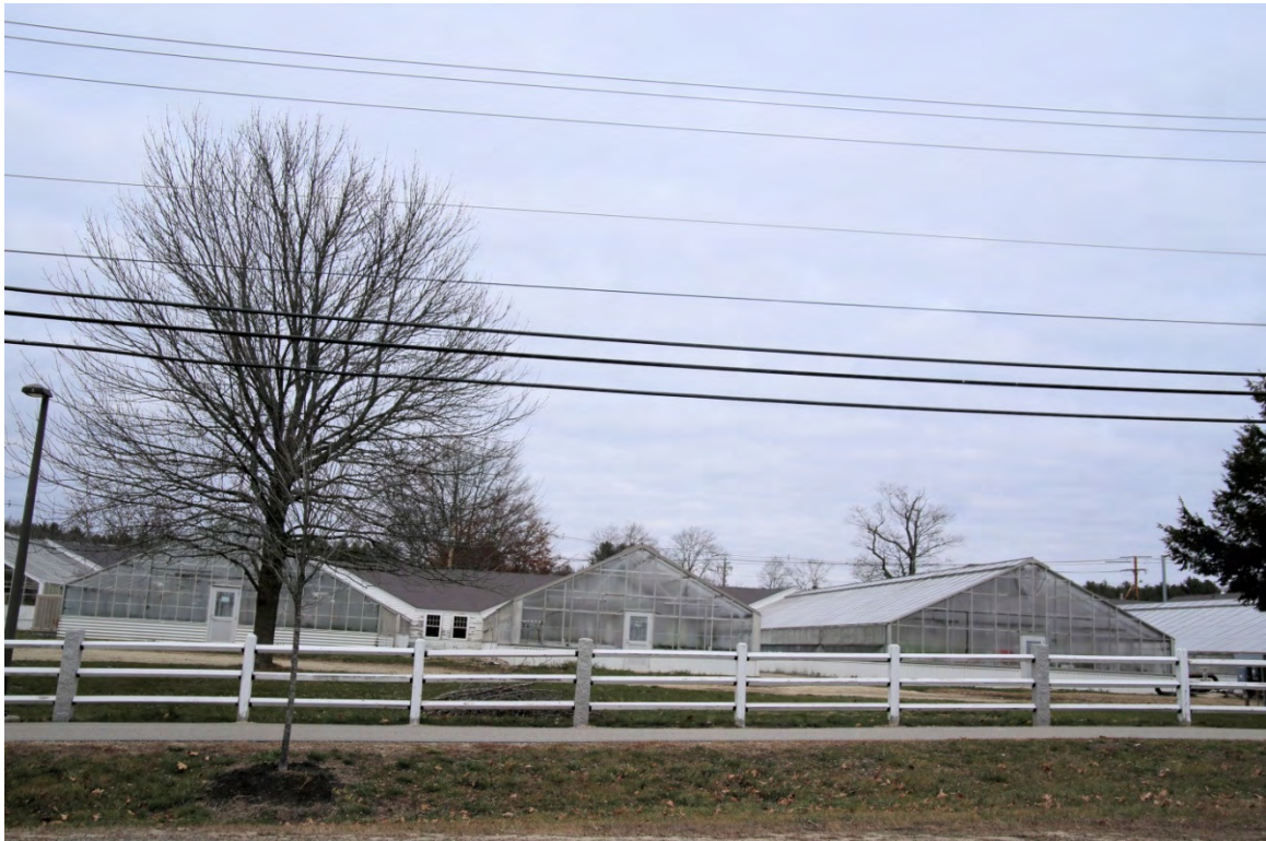
Photo 084) UNH Thompson School – Greenhouses from Main Street ID: D-17, photo taken December 2015
