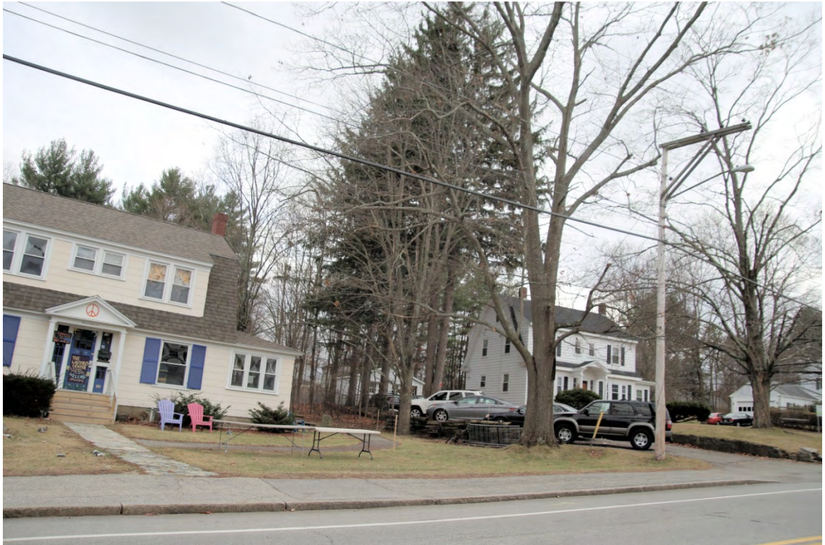
Photo 128) Mill Road Historic Area – 15 and 17 Mill Road ID: D-27, photo taken December 2015
