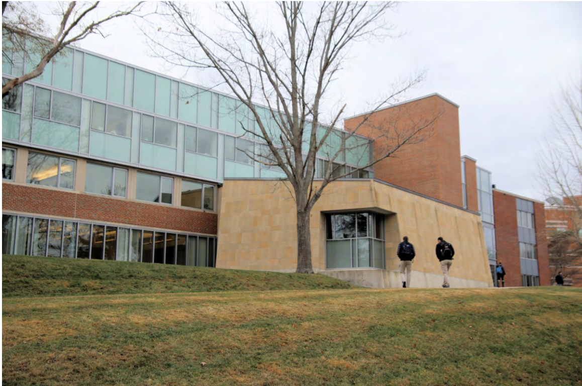
Photo 118) UNH – Academic Way – Kingsbury Hall ID: D-21, photo taken December 2015
