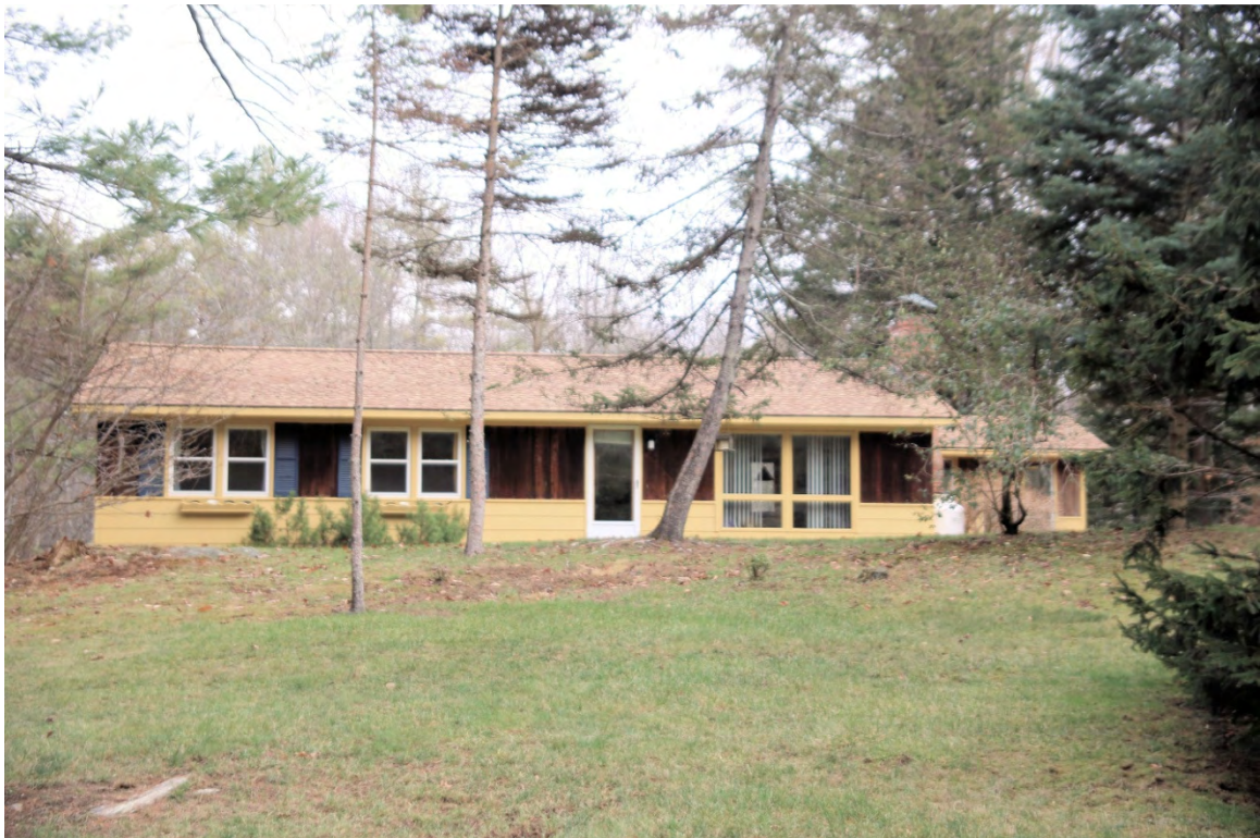
Photo 152) Mill Road/Woodridge Development – 44 Woodridge Road ID: D-32, photo taken December 2015
