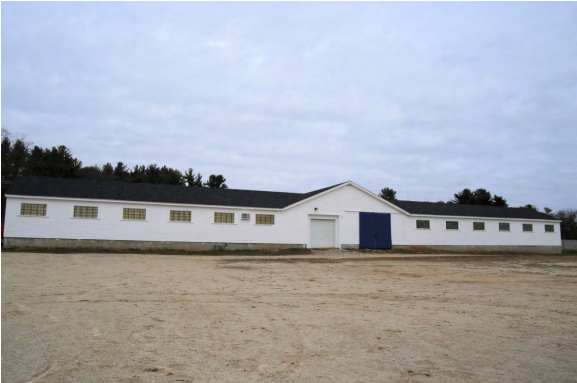
Photo 086) UNH Thompson School – Smith Equine Center from Main Street ID: D-17, photo taken June 2015
