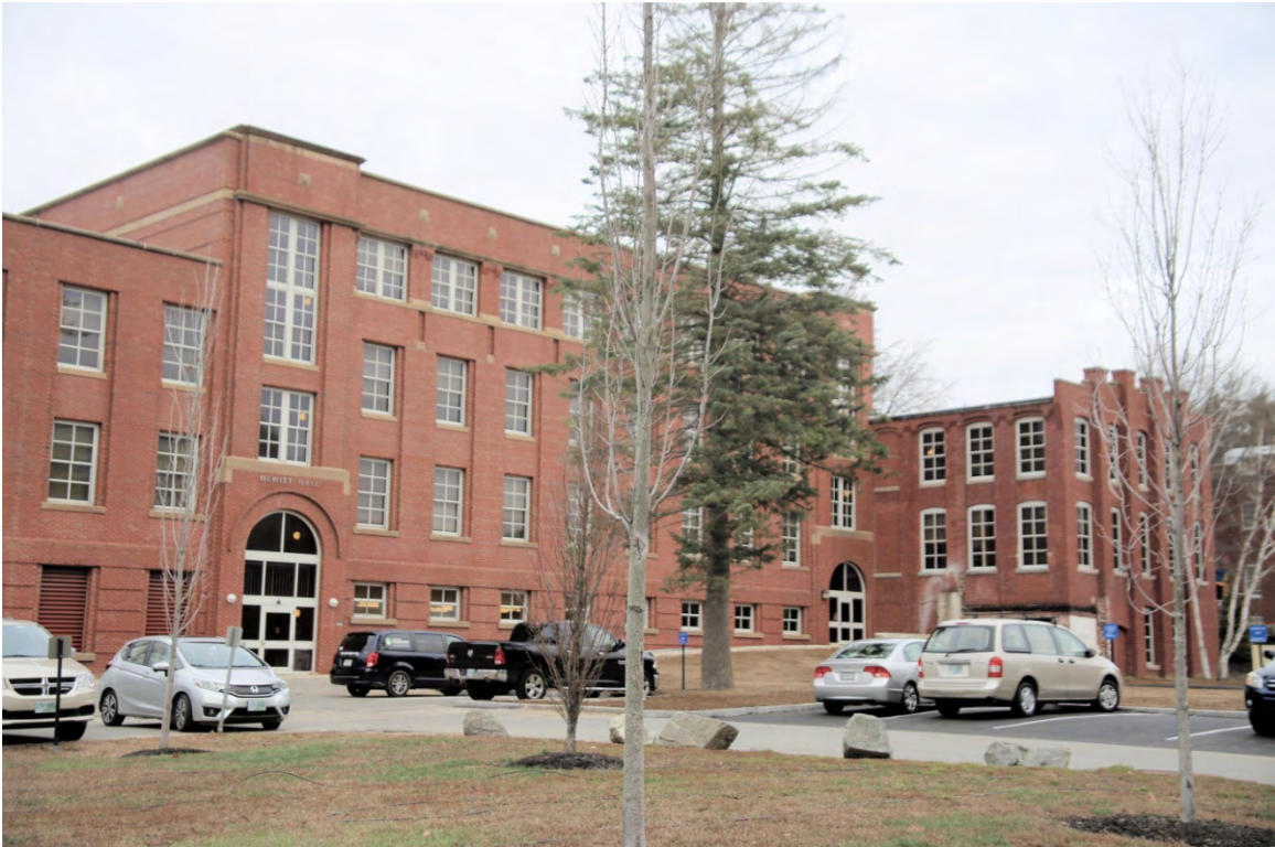
Photo 114) UNH – College Road – Hewitt Hall ID: D-21, photo taken December 2015
