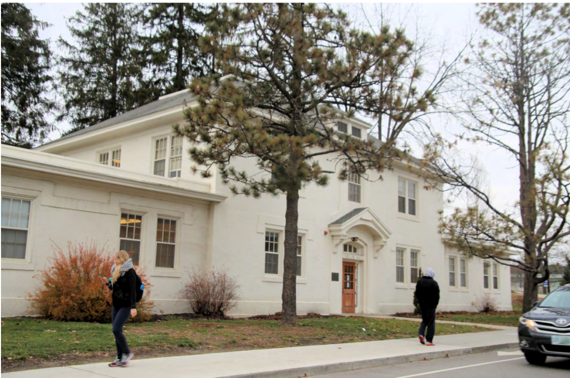
Photo 107) UNH – College Road – Taylor Hall ID: D-21, photo taken December 2015
