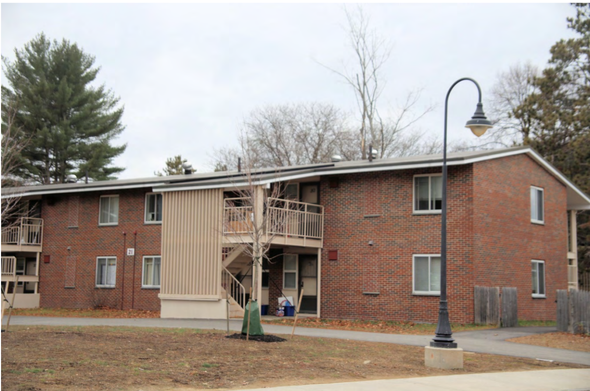
Photo 117) UNH – McDaniel Drive – Forest Park Apartments ID: D-21, photo taken December 2015
