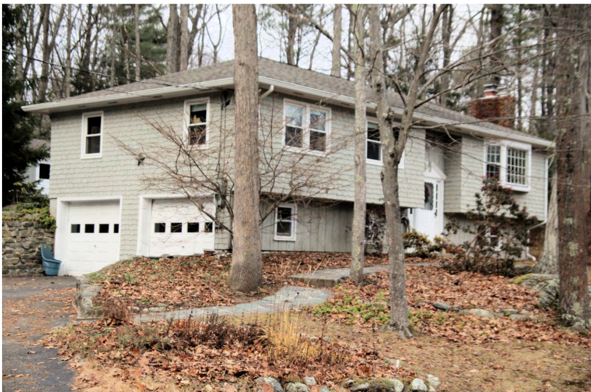
Photo 151) Mill Road/Woodridge Development – 2 Woodridge Road ID: D-32, photo taken December 2015
