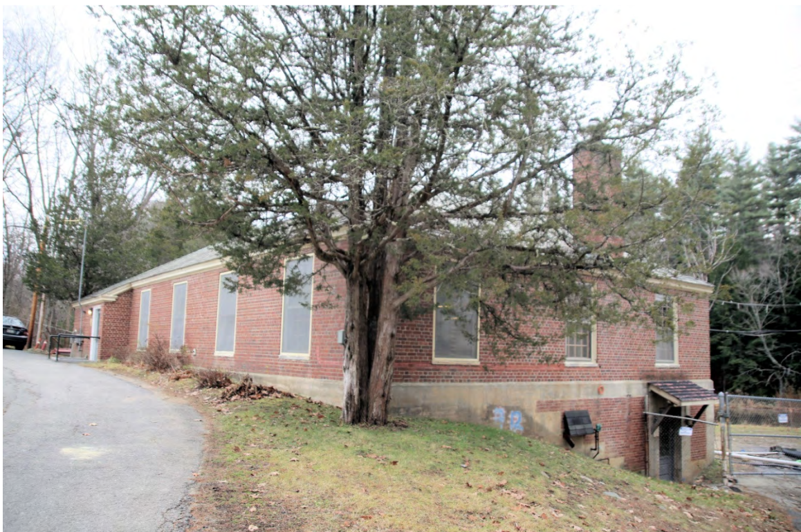
Photo 125) Waterworks Road – Waterworks ID: D-25, photo taken December 2015
