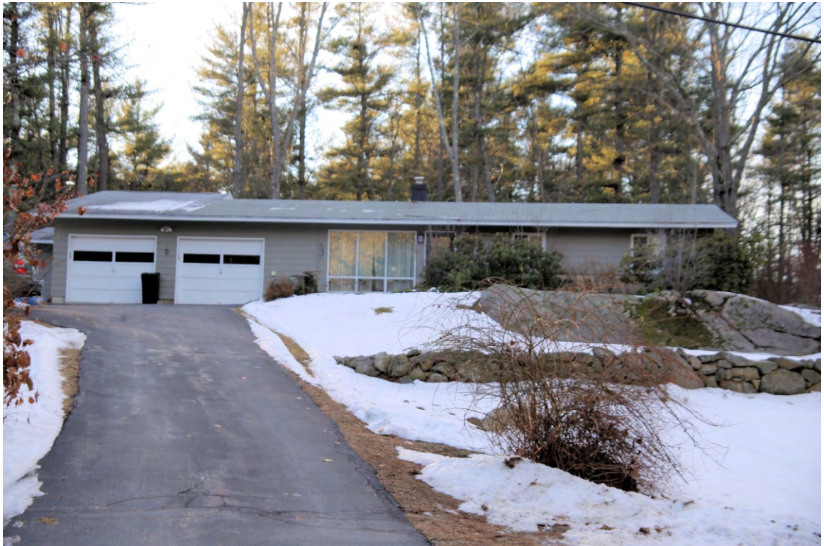
Photo 060) Edgewood Road Area – Davis Avenue ID: D-09, photo taken January 2016
