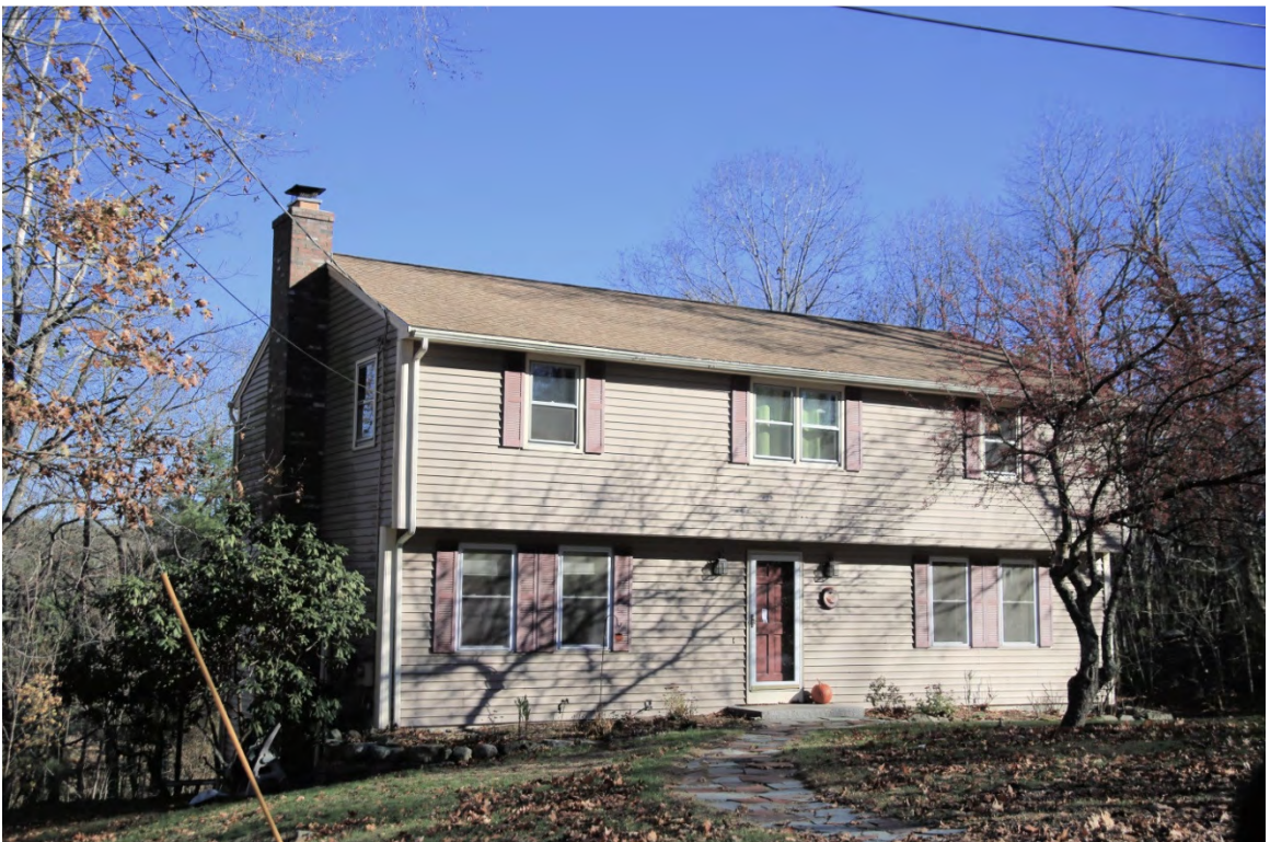
Photo 173) Wedgewood Development – 33 Pinecrest Lane ID: D-51, photo taken November 2015
