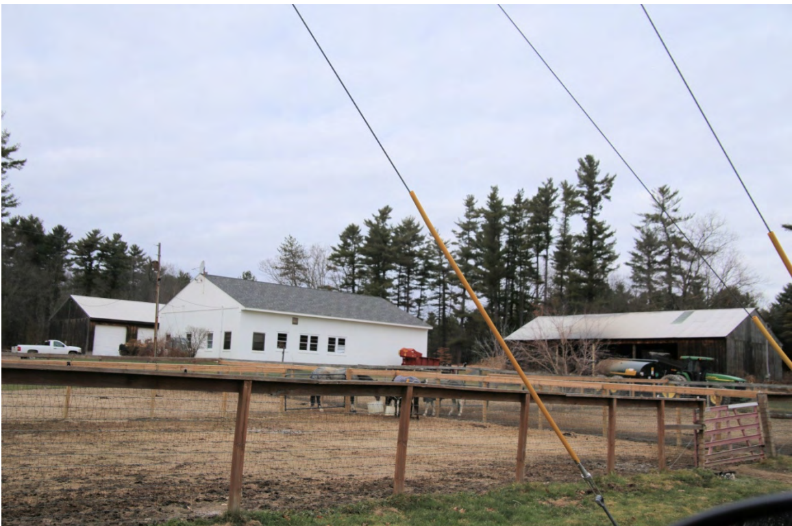
Photo 089) UNH Thompson School – Farm Services Buildings, Mast Road Extension Direction: N ID: D-17, photo taken December 2015
