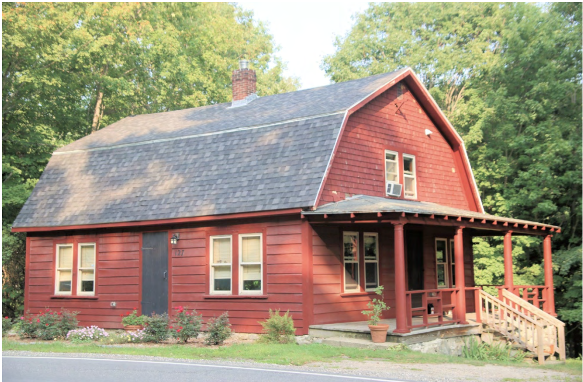
Photo 166) Newmarket-Bennett Road Farms Historic District – 127 Newmarket Road (DUR0013)
