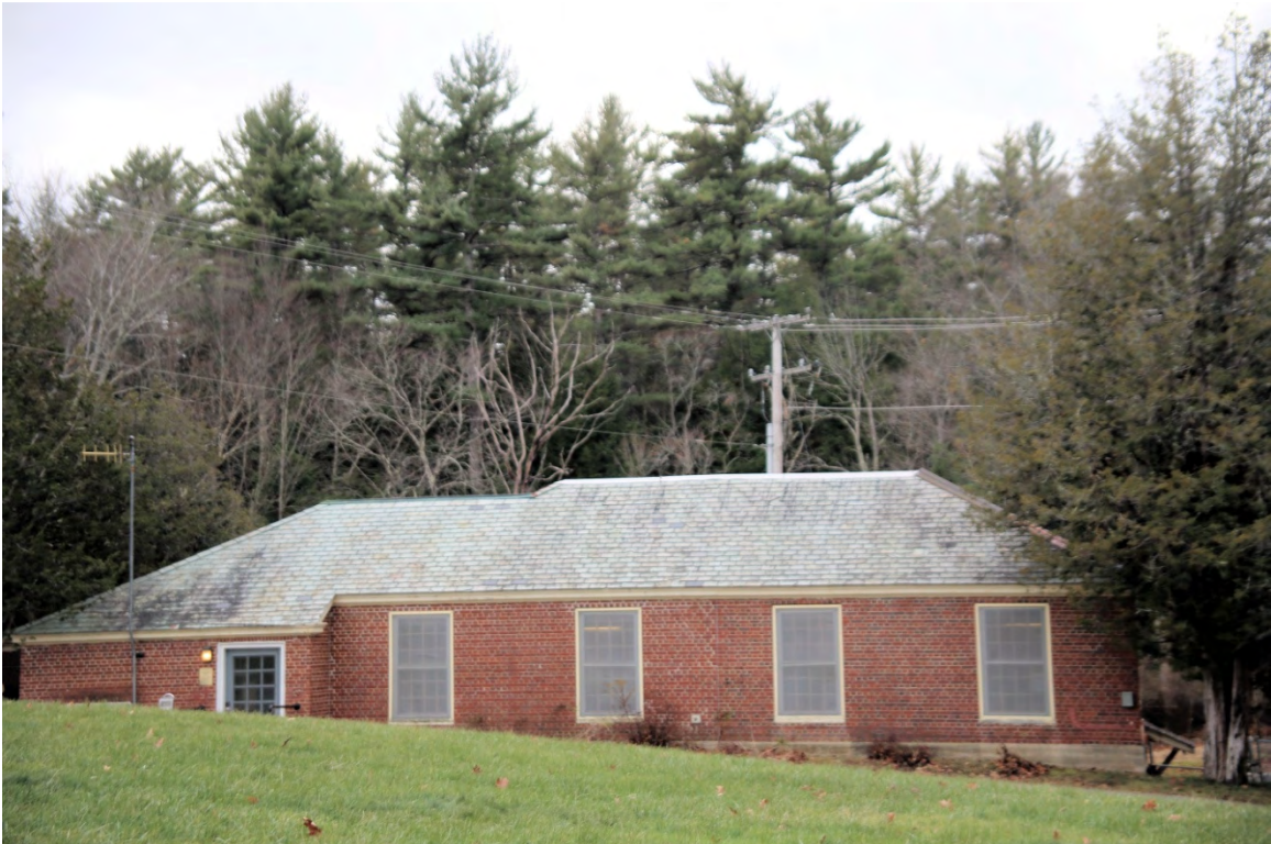
Photo 126) Waterworks Road – Waterworks ID: D-25, photo taken December 2015
