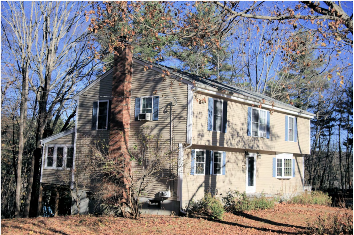
Photo 172) Wedgewood Development – 29 Pinecrest Lane ID: D-51, photo taken November 2015
