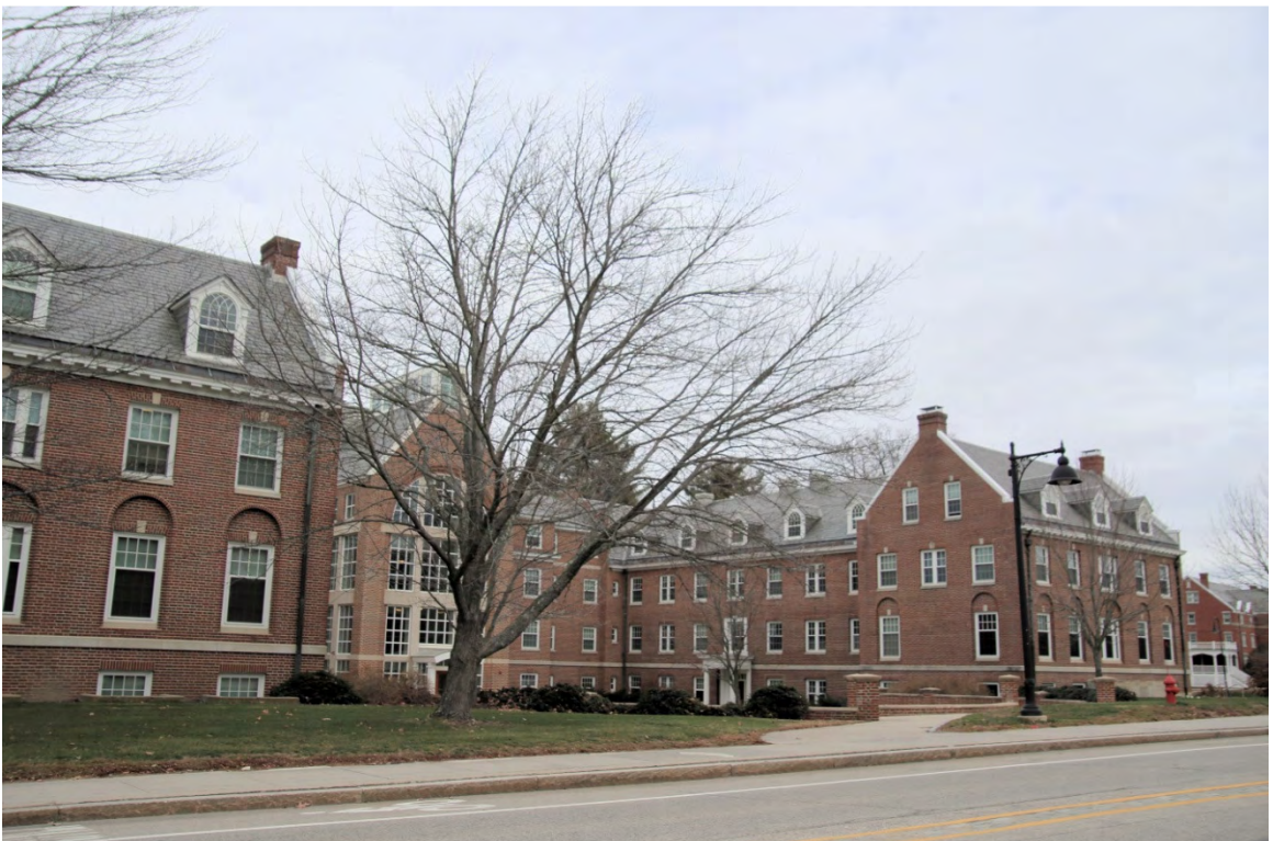
Photo 101) UNH – Main Street – Congreve Hall ID: D-21, photo taken December 2015
