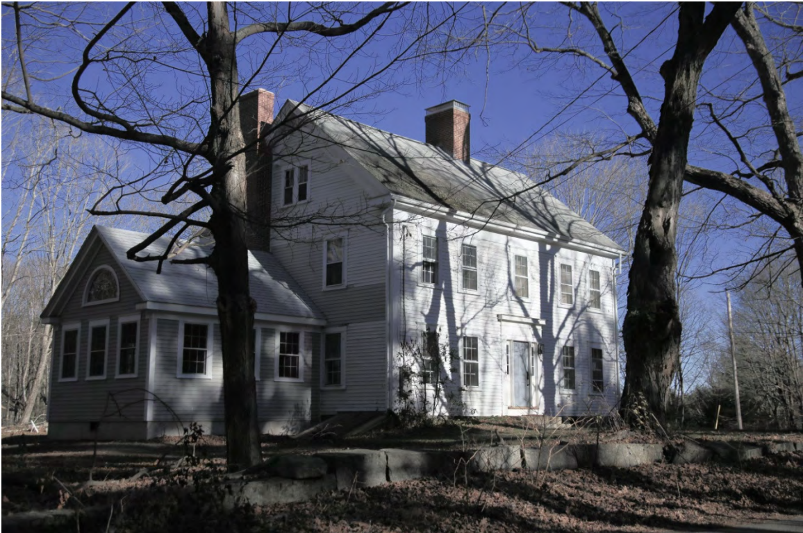
Photo 182) 129 Durham Point Road ID: D-60, photo taken November 2015
