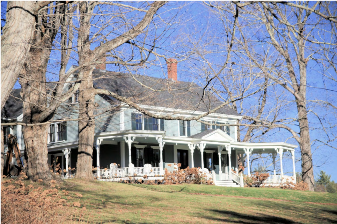
Photo 158) 90 Bennett Road – Thompson Inn (Highland Farm) ID: Outside Project Area, photo taken December 2015
