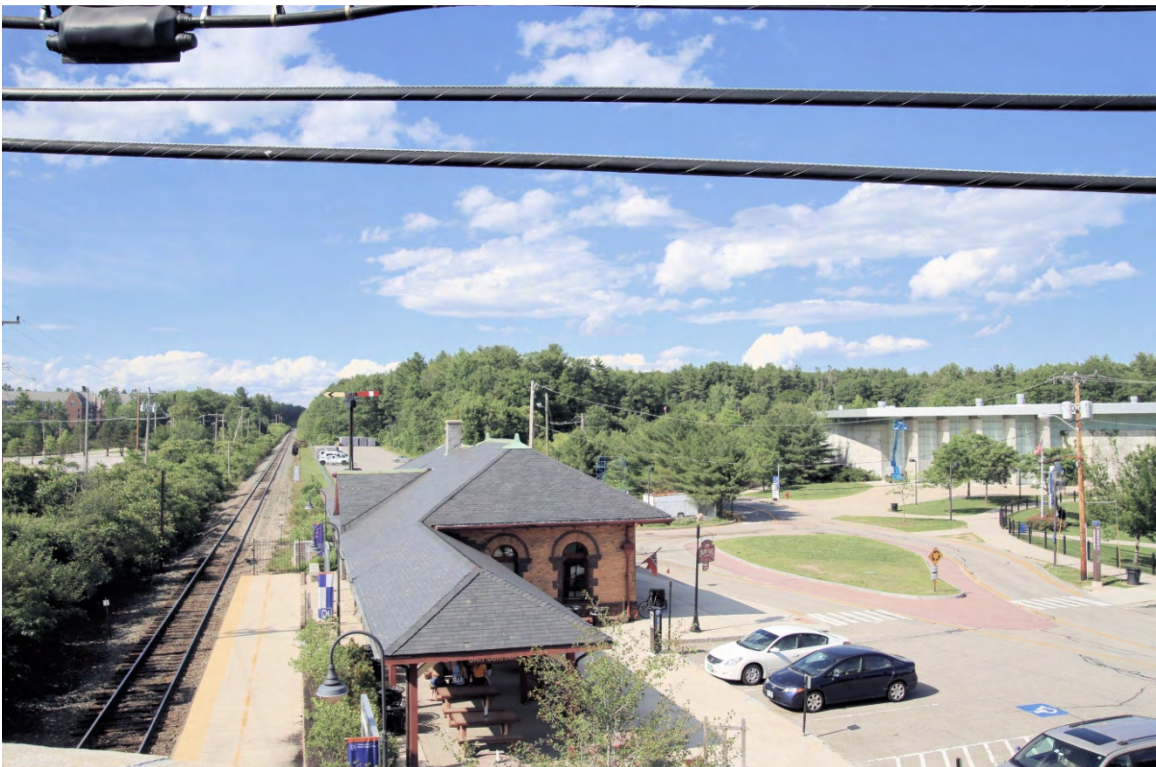
Photo 093) Durham-UNH Railroad Station, from Main Street Bridge
