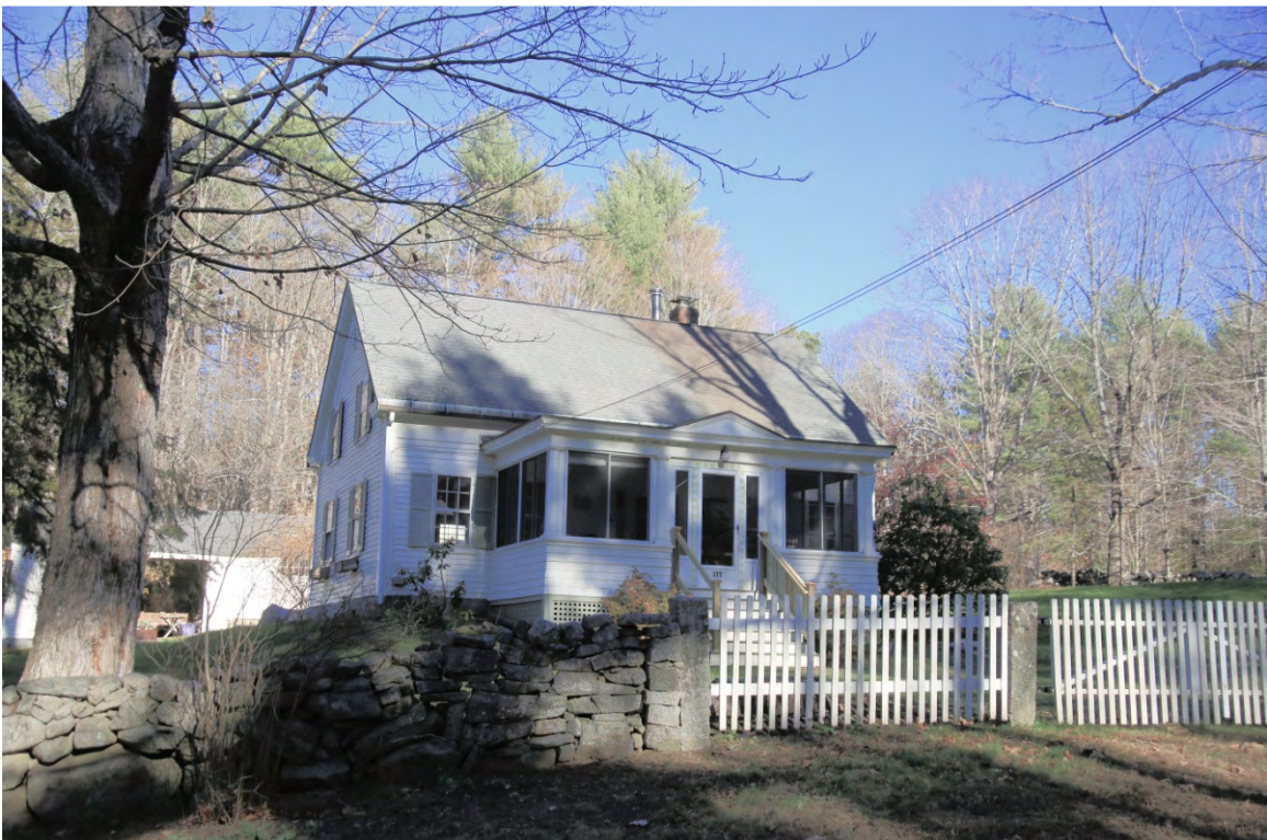
Photo 183) 177 Durham Point Road ID: D-61, photo taken November 2015
