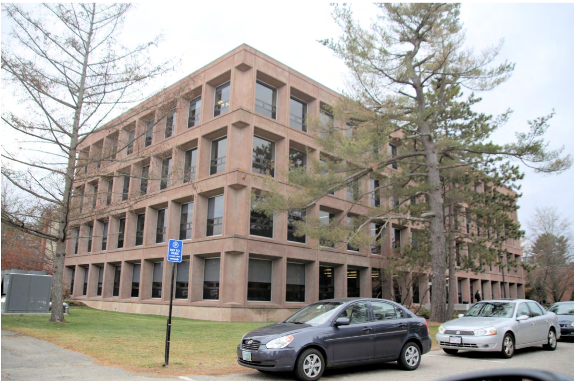
Photo 121) UNH – Academic Way – McConnell Hall ID: D-21, photo taken December 2015
