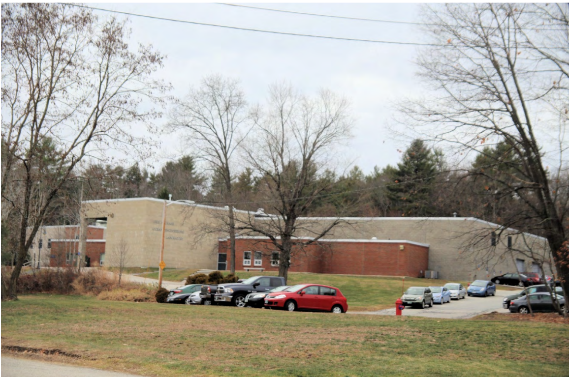
Photo 123) UNH – Colovos Road – Chase Ocean Engineering ID: D-21, photo taken December 2015
