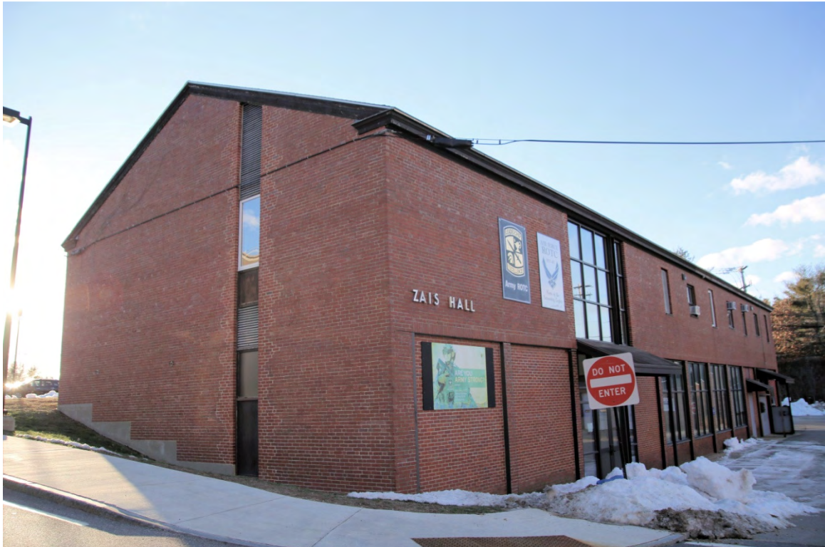
Photo 110) UNH – College Road – Zais Hall ID: D-21, photo taken January 2016
