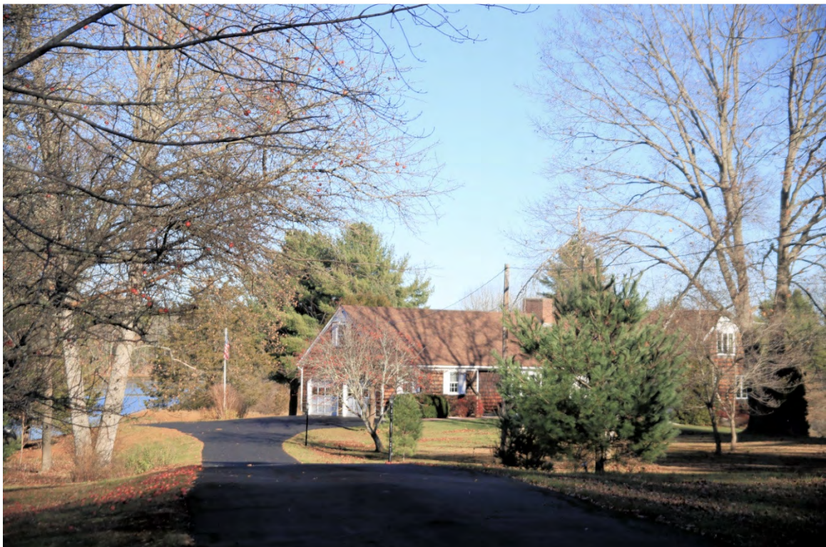
Photo 175) 26 Mathes Cove Road ID: D-53, photo taken November 2015
