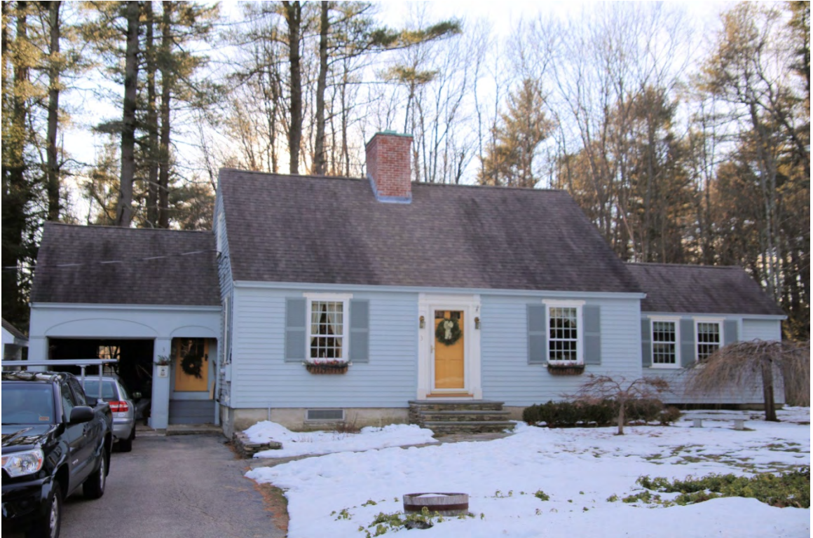
Photo 058) Edgewood Road Area – Davis Avenue ID: D-09, photo taken January 2016
