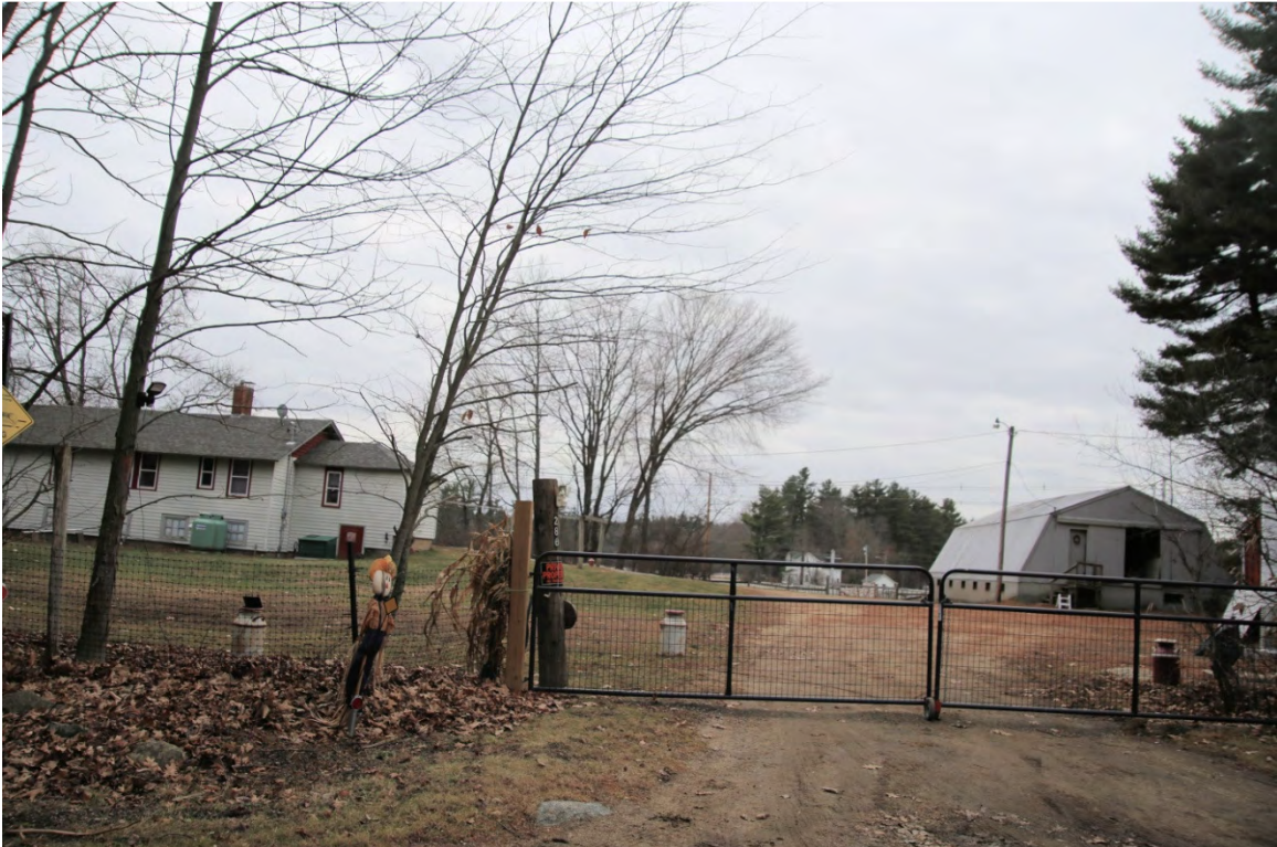
Photo 088) UNH Thompson School – Light Horse Classroom, Mast Road Extension Direction: SW ID: D-17, photo taken December 2015
