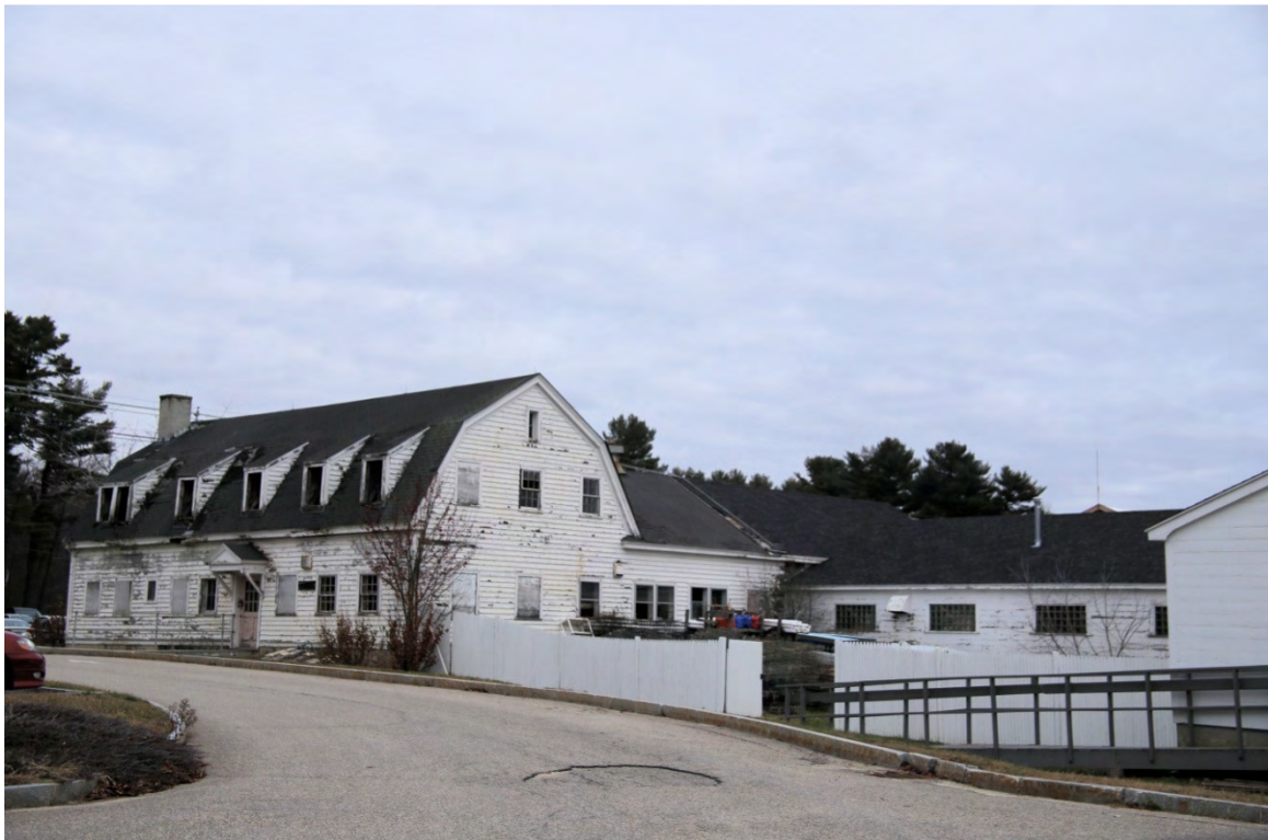
Photo 085) UNH Thompson School – Old Dairy Barn ID: D-17, photo taken December 2015
