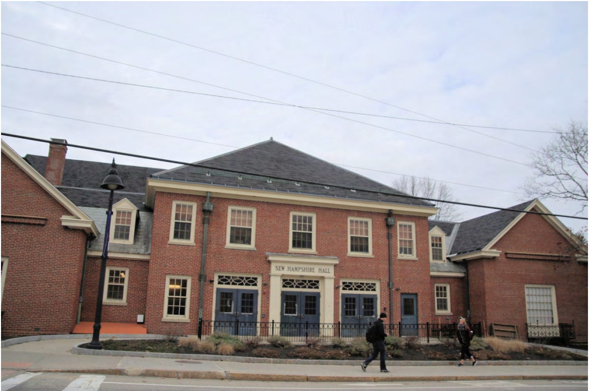
Photo 100) UNH – 124 Main Street – New Hampshire Hall ID: D-21, photo taken December 2015
