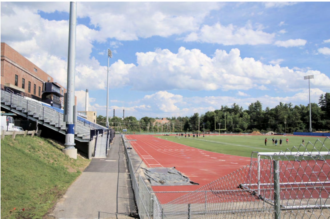
Photo 097) UNH – Stadium and football field ID: D-21, photo taken June 2015
