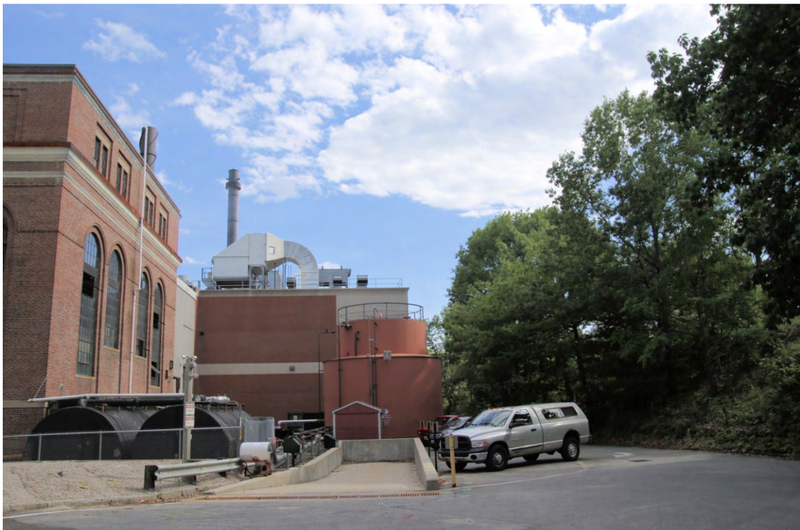
Photo 109) UNH – Rear of Heating Plant, railroad tracks at right ID: D-21, photo taken June 2015
