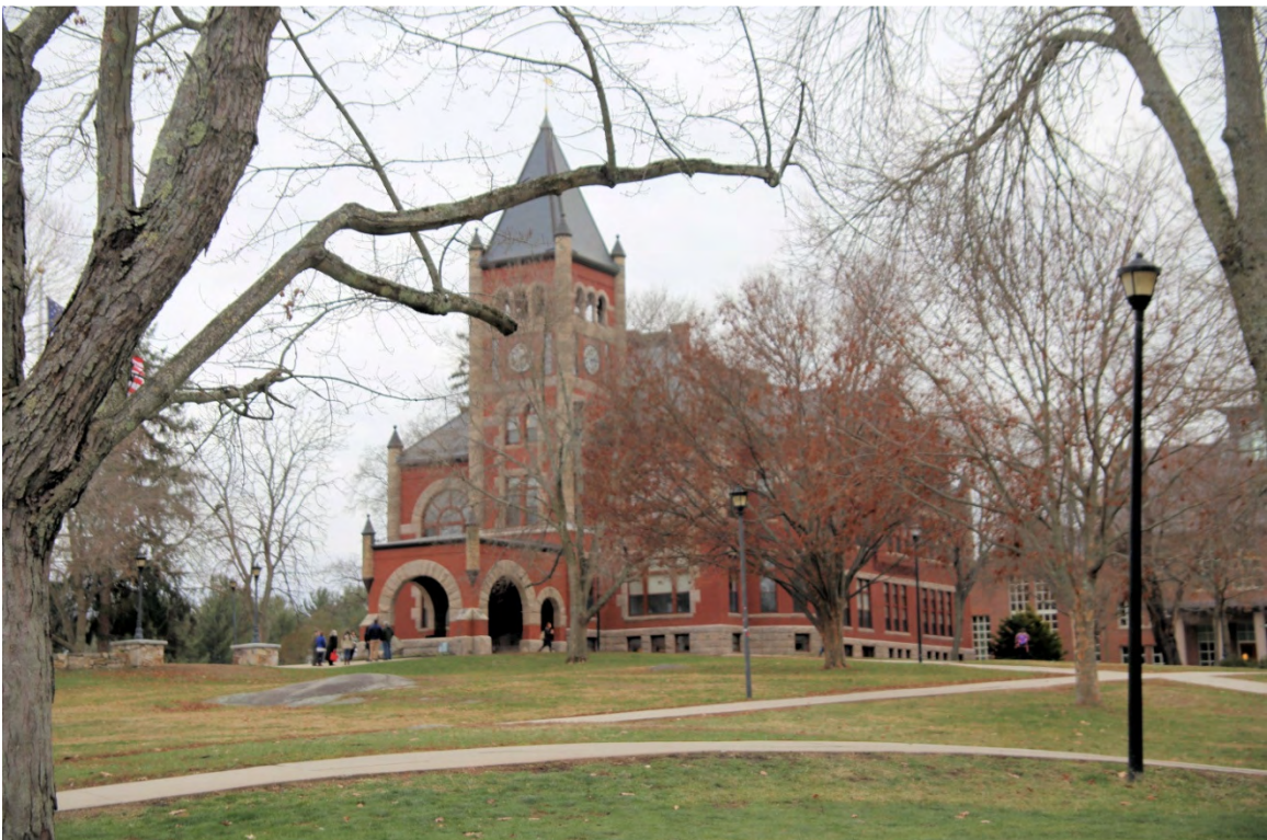
Photo 103) UNH – Main Street – Thompson Hall (DUR0010, on National Register) ID: D-22, photo taken December 2015
