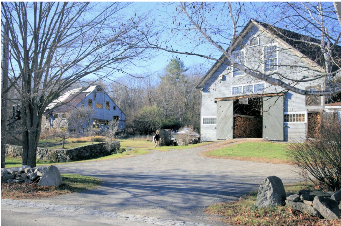
Photo 193) 300 Durham Point Road barns ID: D-67, photo taken November 2015
