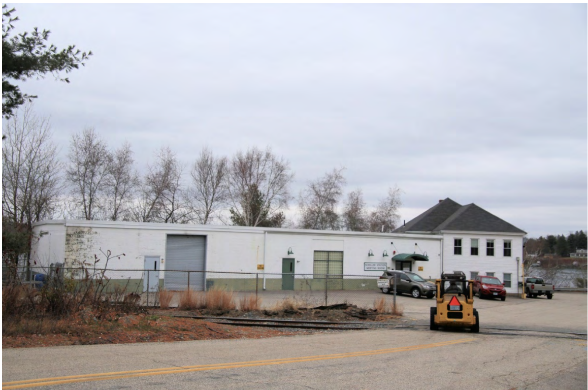
Photo 290) Schiller Power Plant “meeting room” ID: N-87, photo taken December 2015
