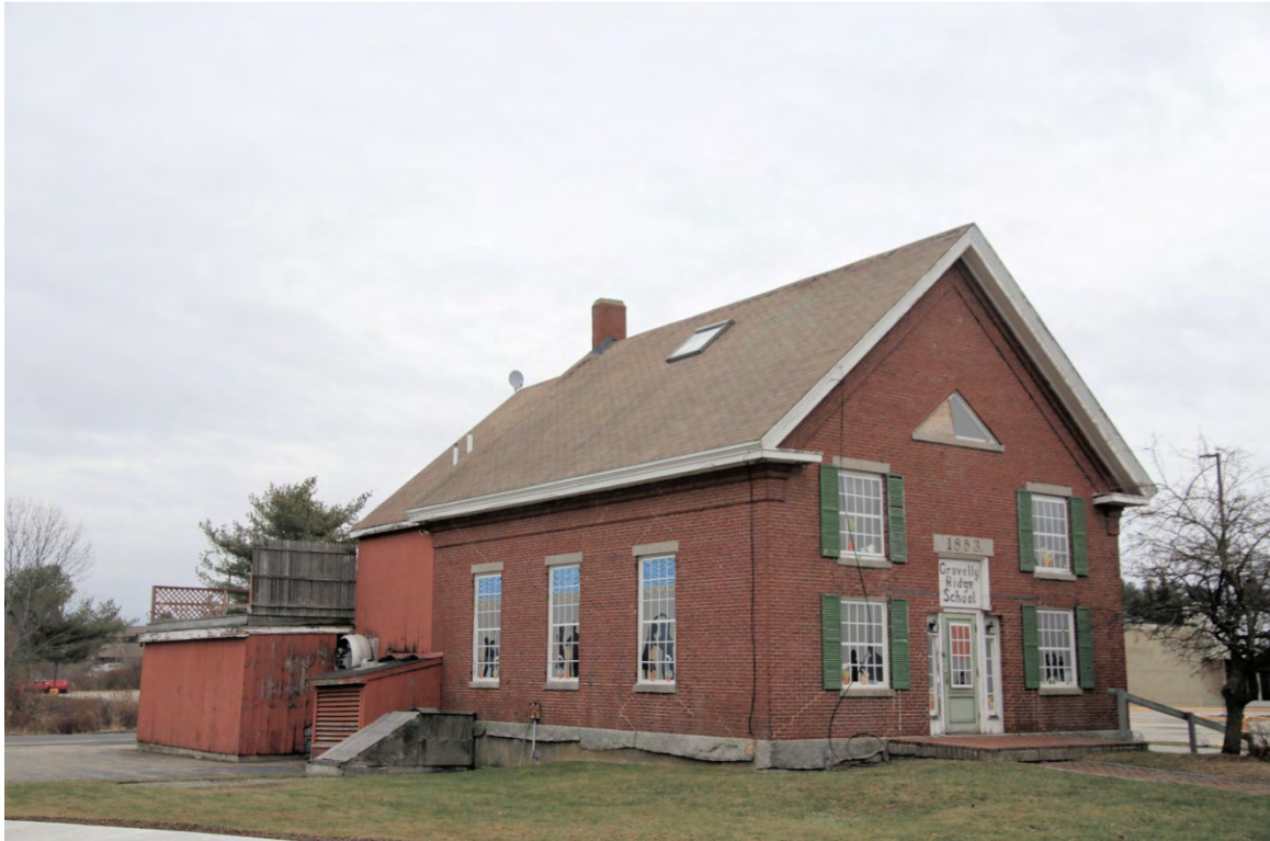
Photo 301) 1465 Woodbury Avenue – Woodbury Schoolhouse ID: P-07, photo taken December 2015
