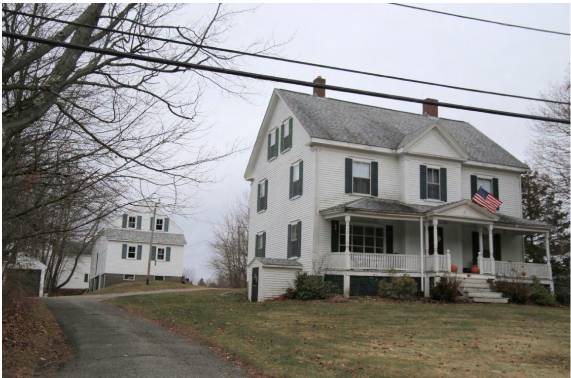
Photo 204) 251 Little Bay Road – Cyrus Frink House (#67) ID: N-10, photo taken December 2015
