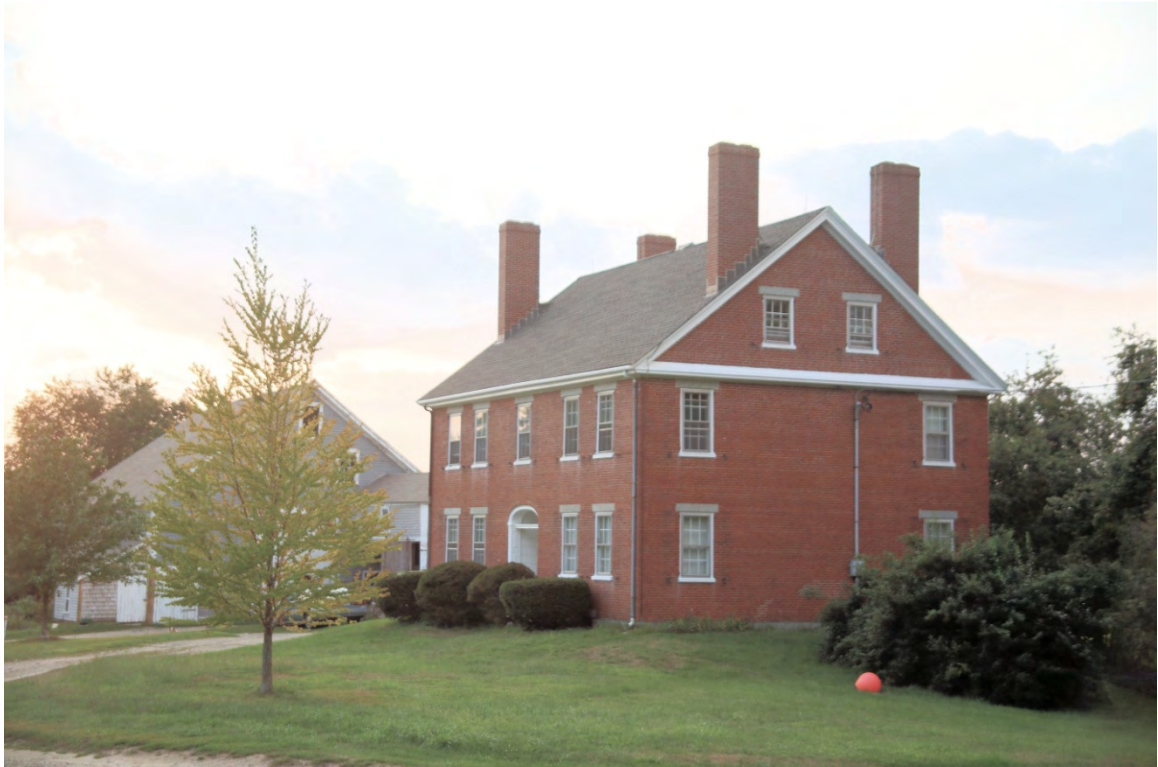
Photo 213) Newington Center Historic District – 272 Nimble Hill Road – Frink Farm (#57)
