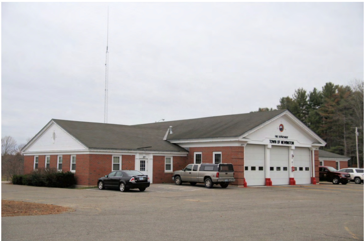
Photo 234) 80 Fox Point Road – Newington Fire Station ID: N-24, photo taken December 2015
