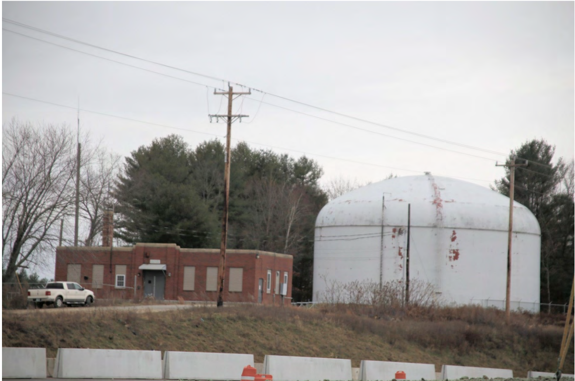
Photo 275) Arboretum Drive, Portsmouth Water Department, Auxiliary Pumping Station (NWN0228)
