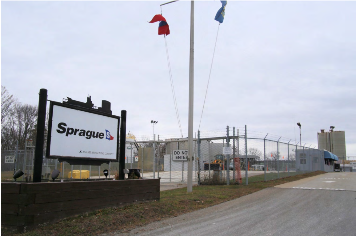
Photo 263) 372 Shattuck Way – Sprague Energy Plant (Area NWN-SP) ID: N-58, photo taken December 2015
