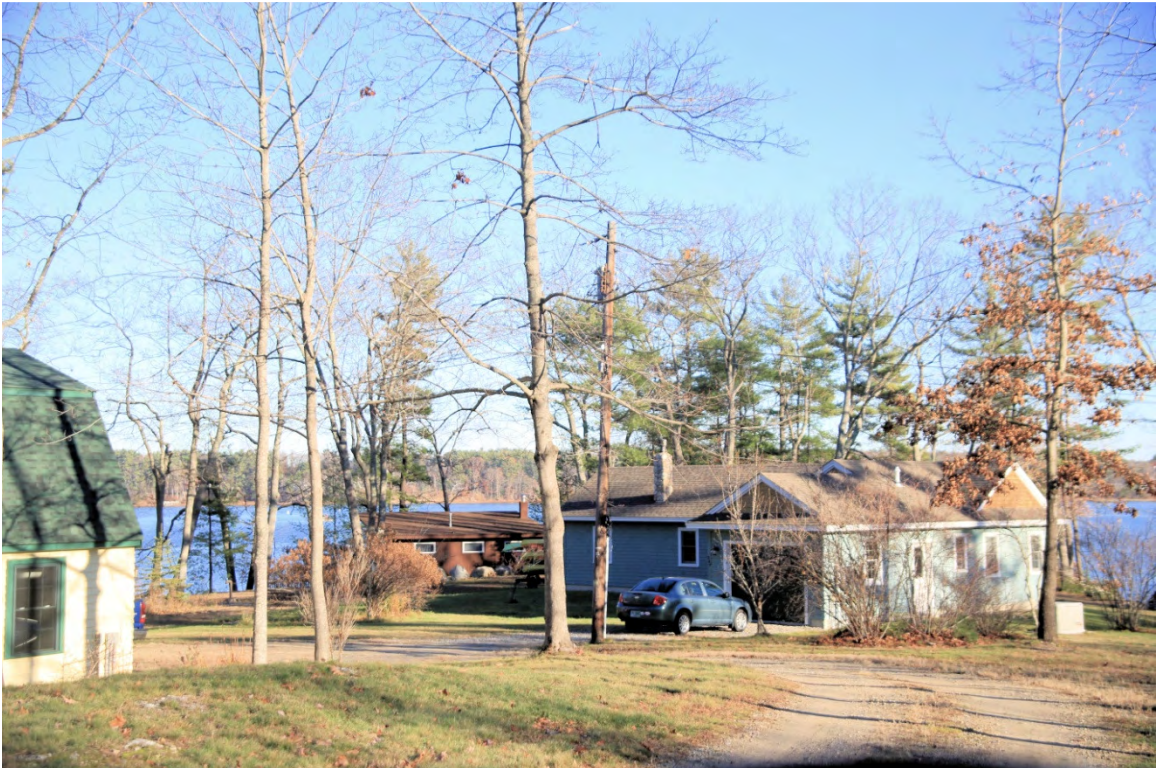
Photo 190) 267 Durham Point Road ID: D-64, photo taken November 2015
