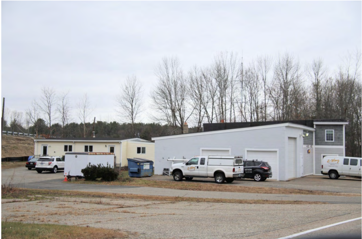
Photo 269) 21 River Road (#184) and 23 River Road (#183, NWN0183) ID: N-62 and N-63, photo taken December 2015
