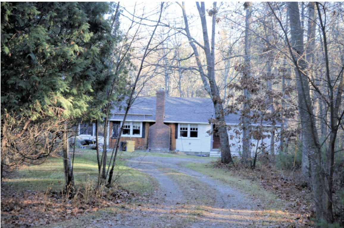
Photo 191) 275 Durham Point Road ID: D-65, photo taken November 2015
