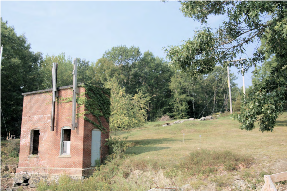
Photo 196) Off Durham Point Road – Cable Switch House ID: D-72, photo taken September 2015
