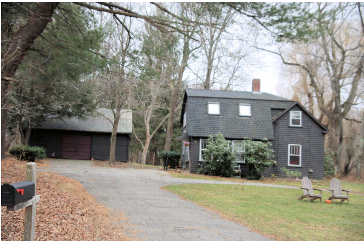
Photo 274) 58 Patterson Lane – Wall Cottage (NWN0199) ID: N-68, photo taken December 2015
