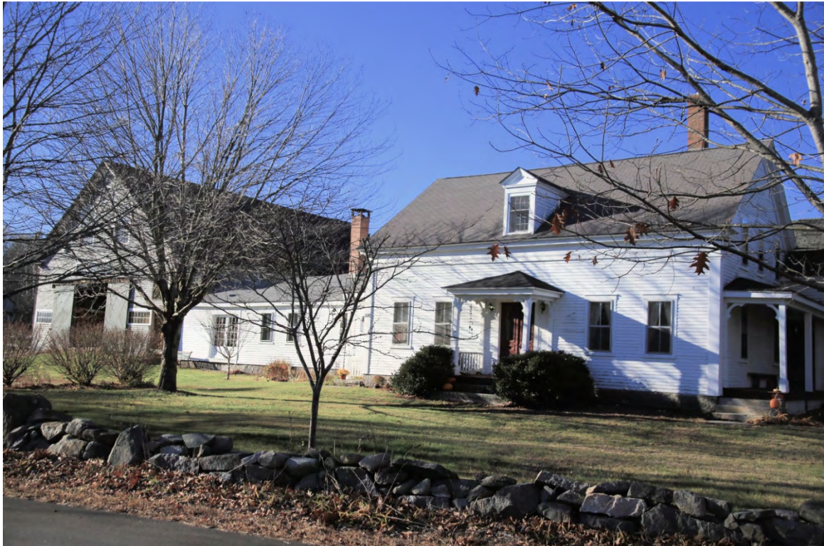
Photo 192) 300 Durham Point Road ID: D-67, photo taken November 2015
