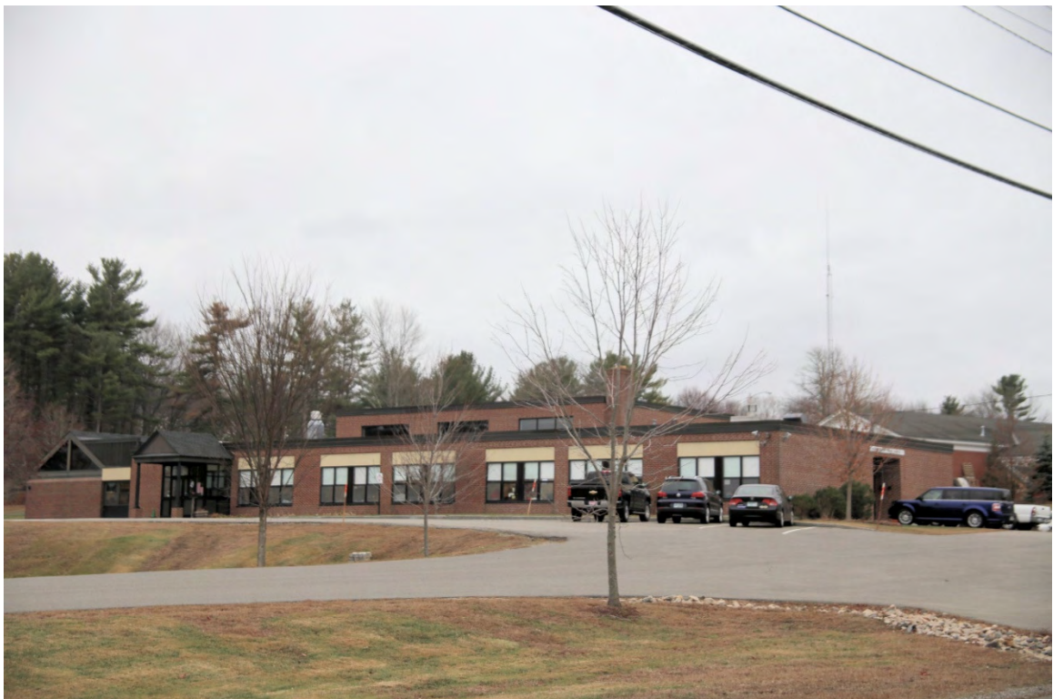
Photo 252) 133 Nimble Hill Road – Newington Elementary School ID: N-42, photo taken December 2015
