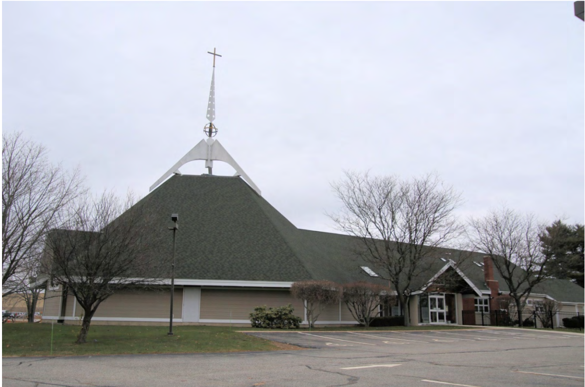
Photo 279) 22 Fox Run Road – Holy Trinity Lutheran Church (#231) ID: N-77, photo taken December 2015
