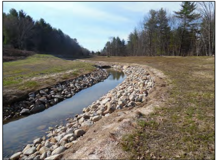
Stream NS50: View upstream (F#3) [Mat Bridge – No Impacts]
