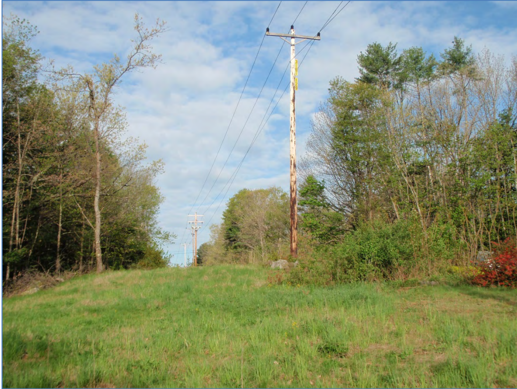
Photo 1 Frost Road, Durham
