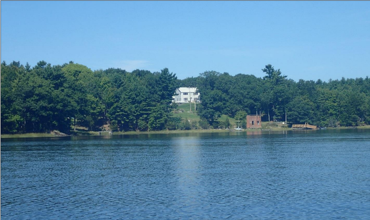
View from Little Bay boat channel looking west at Durham shoreline toward the Project corridor. A monopole and perhaps a portion of a 3-pole wooden structure will potentially be visible. The existing brick structure, a historic element, will be retained in this location.
