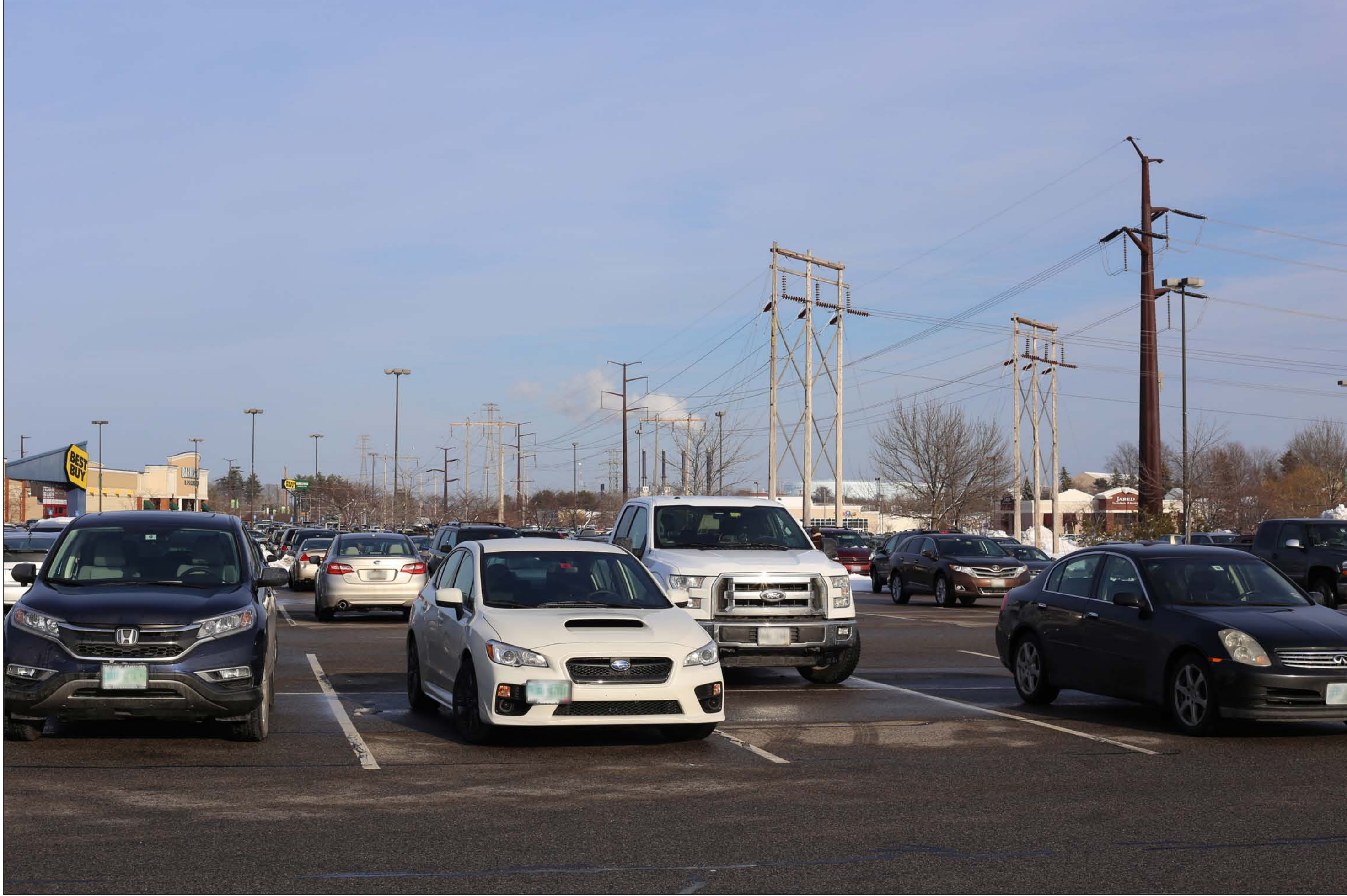
EXHIBIT 16: EXISTING CONDITIONS AT NEWINGTON MALL SHOPPING CENTER, NEWINGTON (SHEET 2 OF 3) SEACOAST RELIABILITY PROJECT VISUAL ASSESSMENT February 2016
