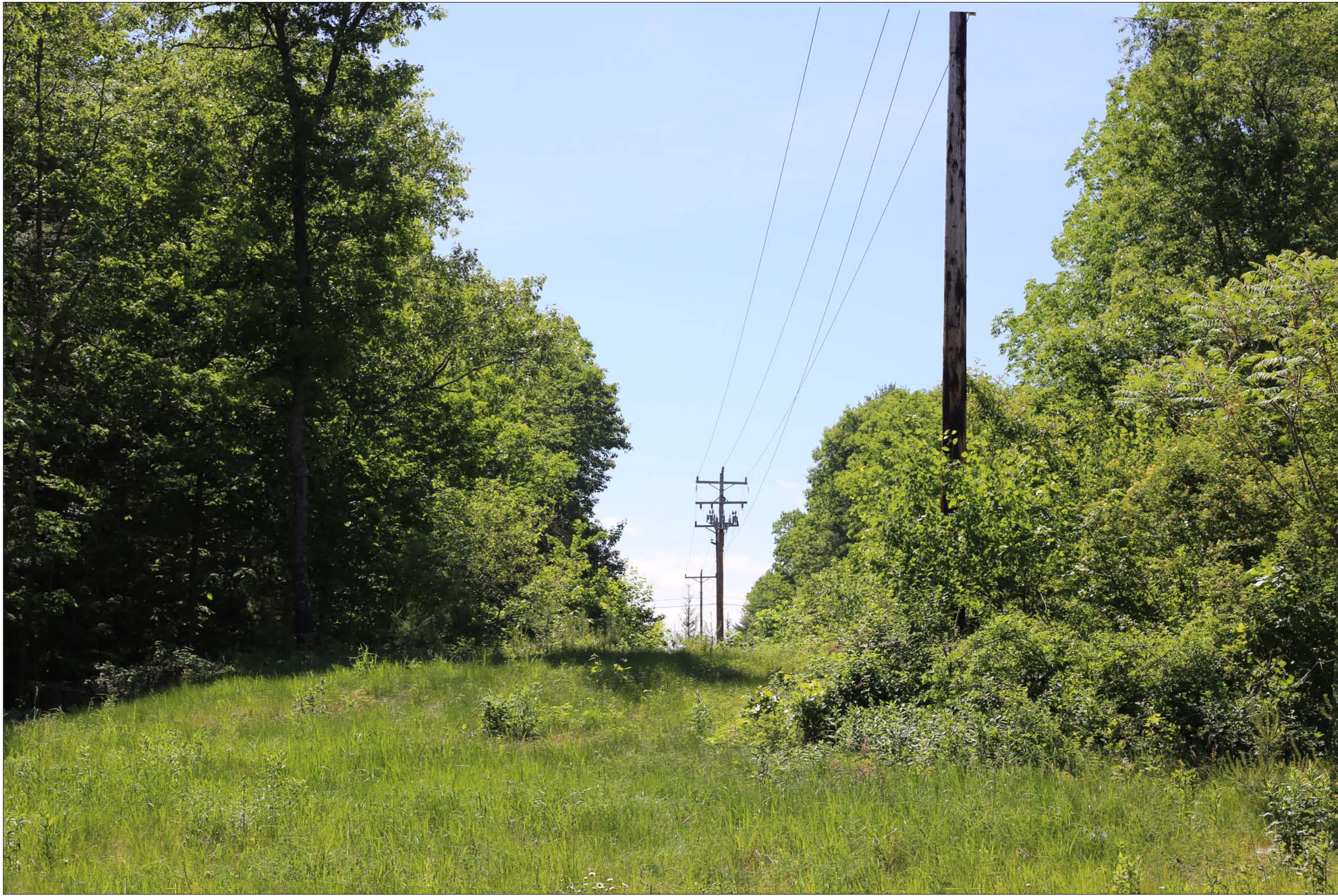
EXHIBIT 15: EXISTING CONDITIONS AT FROST DRIVE, DURHAM (SHEET 2 OF 3)
