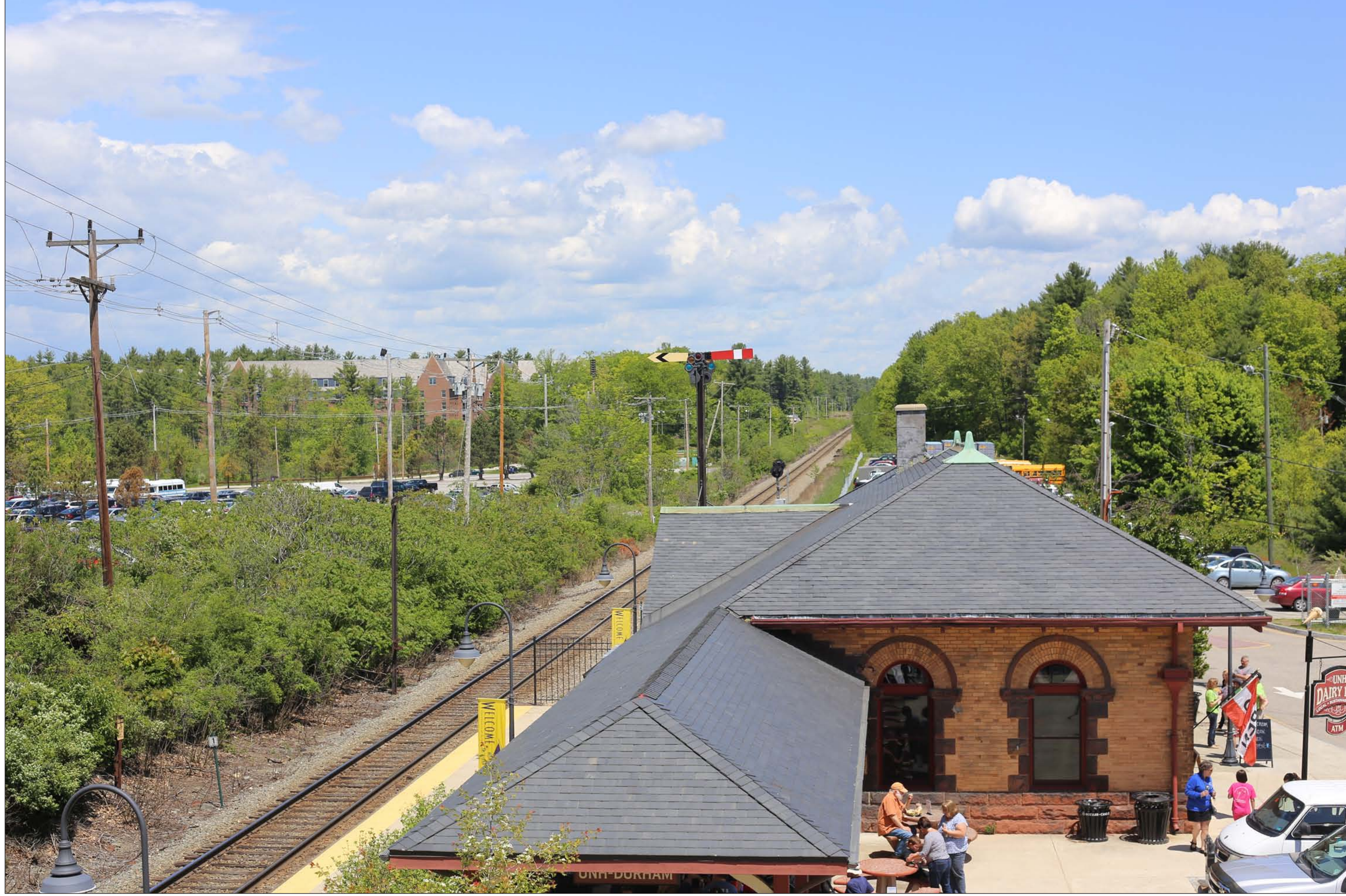
EXHIBIT 8: EXISTING CONDITIONS FROM DURHAM MAIN STREET/UNH DAIRY BAR, DURHAM, NH (SHEET 2 OF 3)
