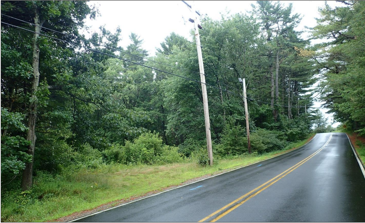
7. Little Bay Road (#45): Existing utility lines along Little Bay Road
