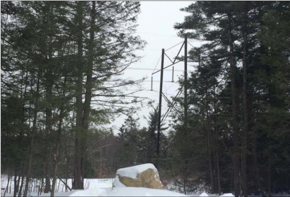
Figure 4.1.3 Photograph of Study Area #3 -- 345 kV Cross Section
