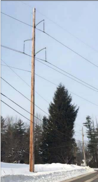
Figure 4.1.4 Photograph of Study Area #3 -- 115 kV Cross Section
