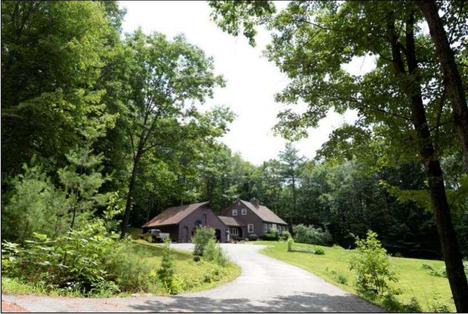
Figure 5.2.6.3 Photograph of Lot 48 (non-abutting) as Improved (taken 7/14/2014)
