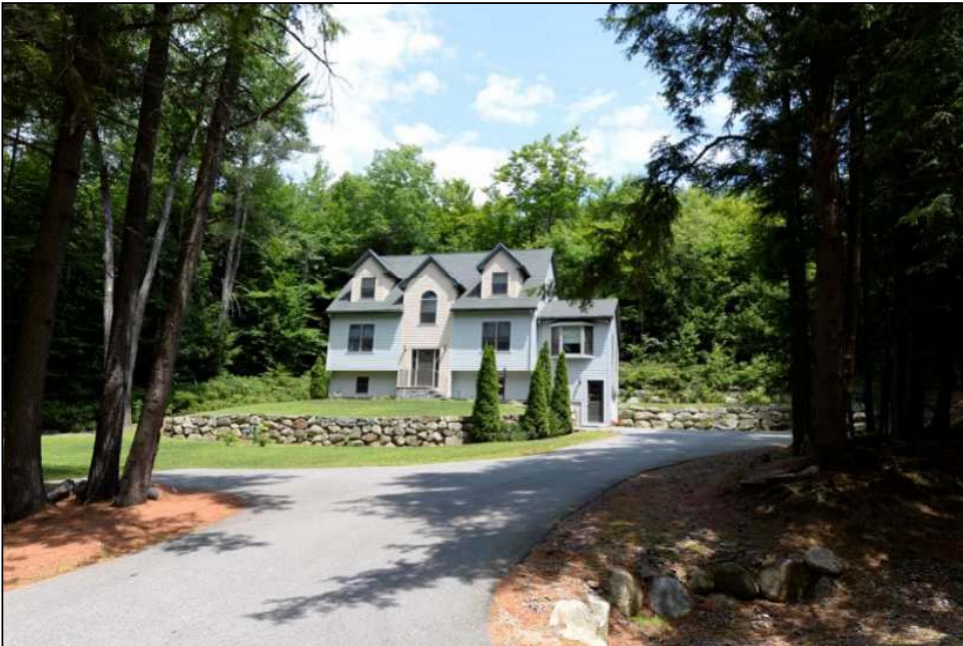
Figure 5.2.6.4 Photograph of Lot 71 (non-abutting) as Improved (taken 7/14/2014)
