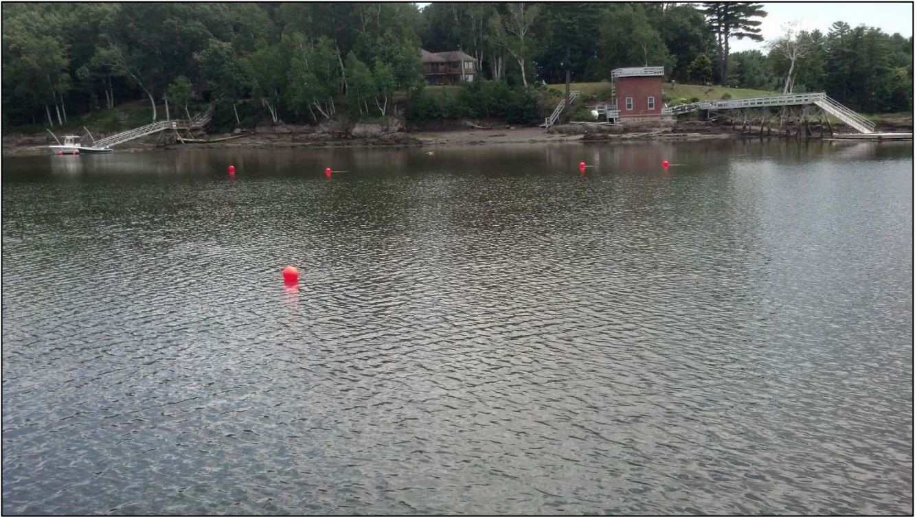
Figure 4: View of the work area at the Eastern Shore landing approach; floats were affixed to the as-found cables by divers.
