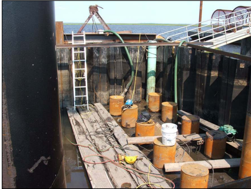
Marine Cofferdam Construction
