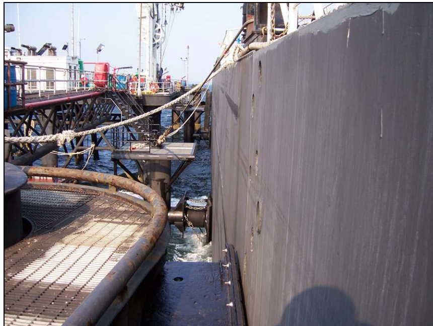
Fender Installation at Offshore Platform
