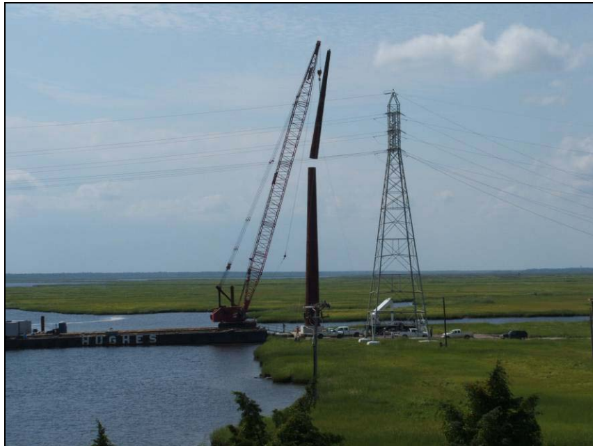
Transmission Tower Installation
