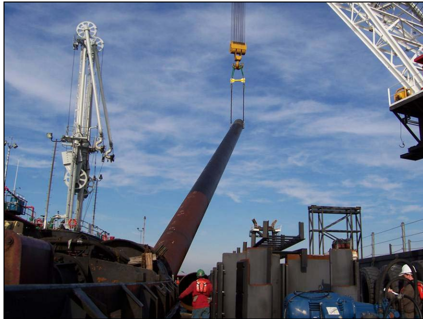
170 Foot Mono-Pile Installation at Offshore Platform
