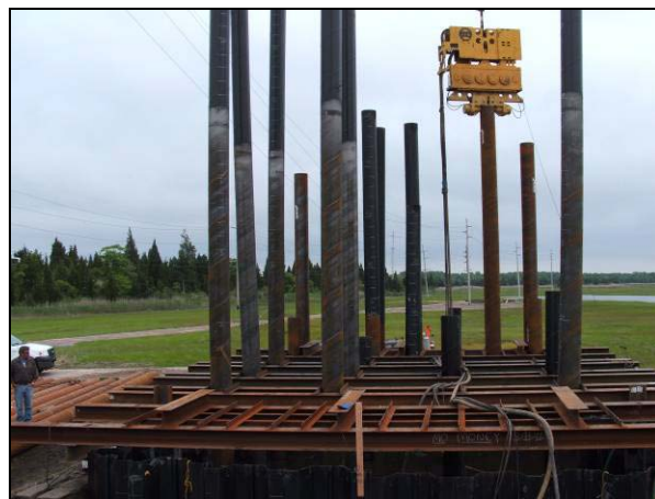
Marine Pile driving at a River Estuary site
