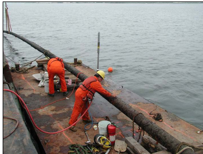
HDD Tie-in of existing 12" Submarine product line
