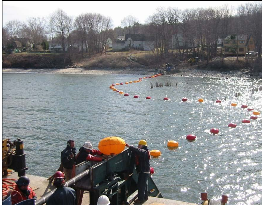
Turnkey Submarine Power Cable Installation Fox Island ME
