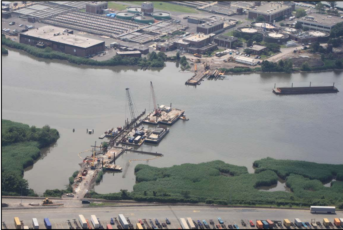
Submarine Pipeline Installation
