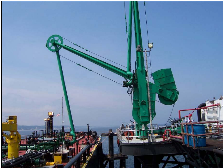
Loading Arm installation at offshore platform
