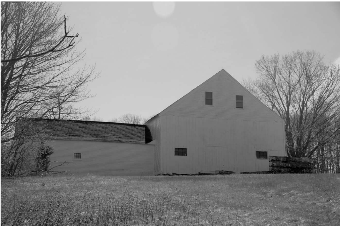
Photo 7) Rear (northeast elevation) of nineteenth-century barn
