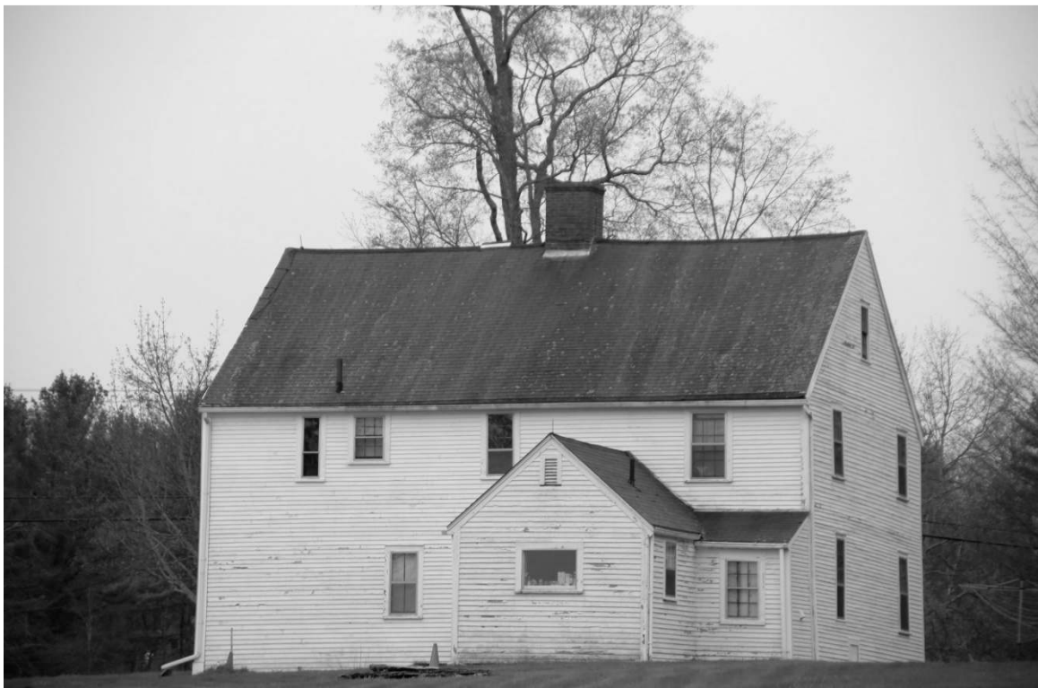
Photo 9) Rear (north) and west elevations of Adams House Date taken: May 2016
