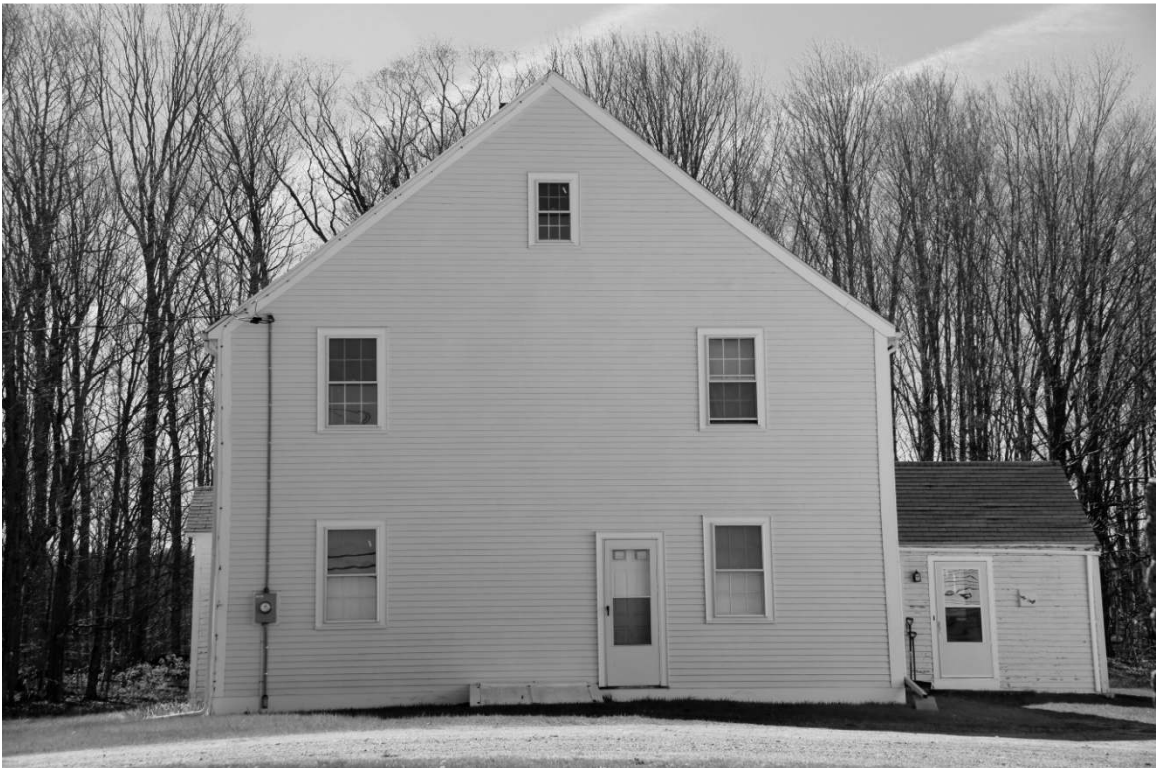
Photo 3) Adams House, east gable end and rear ell
