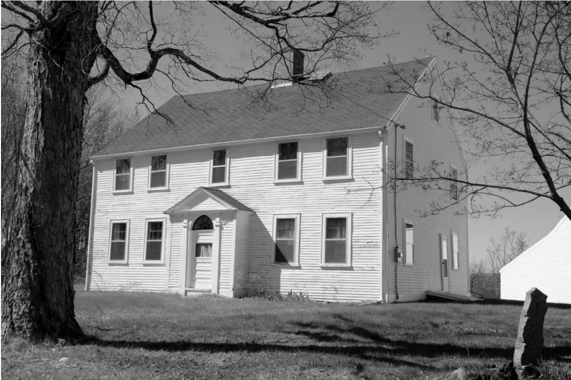
Photo 2) Adams House, façade (south) and east elevations
