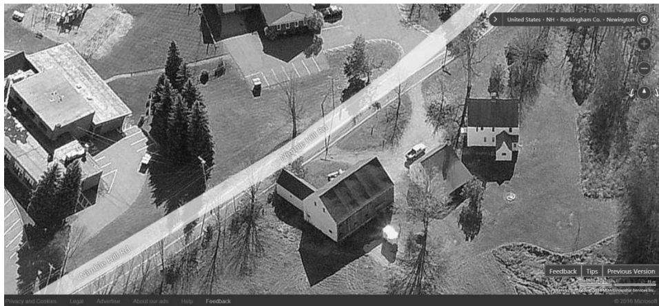
Bird's-Eye of rear of barns and house and elementary school across the street, facing south (Bing map)
