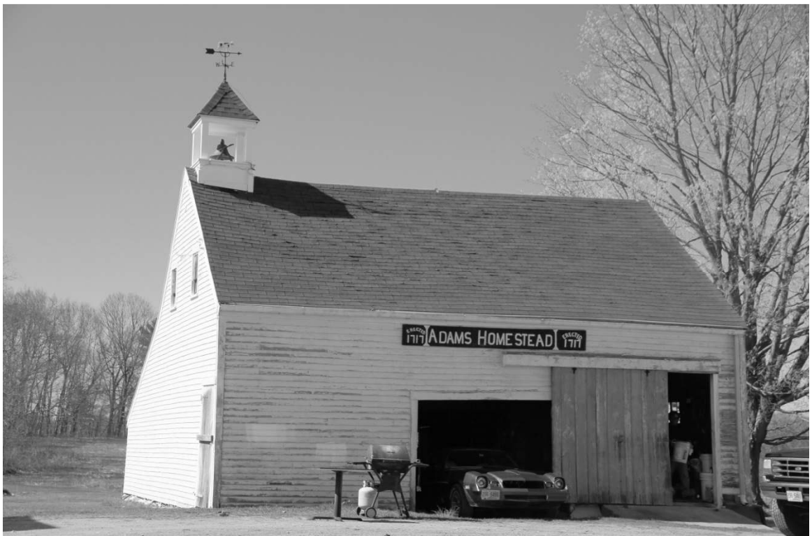
Photo 5) English barn, southwest and southeast elevations
