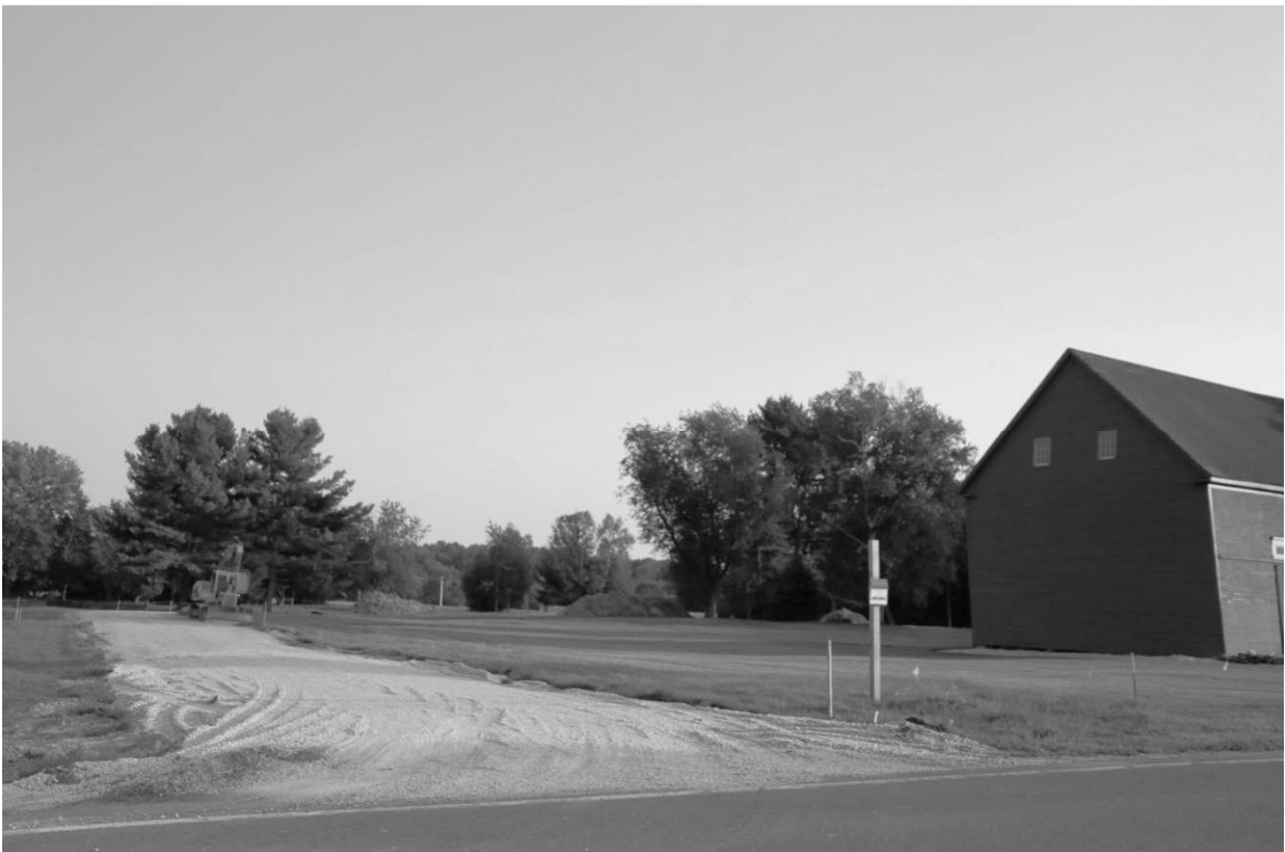
Photo 7) Driveway construction, new house site Date taken: August 2015
