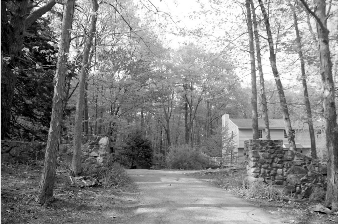
Photo 52) 1 Langley Road stone gates to former Mathes property Date taken: May 2016
