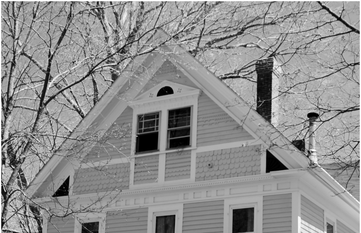
Detail of Photo 16, 253 Durham Point Road, gable detail (NE)
