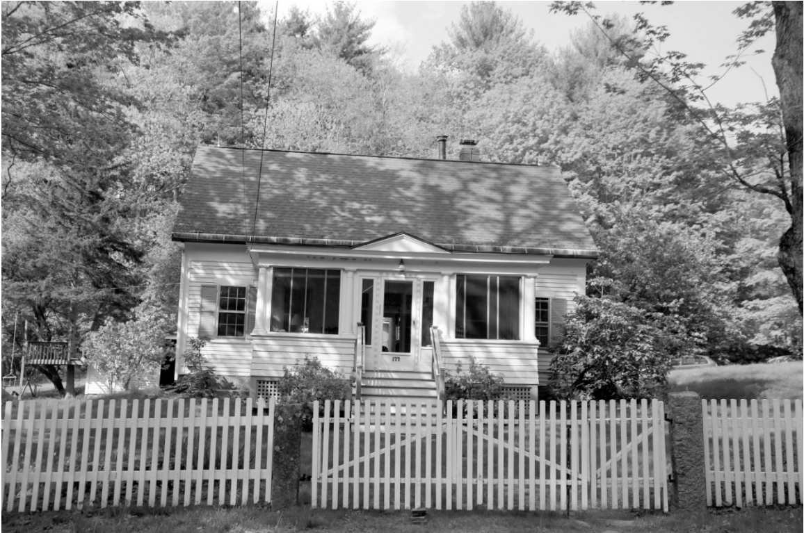
Photo 48) 177 Durham Point Road façade Date taken: May 2016
