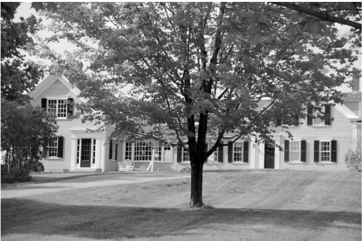
Photo 63) 15 Langley Road, shows entry detail Date taken: May 2016
