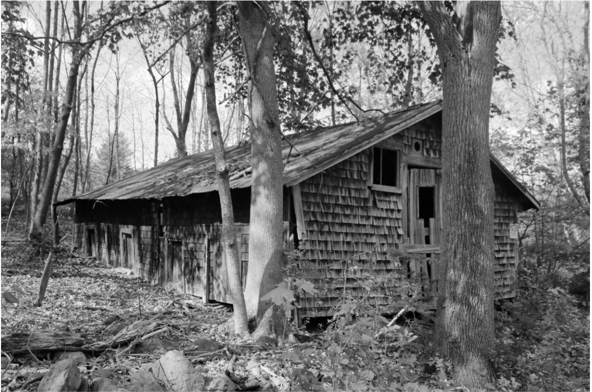
Photo 68) Shed on parcel 12-12-00 Date taken: May 2016
