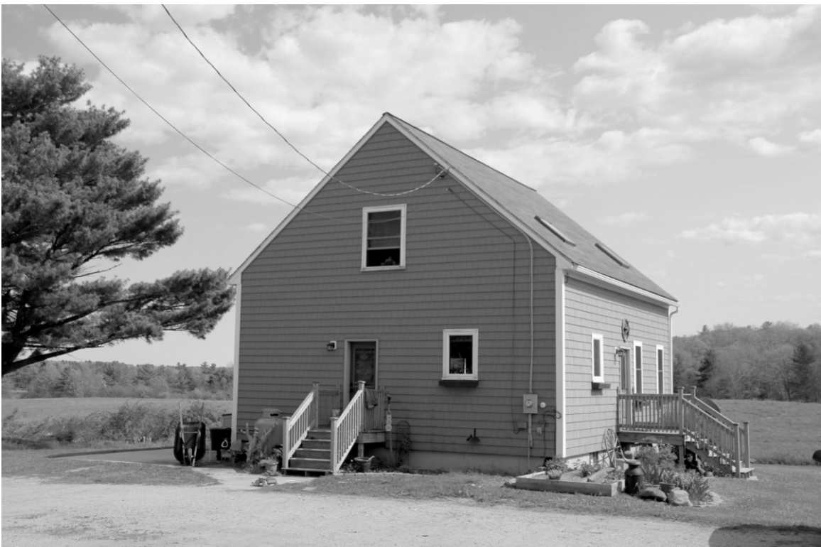
Photo 73) 50 Langley Road house-shop Date taken: May 2016
