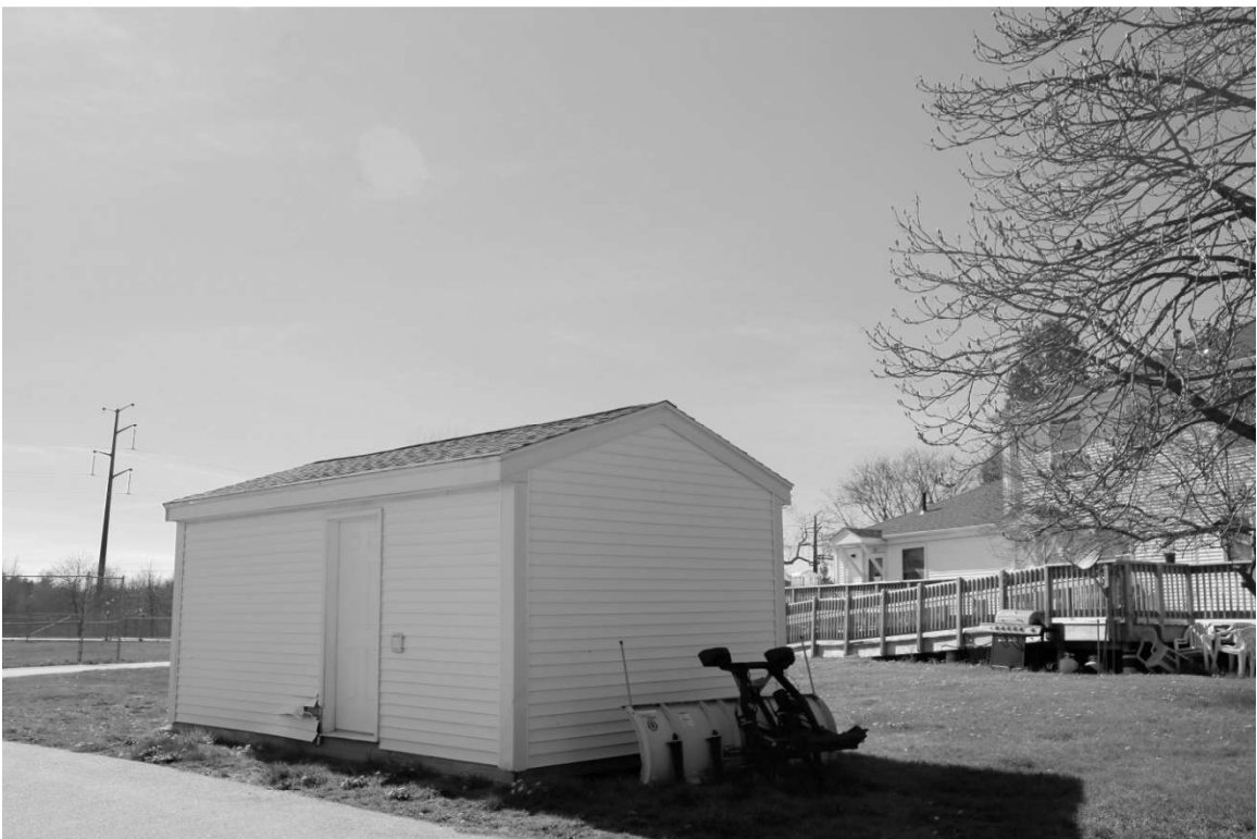
Photo 12) Shed with Building B-5 in background
