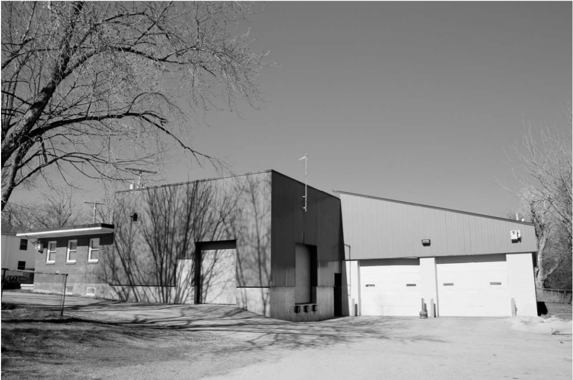
Photo 11) Recent Additions to Office/Recreation/Maintenance/Powerhouse
