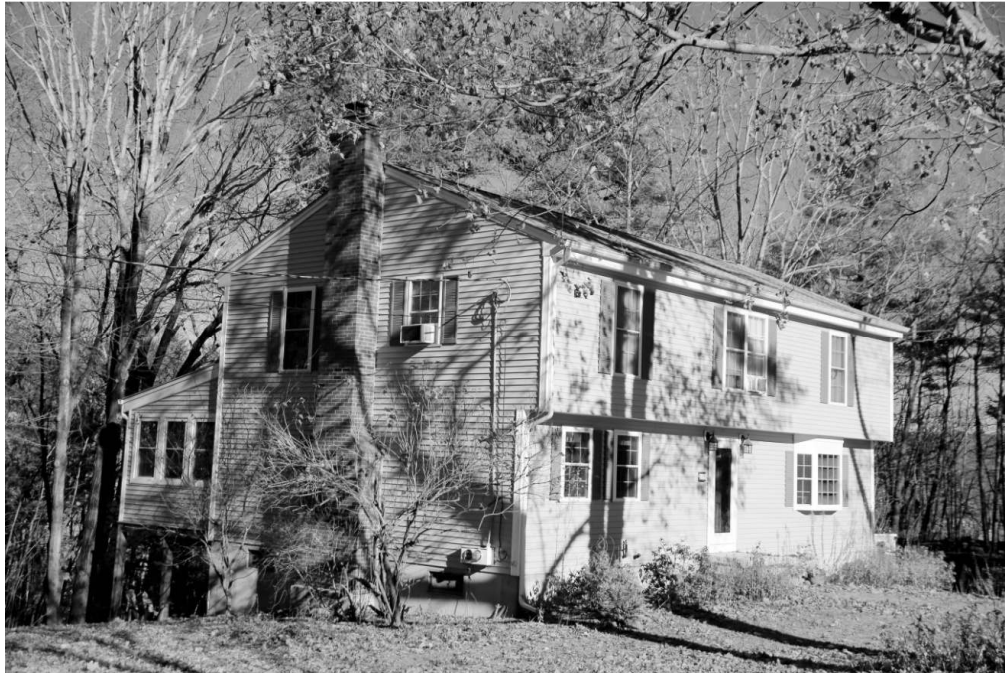
Wedgewood Development – 29 Pinecrest Lane, Durham
