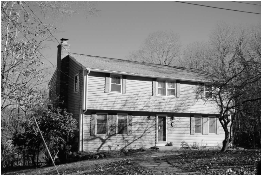
Wedgewood Development – 33 Pinecrest Lane, Durham
