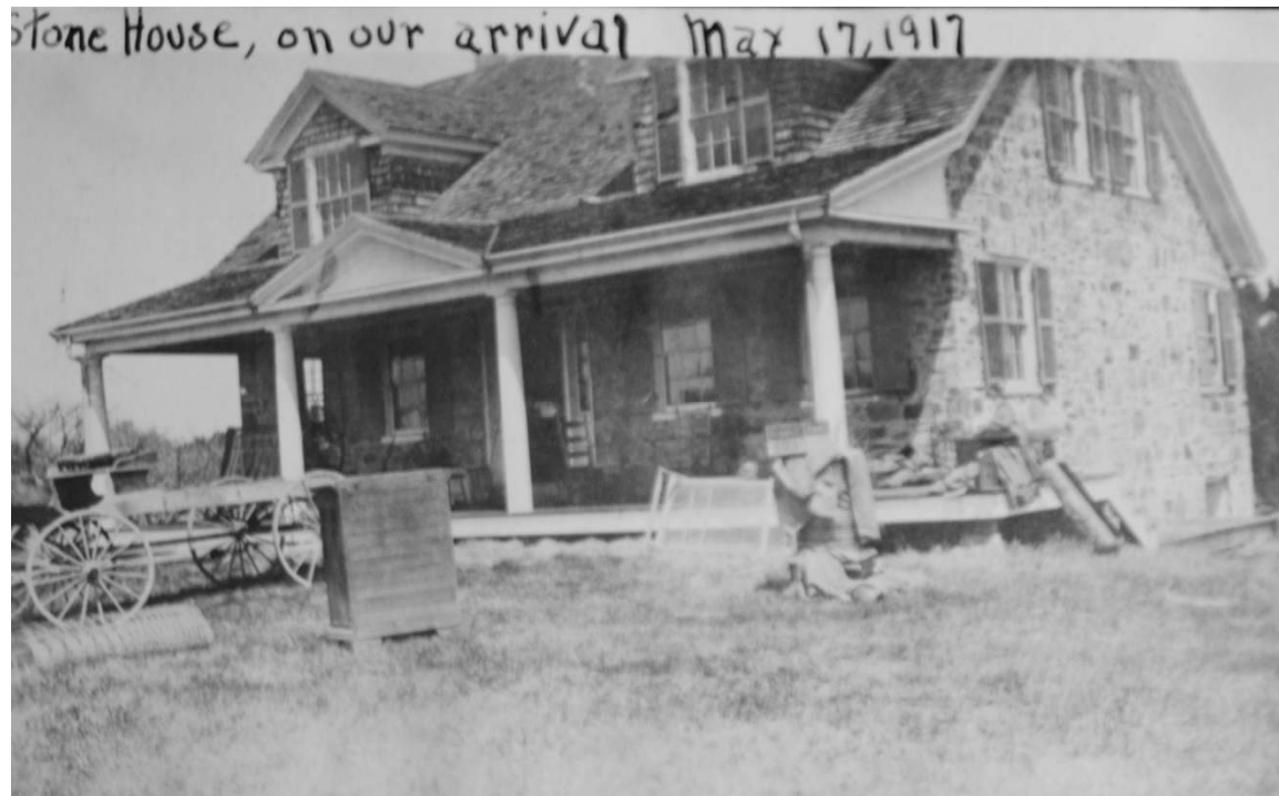
May 1917, facing north
