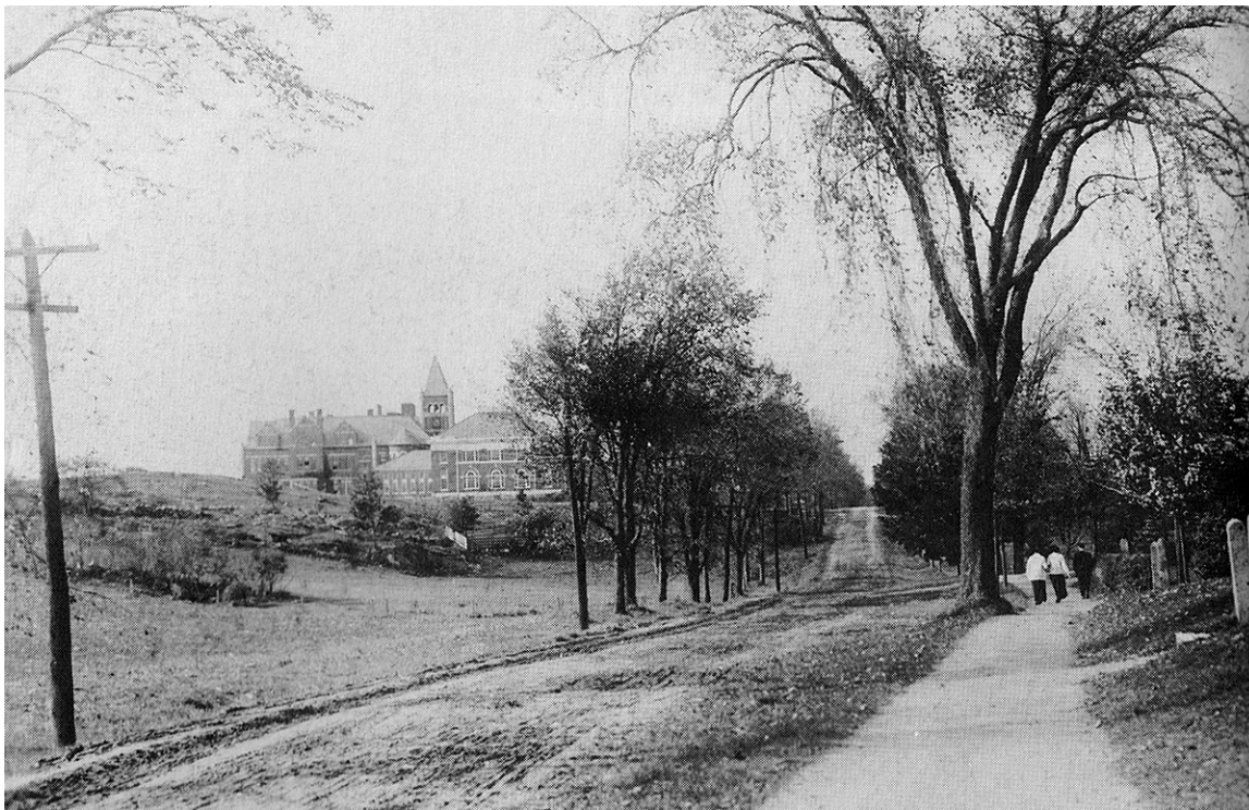
Main Street facing west toward campus, Hamilton Smith and Thompson halls, ca. 1910 (Ross and House 1996, 100)
