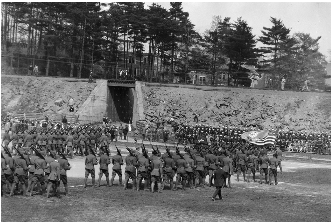
Library Way Railroad Bridge from Brackett Field, ca. 1926 (University of New Hampshire Library Digital Collections)
