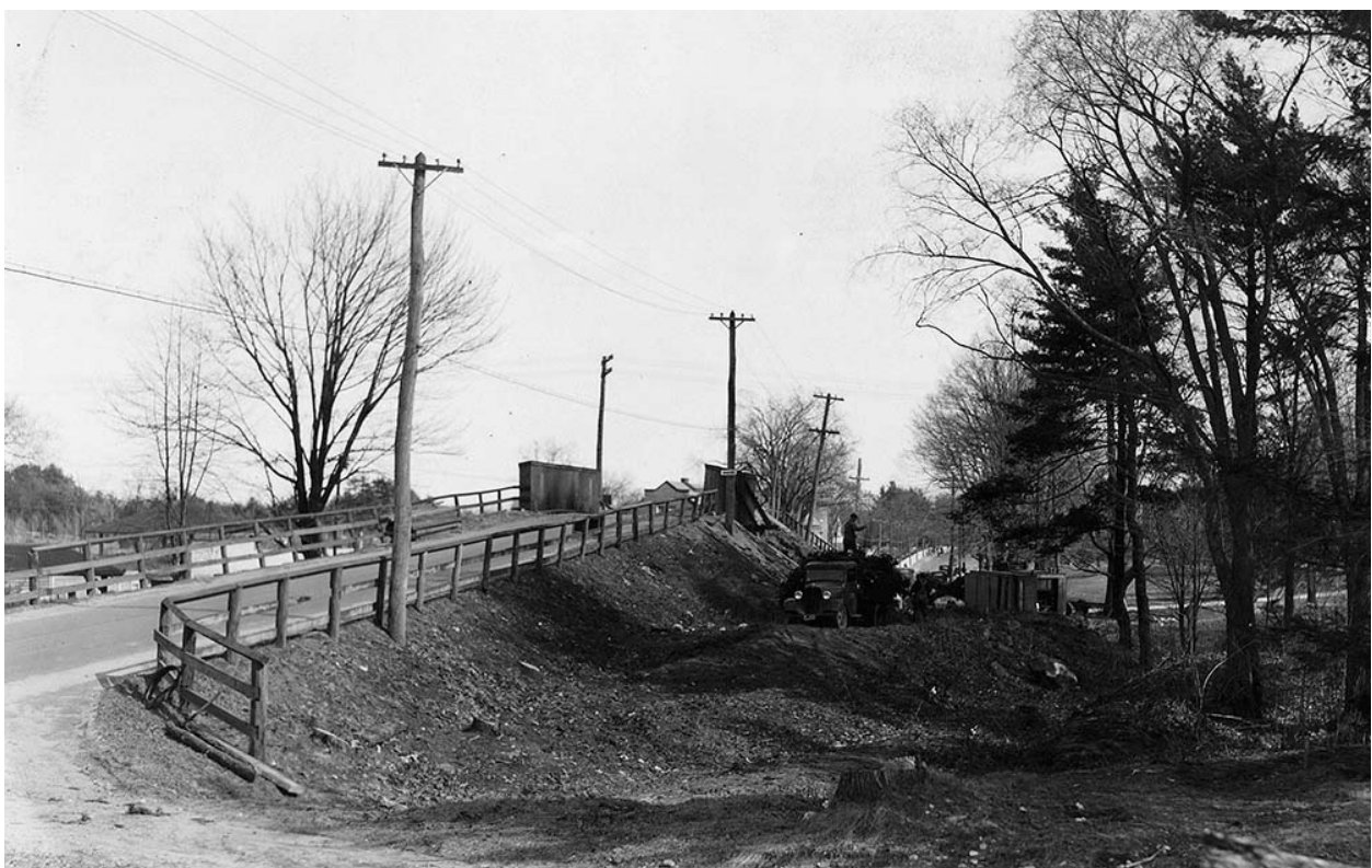
Main Street railroad overpass built ca. 1911-12 before replacement, ca. 1935 view (University of New Hampshire Library Digital Collections)
