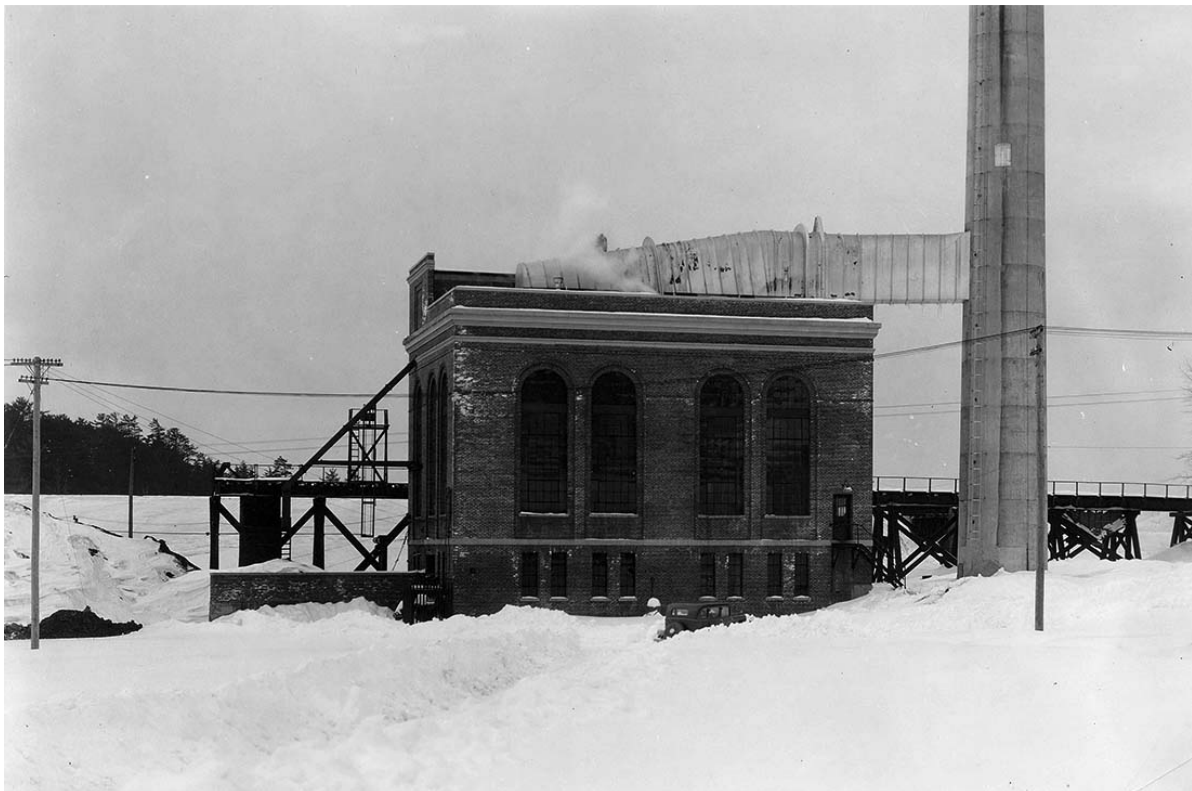
Heating Plant, Library Way, ca. 1935 (University of New Hampshire Library Digital Collections)
