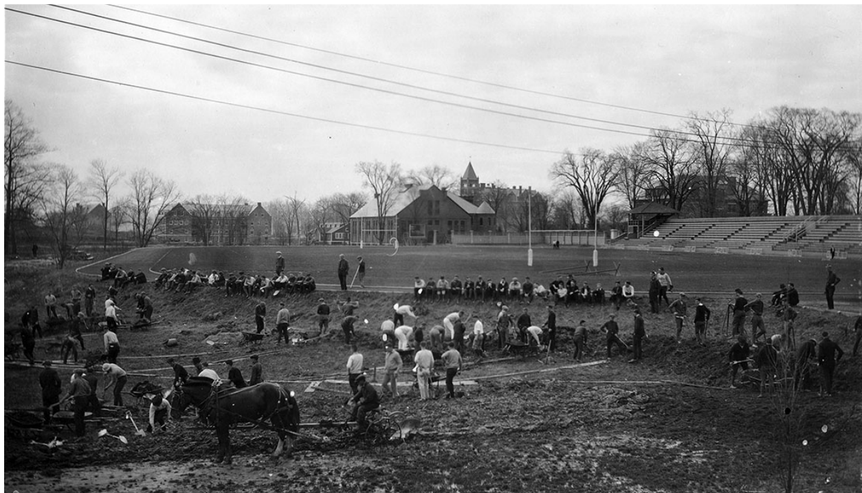
Memorial Field, 1923, looking toward center of campus (University of New Hampshire Library Digital Collections)
