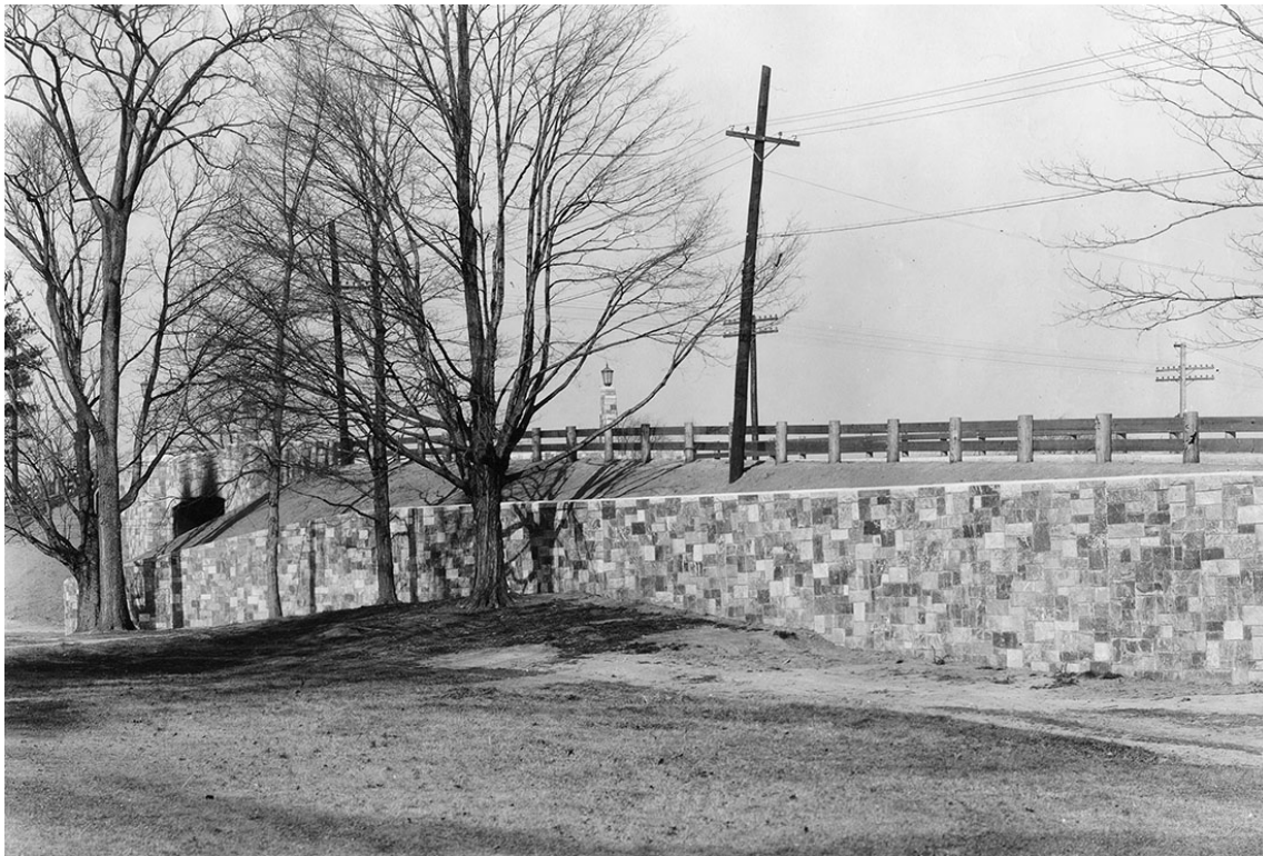
Main Street Bridge over Boston & Maine Railroad, completed 1936 (University of New Hampshire Library Digital Collections)
