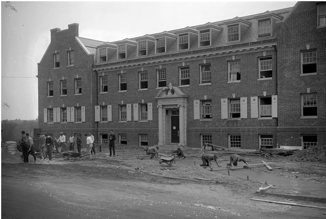
Fairchild Hall, concrete walk construction, 1922 (University of New Hampshire Library Digital Collections)
