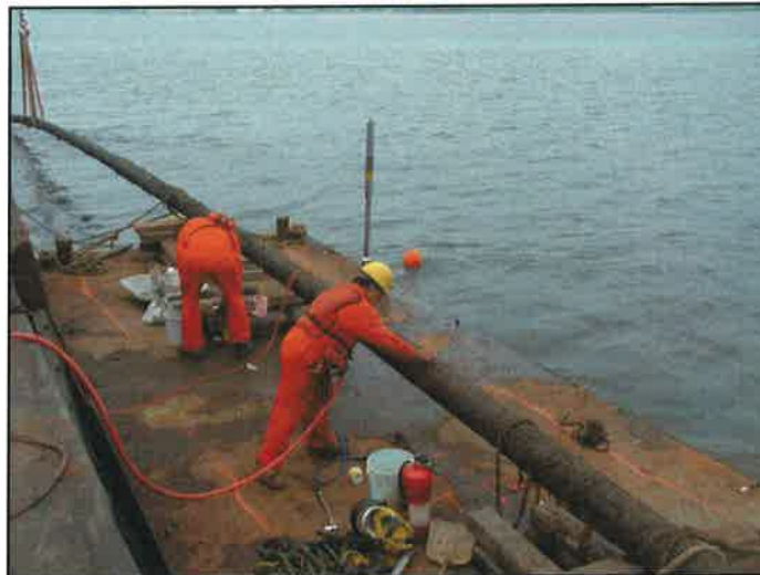
HDD Tie-in of existing 12" Submarine product line
