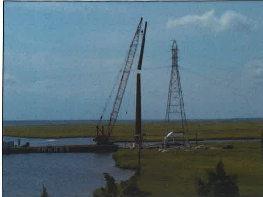
Transmission Tower Installation
