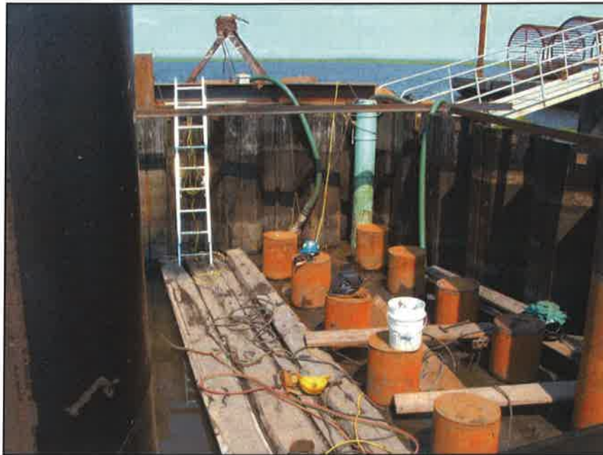
Marine Cofferdam Construction
