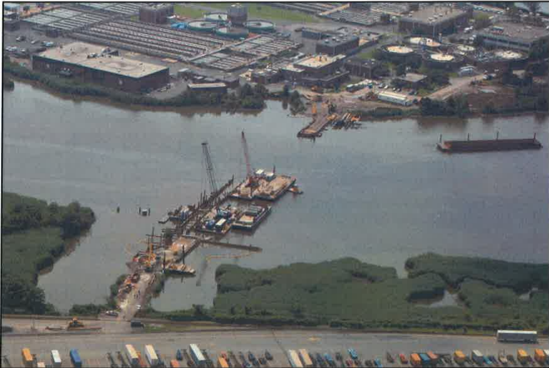
Submarine Pipeline Installation
