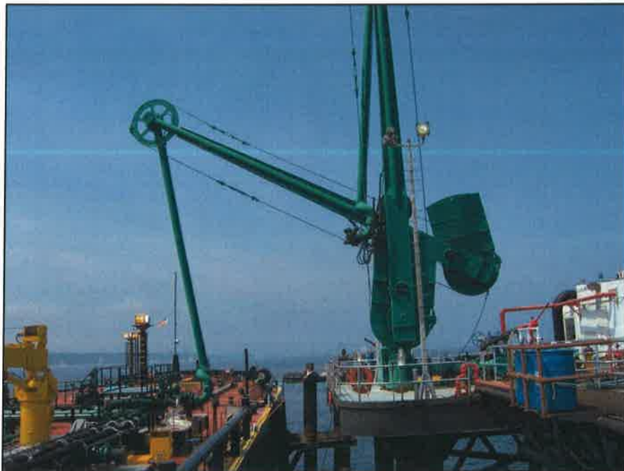
Loading Arm installation at offshore platform
