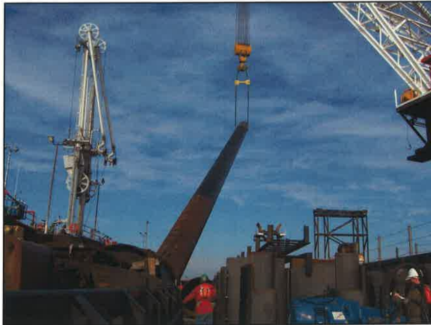
170 Foot Mono-Pile Installation at Offshore Platform
