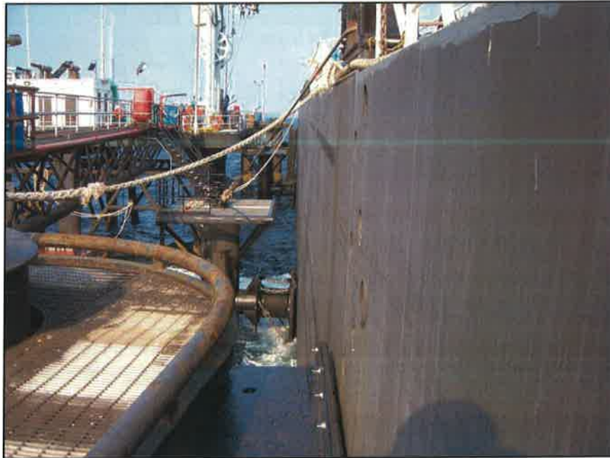
Fender Installation at Offshore Platform
