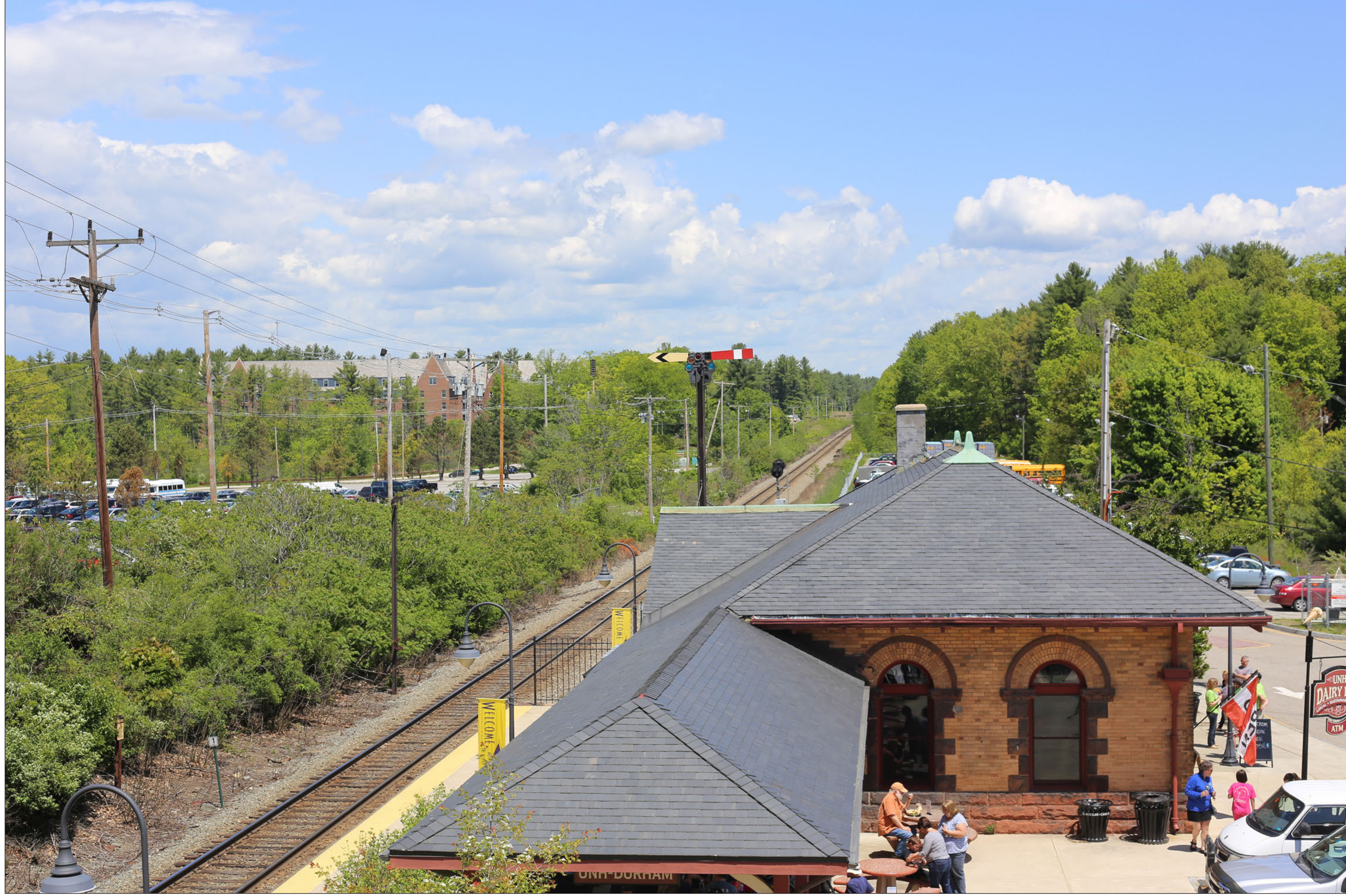
EXHIBIT 8A: EXISTING CONDITIONS FROM DURHAM MAIN STREET/UNH DAIRY BAR, DURHAM, NH (SHEET 2 OF 3)
