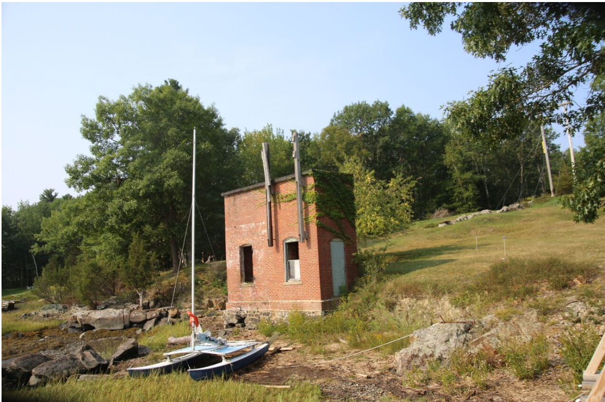
Durham Underwater Cable Terminal House, viewed facing southwest
