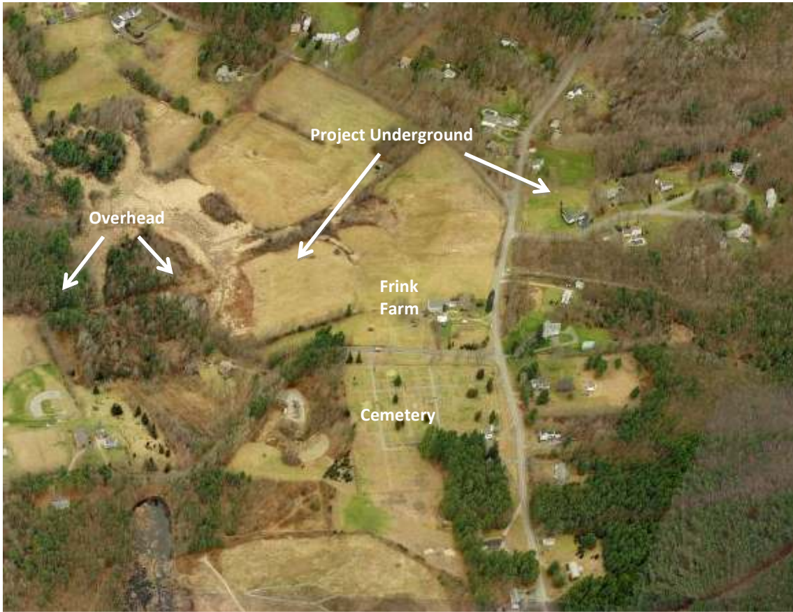
Newington Center Historic District bird's eye view facing north (Bing Maps)
