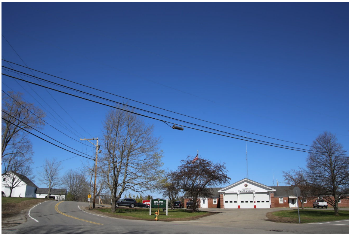
Nimble Hill Road at Fox Point Road, showing setting including twentieth century fire station, facing east
