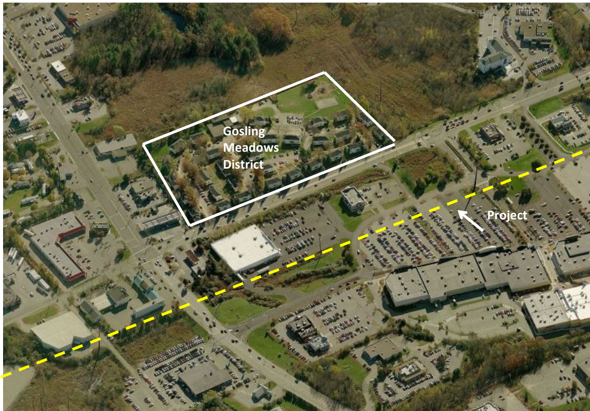
Bird's eye facing south toward Woodbury Avenue/Gosling Road intersection shows extent of late twentieth century development (Bing Maps)
