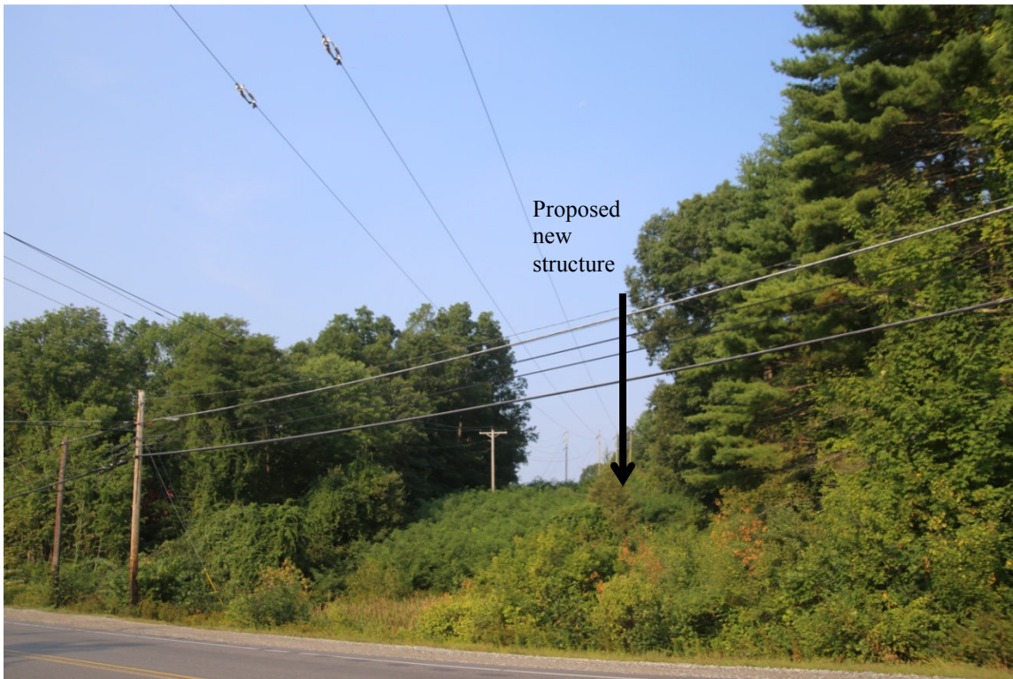
Electric utility corridor west of Newmarket Road, facing west-southwest behind 4 Bennett Road. New H-frame will be visible. Existing H-frames will be removed, single poles will remain.
