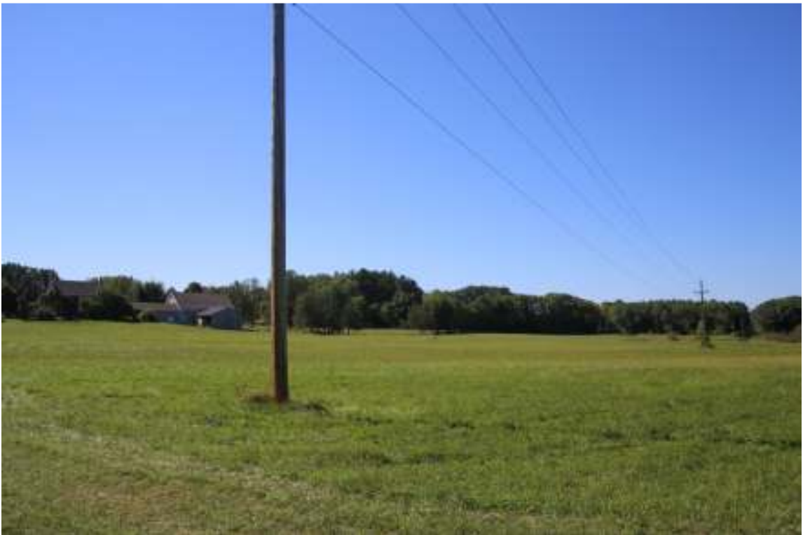
Newington Center Historic District - Frink Farm, facing southwest from Nimble Hill Road . Existing distribution line to be removed and underground transition line installed. Overhead transition at right-hand edge of view.
