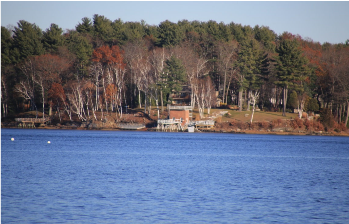
Newington cable house, facing east
