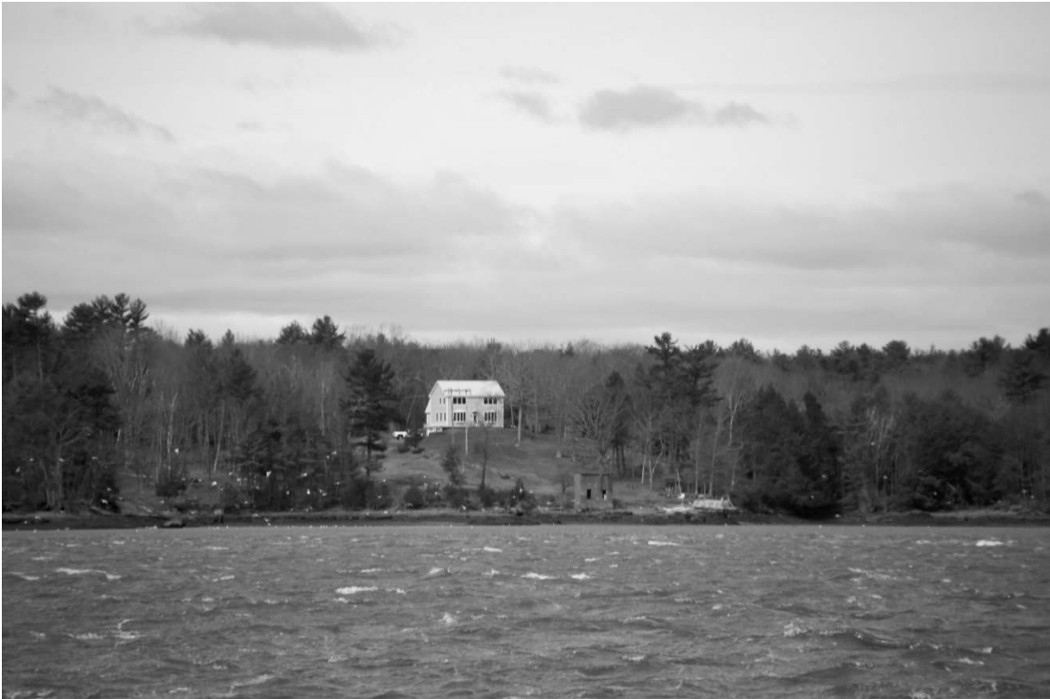
Photo 6) Durham Cable House, from Newington shore of Little Bay
