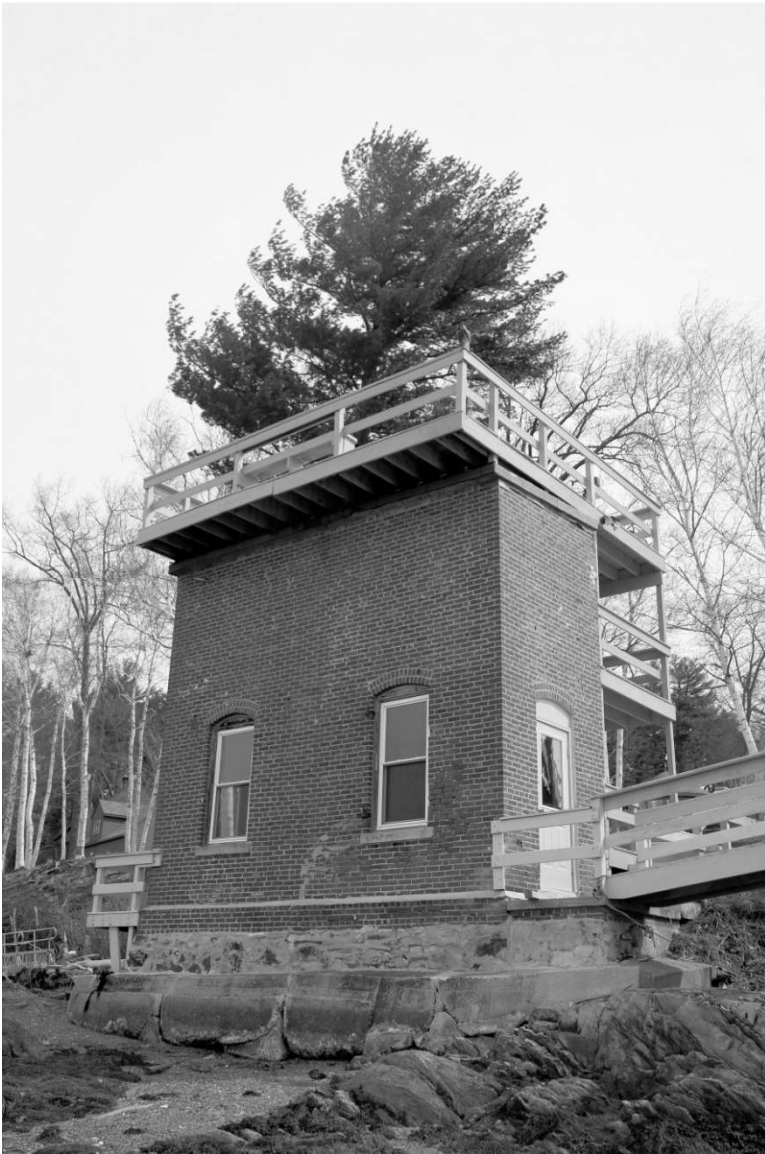
Photo 2) Newington Cable House, from Little Bay shore
