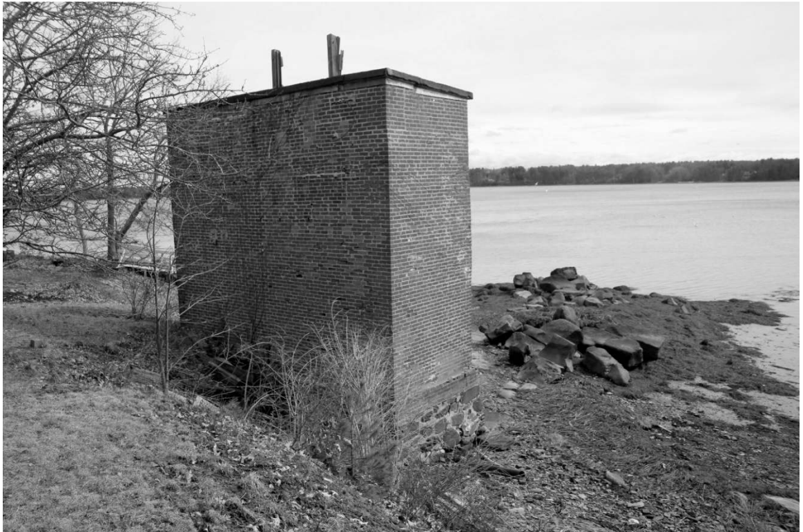
Photo 8) Durham Cable House
