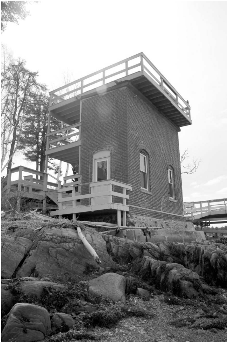
Photo 4) Newington Cable House from the shore of Little Bay
