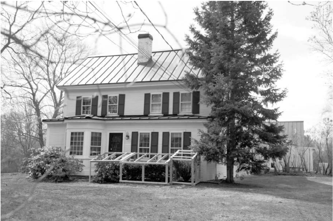
Photo 2: House, east (street) elevation
