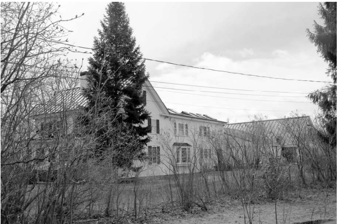
Photo 3: North elevation of house
