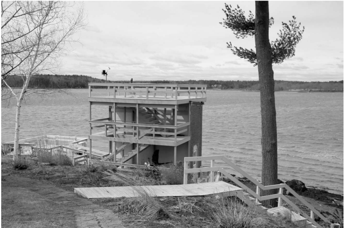
Photo 3) New stairs and deck on cable house from grounds of 44 Gundalow Landing Direction: SW
