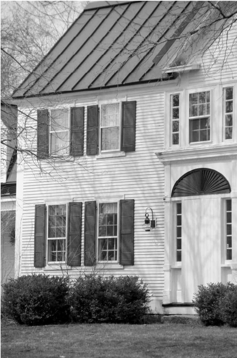
Photo 5: Detail of distinctive frontispiece and 9/9, 6/6, and three-part windows
