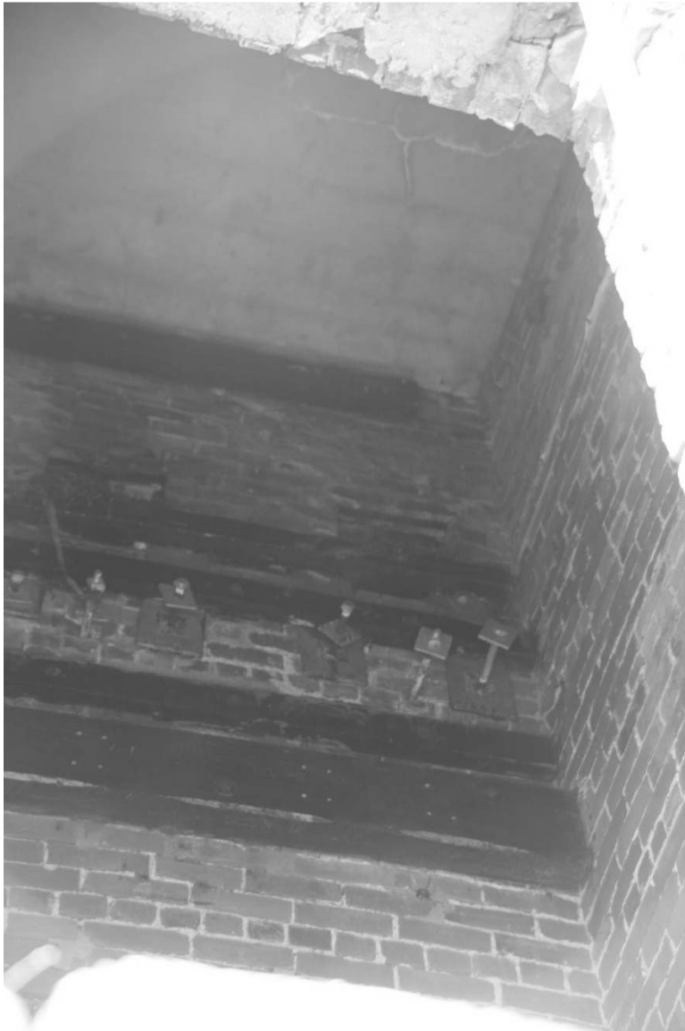
Photo 9) Durham Cable House, interior walls and ceiling
